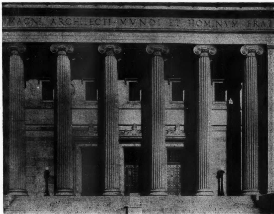
DETAIL OF MAIN ENTRANCE
