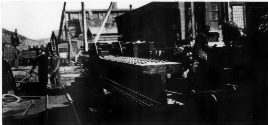
A THIRTY-SIX FOOT COLUMN SECTION WEIGHING NINETEEN TONS IN THE SHOP YARD READY FOR LOADING ON CARS. AN INSPECTOR'S MARK IS SEEN ON THE UPPER PART OF THE COLUMN SECTION
