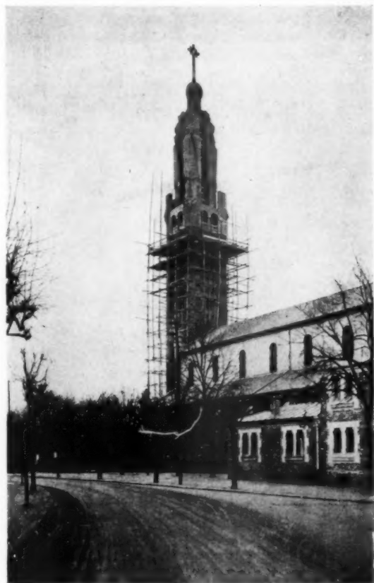
THE CHURCH AT VILLEMOMBLE AND THE TOWER IN COURSE OF CONSTRUCTION
