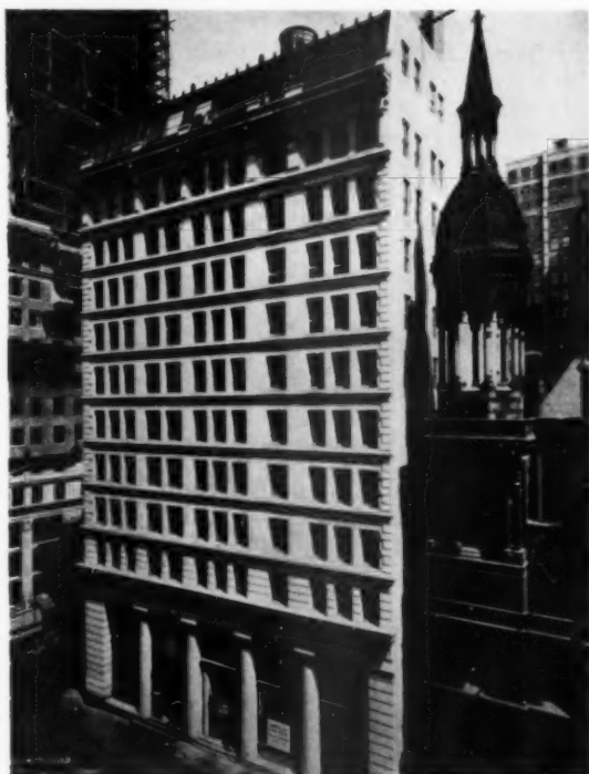
AN ALTERATION TO AN ELEVEN STORY BUILDING TO PROVIDE FOR ADDITIONAL BAYS THAT REQUIRED UNUSUAL ENGINEERING FEATURES. STRUCTURAL WORK OF THIS ORDER REQUIRES THE MOST EXACTING INSPECTION FROM MILL TO BUILDING TO SECURE ACCURACY AND SAFE CONNECTIONS. ORIGINAL BUILDING CONSISTED OF THE THREE BAYS AT THE LEFT. THE ADDITION HAS PROVIDED THE TWO BAYS SEEN AT THE RIGHT
