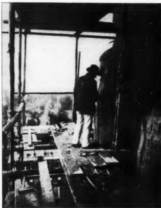
PART OF UPPER SCAFFOLDING
