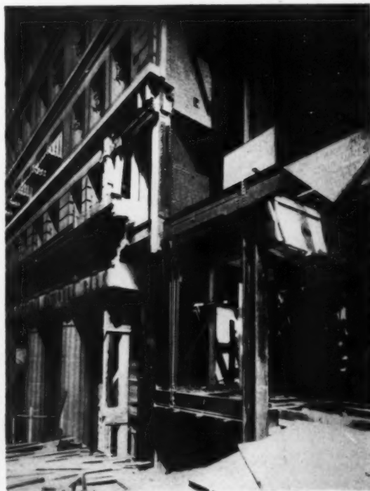
AN ALTERATION TO AN ELEVEN STORY BUILDING TO PROVIDE FOR ADDITIONAL BAYS THAT REQUIRED UNUSUAL ENGINEERING FEATURES. STRUCTURAL WORK OF THIS ORDER REQUIRES THE MOST EXACTING INSPECTION FROM MILL TO BUILDING TO SECURE ACCURACY AND SAFE CONNECTIONS. ORIGINAL BUILDING CONSISTED OF THE THREE BAYS AT THE LEFT. THE ADDITION HAS PROVIDED THE TWO BAYS SEEN AT THE RIGHT
