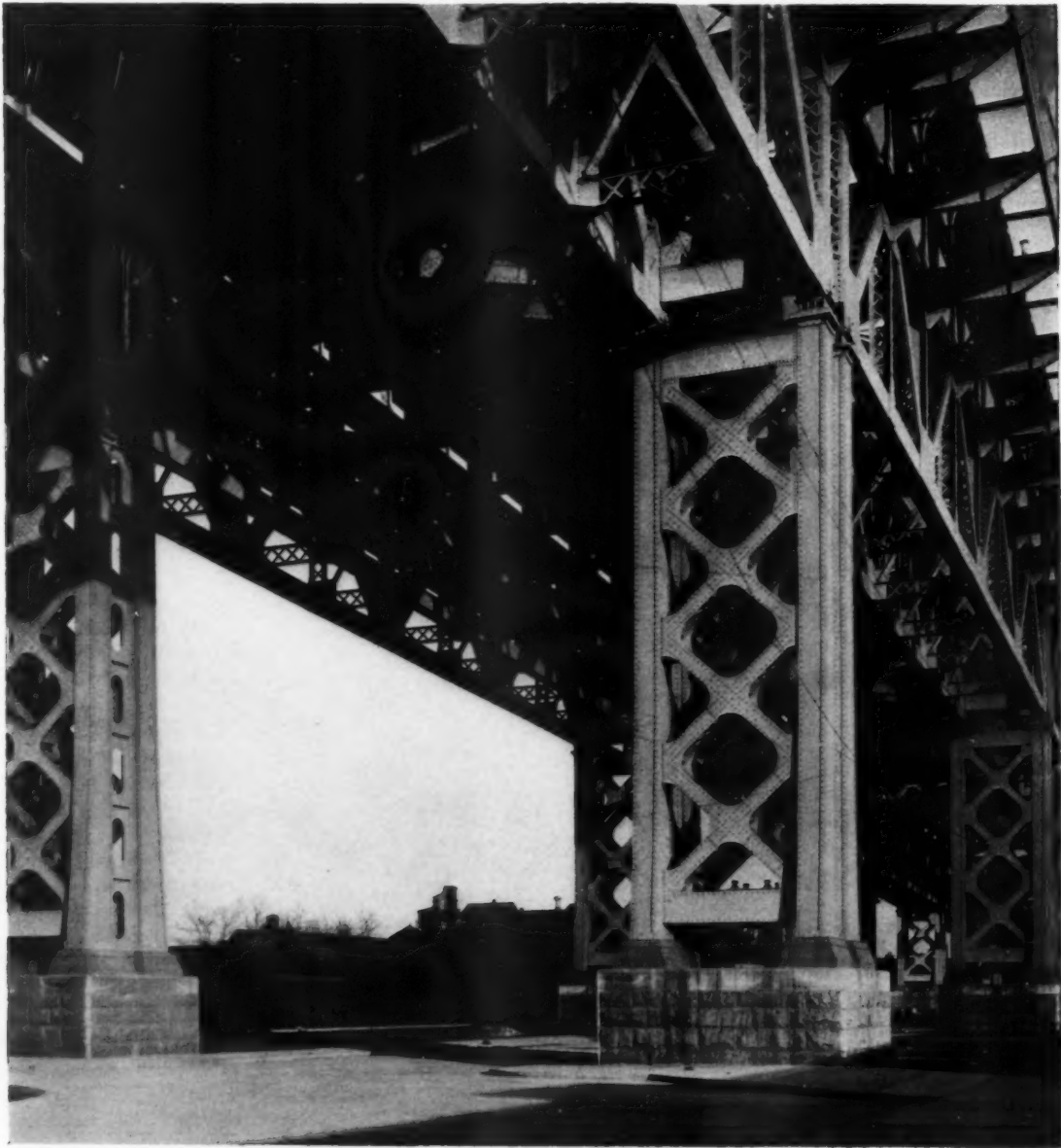
OVER LAND, STEEL TOWERS AND STURDY TRUSSES BRING THE ROADWAYS DOWN TO CITY STREETS
