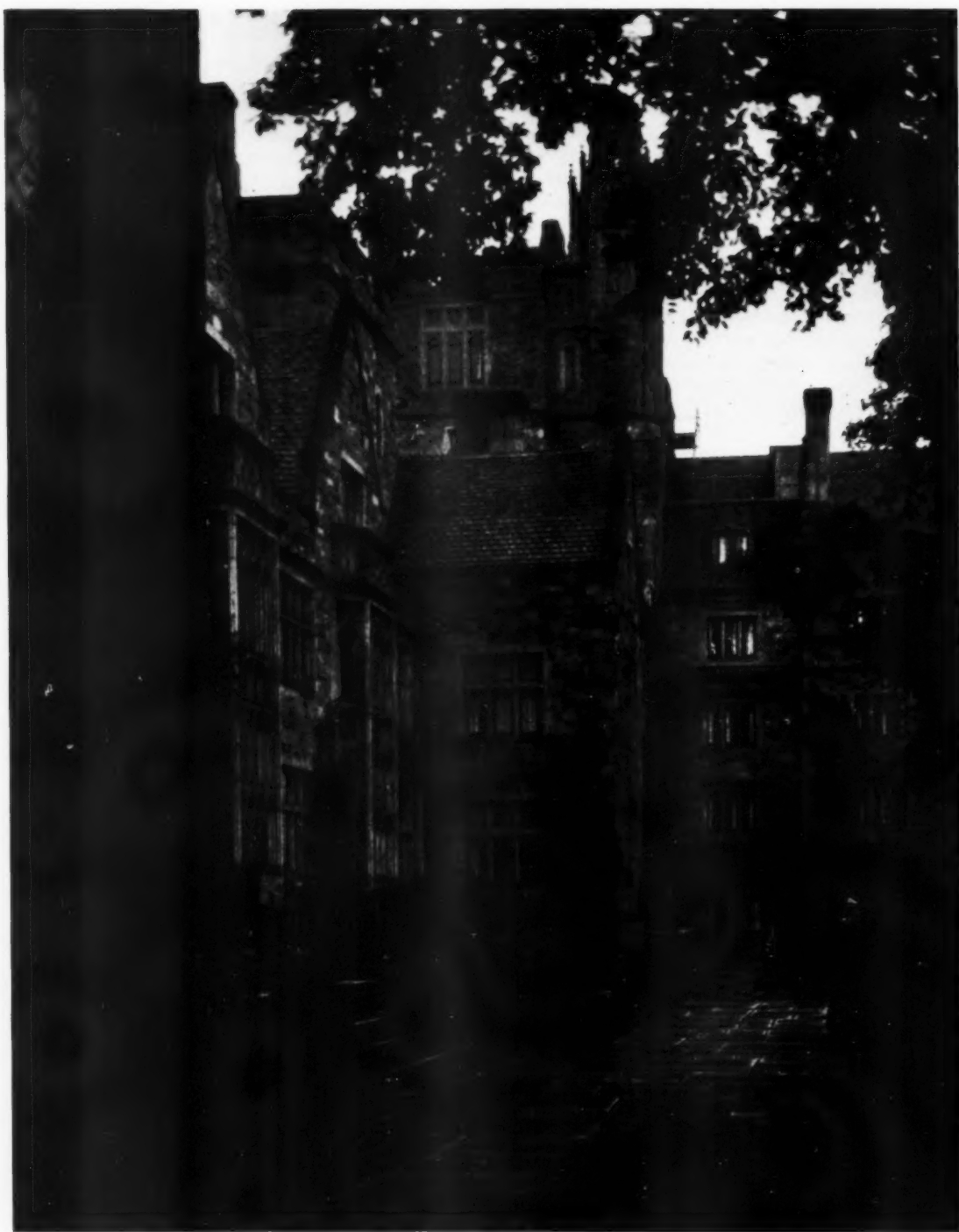
THE HARKNESS QUADRANGLE, YALE UNIVERSITY, ON A RAINY DAY WORKING PHOTOGRAPHS—SERIES II FROM THE ORIGINAL NEGATIVE BY DWIGHT JAMES BAUM, ARCHITECT
