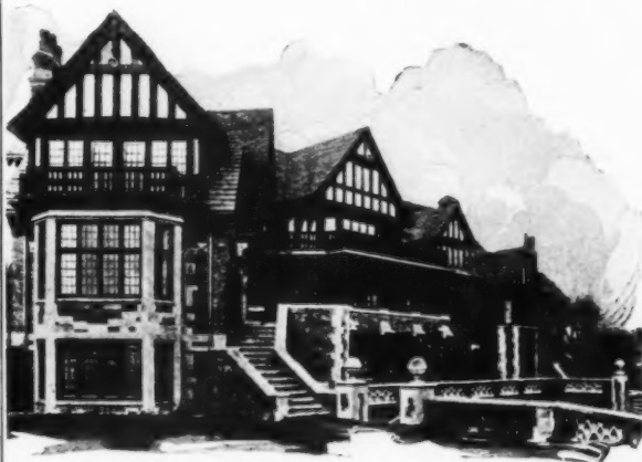
Residence of Ralph Rollins Des Moines, Ia. Boyd & Moore, Architects, Des Moines, Ia. Stanley Ball Bearing Butts used throughout.
