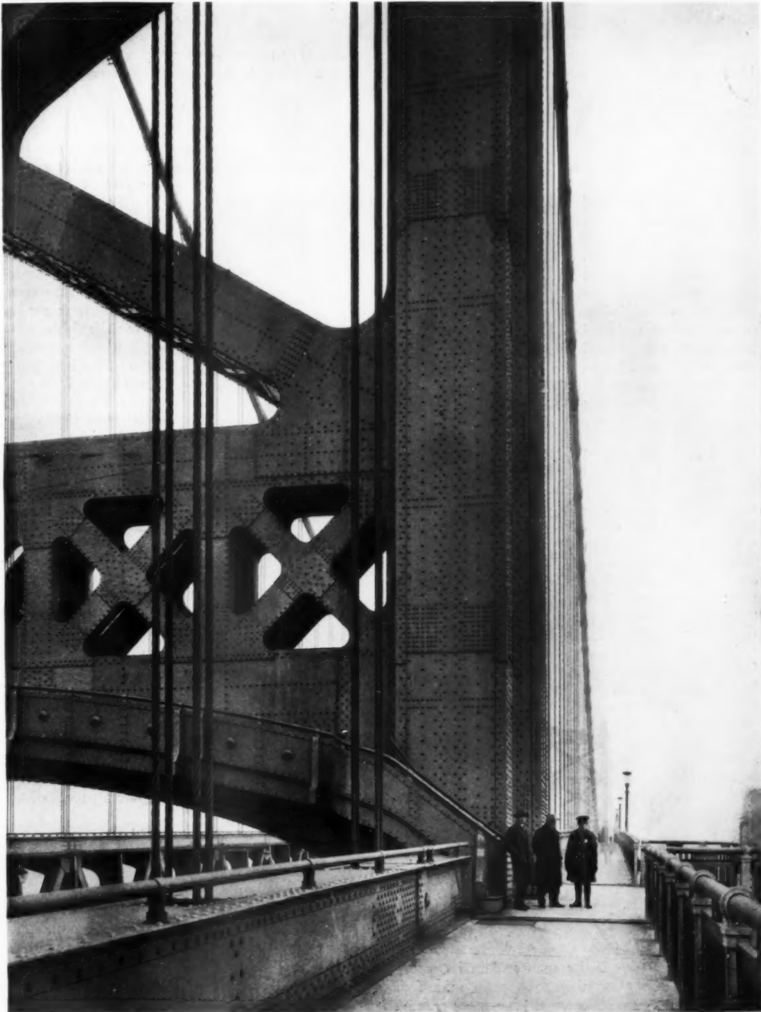
THE FOOTWALKS OUTSIDE THE CABLES AND TRUSSES AFFORD A PROMENADE HIGH ABOVE THE HARBOR. RIVETS WITH COMMONPLACE FUNCTION OF BINDING PLATES AND ANGLES ASSUME PLEASING PATTERNS OF SYMMETRY
