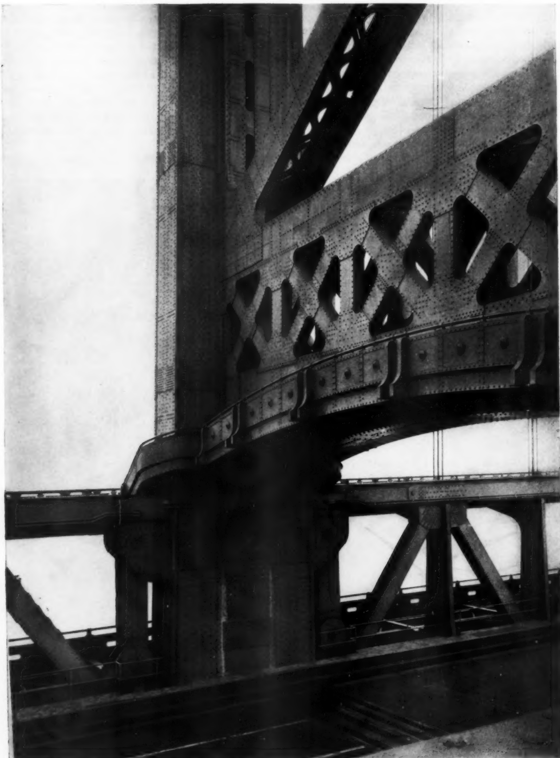
THE ROADWAY PASSES UNDER AN ARCH OF STEEL AT EACH TOWER. ELSEWHERE THERE IS NO CONSTRUCTION OVERHEAD. SIX LINES OF VEHICLES AND FOUR OF RAPID TRANSIT AND TROLLEY CARS CAN MOVE ABREAST
