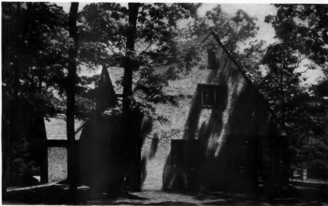
THE DESIGN OF THE EXTERIOR IS FEATURED BY SIMPLE LINES AND GOOD PROPORTION
