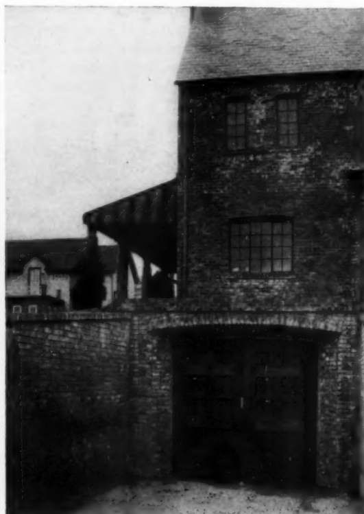
AT LEFT: HOUSE AT GREAT NECK, LONG ISLAND, N. Y., UNDER CONSTRUCTION BEFORE ROOF SLAB WAS PLACED. AT RIGHT: GARAGE ENTRANCE AT CELLAR LEVEL PROVIDING DIRECT ACCESS TO STREET. BRICK RETAINING WALLS MAINTAIN IN MATERIAL, COLOR AND TEXTURE UNIFORMITY WITH THE HOUSE PROPER
