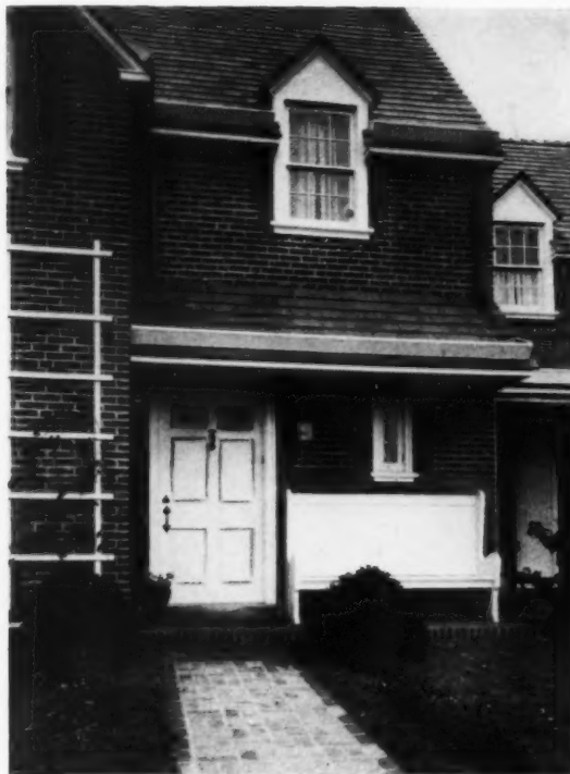
ENTRANCE DETAIL. HOUSE AT DREXEL PARK, PA.
