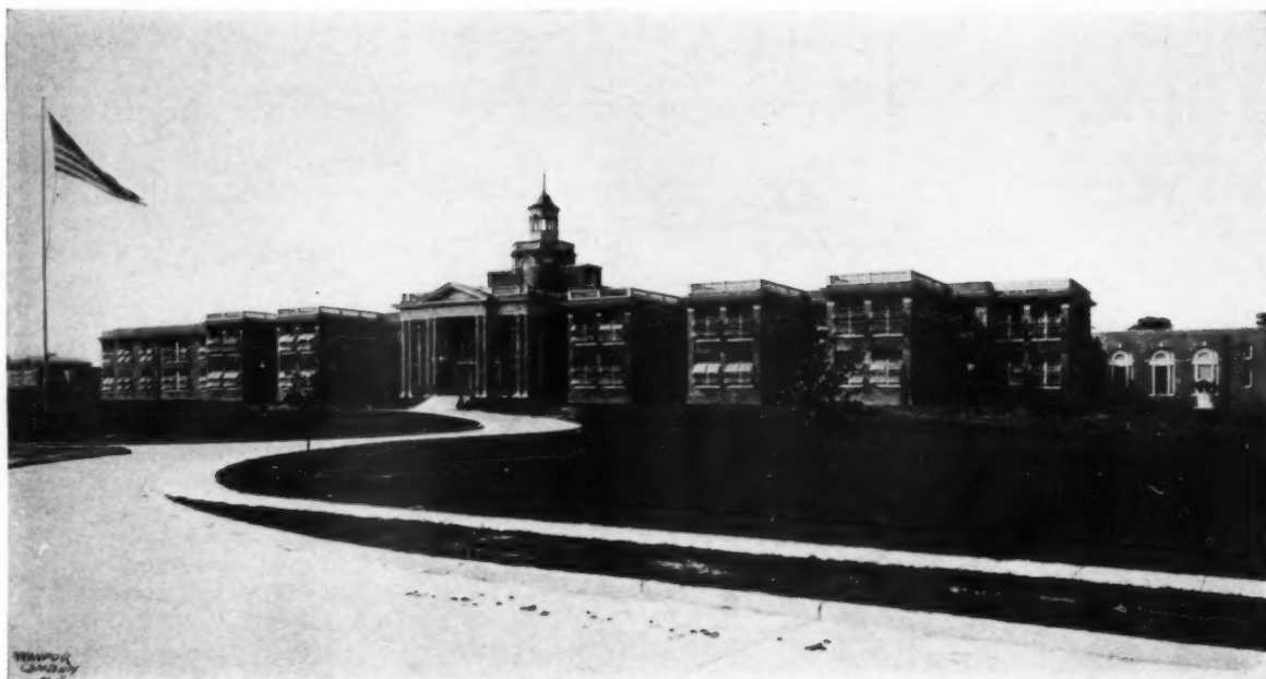
CAMDEN COUNTY TUBERCULOSIS HOSPITAL, LAKELAND, N. J.—ARNOLD H. MOSES, ARCHITECT
