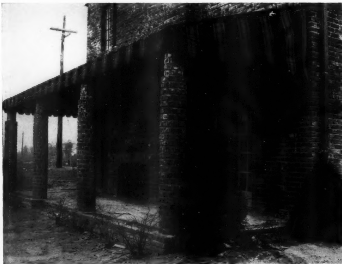
DETAIL OF THE TERRACE. NOTE THE FLOWER BOXES BETWEEN COLUMNS AT THE TERRACE FLOOR LEVEL. THE COLUMNS SUPPORTING THE FRAMEWORK FOR THE AWNING ARE 12" IN DIAMETER FOR A HEIGHT OF 6' 0". THE IMPOSTS ARE 9" IN DIAMETER AND 1' 4" HIGH. THE COLUMNS WERE BUILT UP BY A SERIES OF DRUMS, EACH ONE BRICK COURSE HIGH, MADE IN MOULDS ON THE GROUND, AND SET AS A UNIT OR LAYER OF BRICK AND MORTAR
