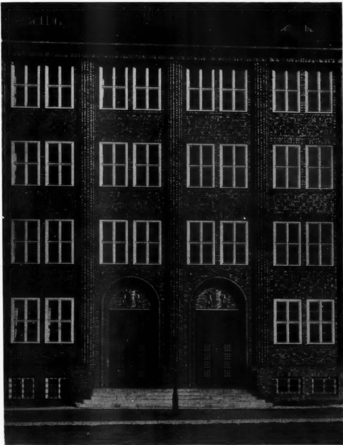
THE SCHOOL FOR THE EDUCATION OF YOUNG MERCHANTS OF HAMBURG, CONSTRUCTED ALMOST COMPLETELY OF BRICKS, HAS MANY NOVEL TREATMENTS. THE VERTICAL FLUTED COLUMNS, THE FLUTES BEING CONVEX INSTEAD OF CONCAVE, CARRY ON THE SPIRIT OF UPWARDS, EVER UPWARDS!—FROM WHICH ONE CAN NEVER BE ABSENT IN MODERN WORK OF THIS SECTION
