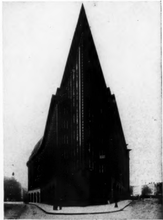
THE CHILI BUILDING SEEN FROM ITS PROW, AS IT MIGHT APPROPRIATELY BE DESCRIBED, CERTAINLY GIVES THE IMPRESSION OF A FORWARD MOVING SPIRIT. ONE CAN HARDLY IMAGINE SUCH A BUILDING BEING DESIGNED BY A DOWNWARD-LOOKING, BACKWARD-SEARCHING ARCHITECT
