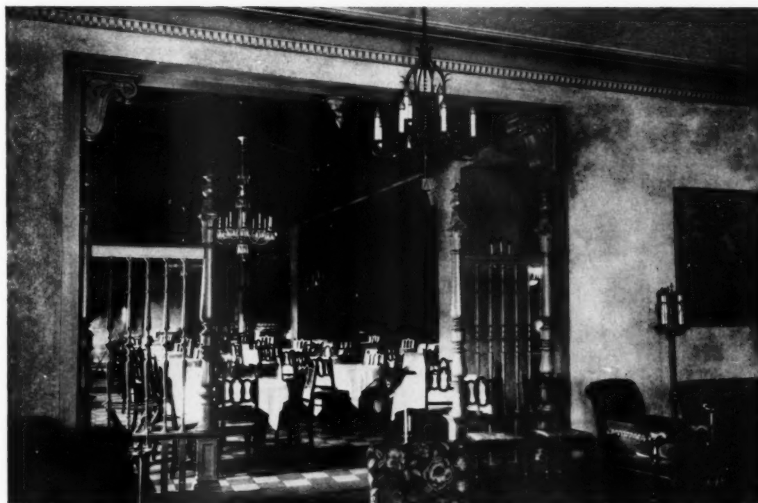
HOTEL ORNDORFF, EL PASO, TEXAS TROST & TROST, ARCHITECTS AND ENGINEERS
