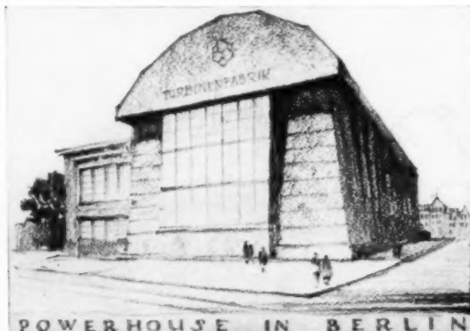
POWERHOUSE IN BERLIN
