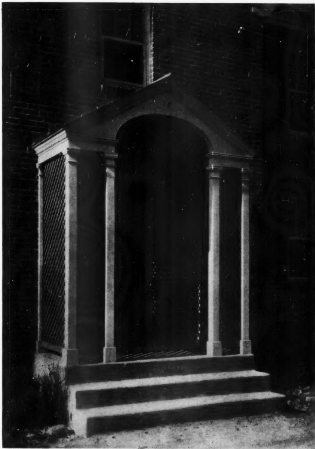
A TYPICAL SHALER LANE DOORWAY
