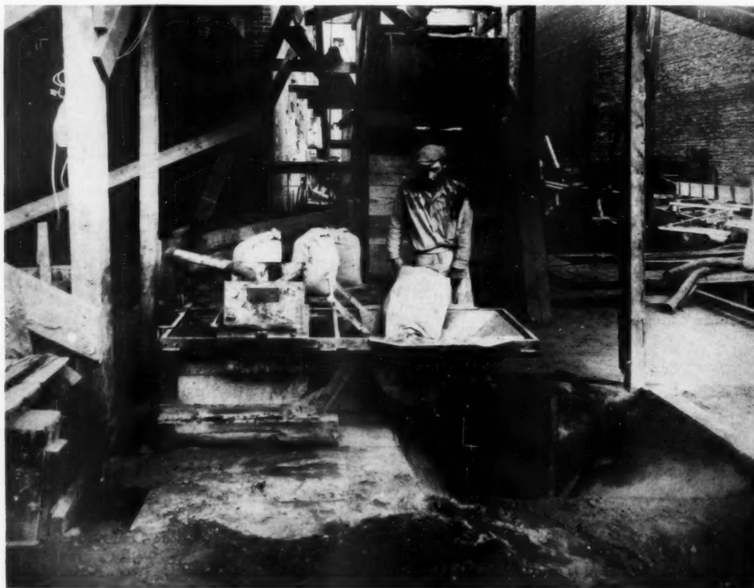
"STRENGTH REGULATOR" IN USE ON A CONCRETE CONSTRUCTION JOB. THE WATER RATIO BALANCING ARM IS SEEN IN FRONT OF THE WATER TANK AND TO THE LEFT OF THE CEMENT HOPPER. THE COMPENSATING MOISTURE ARM IS ON THE OPPOSITE SIDE OF THE MACHINE
