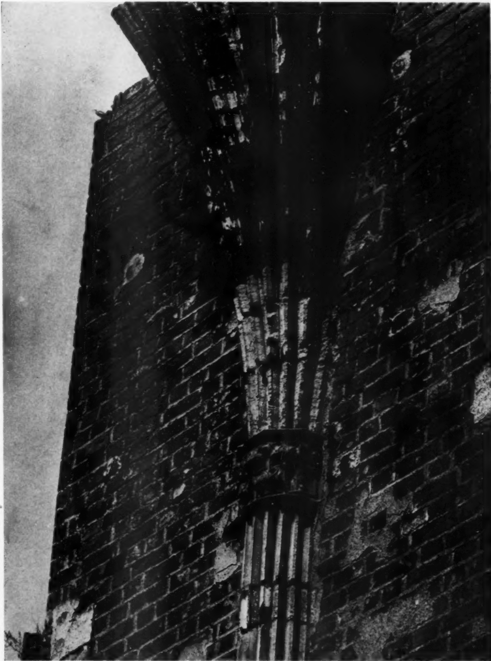
FIGURE 2. VAULTING SPRING IN THE REFECTORY OF ORDENSSCHLOSS REHDEN, NEAR GAUDENZ. THE BUILDING IS ONE OF THE BEWITCHING MONUMENTS OF THE XIII CENTURY
