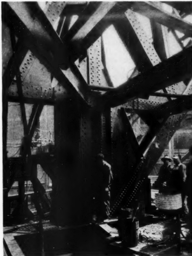
THE LARGE GUSSET PLATE IN TRUSS D1 THAT CONNECTS ITS UPPER AND LOWER PORTIONS
