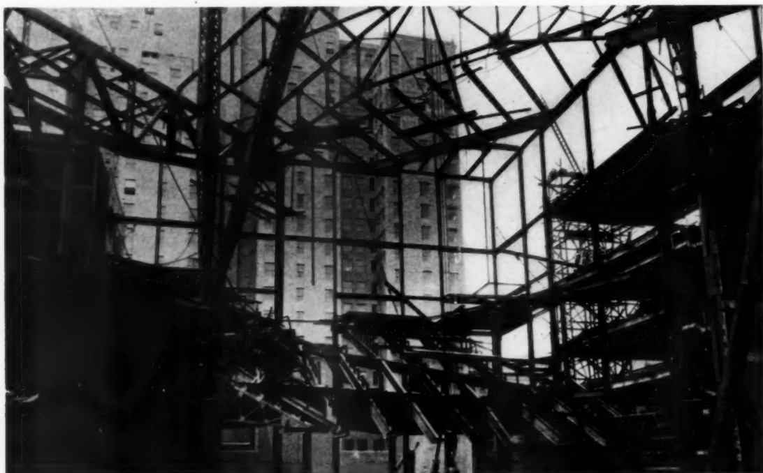
THE BALCONY CANTILEVERED BEAMS PASS THROUGH THE WEB OF GIRDER D4. STEEL ROOF FRAMING IS SEEN IN COURSE OF ERECTION ABOVE THE BALCONY
