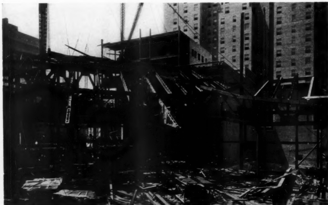
GENERAL VIEW OF BALCONY FRAMING. TRUSS D1 IN UPPER BACKGROUND, WITH TRUSS D3 BELOW AND IN FRONT. CANTILEVER TRUSSES D5 PASS THROUGH TRUSS D3. TRUSS D2 AT RIGHT. GIRDER D4 IN PLACE AT LEFT
