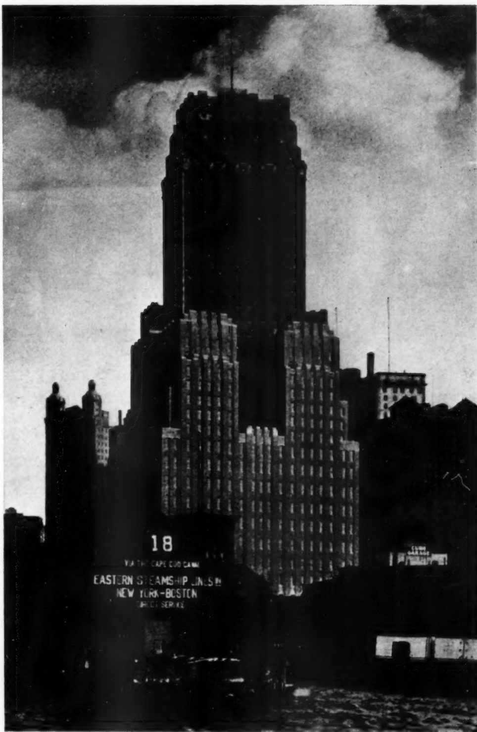
VIEW OF BUILDING FROM THE HUDSON RIVER
