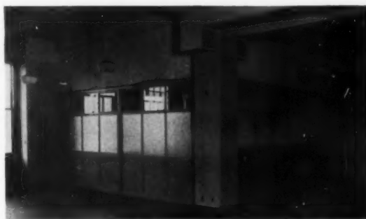
TYPICAL GENERAL CLERICAL SPACE. NOTE VENTILATING SUPPLY OUTLET NEAR CEILING. AIR IS EXHAUSTED THROUGH DUCTS CUT OFF ONE FOOT ABOVE THE FLOOR. ONE OF THESE DUCTS CAN BE SEEN AT THE EXTREME RIGHT
