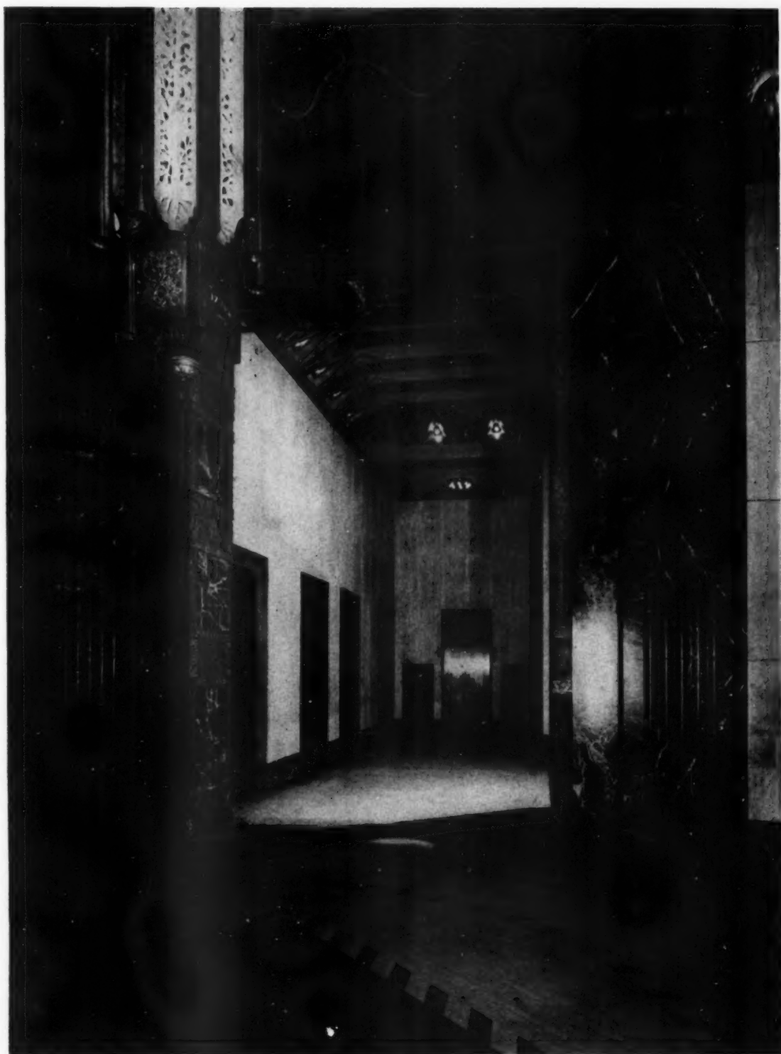
DETAIL IN MAIN CORRIDOR
