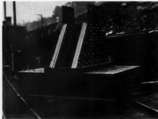
AT LEFT: STEEL FRAMING OF A TYPICAL STORY. AT RIGHT: GRILLAGE AND COLUMN STUB SECTION FOR COLUMN 75. GRILLAGE CONSISTS OF NINE 24" I'S 115# 8'-6" LONG. SLABS 40" X 4" X 6'-10". COLUMN STUB SECTION MADE UP OF FOUR ANGLES 8" X 8" X 1". TWO WEB PLATES 17" X 1". TEN 15/16" COVER PLATES AND TWO 3/8" COVER PLATES. TOTAL WEIGHT 11 TONS
