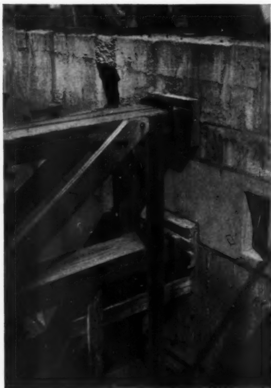
AT LEFT: WEDGING OF TEMPORARY CROSS-LOT TIMBER IN PLACE AGAINST THE FOUNDATION WALL. AT RIGHT: STEEL WEDGES IN PLACE BETWEEN THE MEMBERS OF PERMANENT STEEL CROSS-LOT BRACING AT BASEMENT C LEVEL
