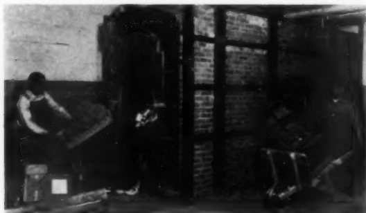
INCINERATOR FOR BURNING WASTE MATERIAL
