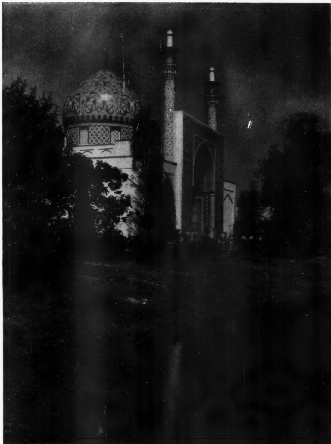
THE PERSIA BUILDING—CARL A. ZIEGLER, ARCHITECT SESQUI-CENTENNIAL INTERNATIONAL EXPOSITION, PHILADELPHIA, PA.
