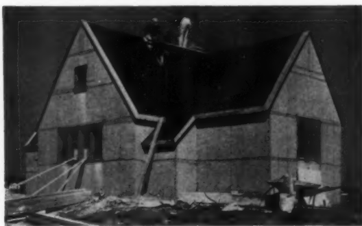
UNIT CONSTRUCTION IS AN AID TO SPEED IN ERECTION AND REDUCES INTERFERENCE BETWEEN TRADES
