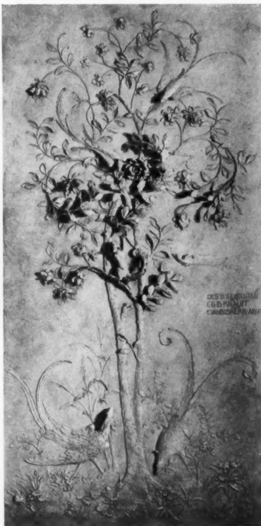
A TEXTURED SURFACE AND ORNAMENT. MODELED BY HAND IN RELIEF, OBTAINED BY A MODERN PLASTIC PRODUCT IN ONE OPERATION
