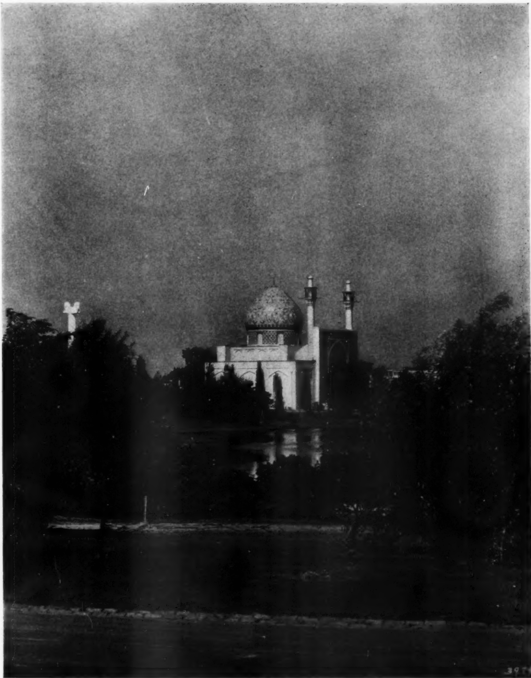
THE PERSIA BUILDING—CARL A. ZIEGLER, ARCHITECT SESQUI-CENTENNIAL INTERNATIONAL EXPOSITION, PHILADELPHIA, PA.
