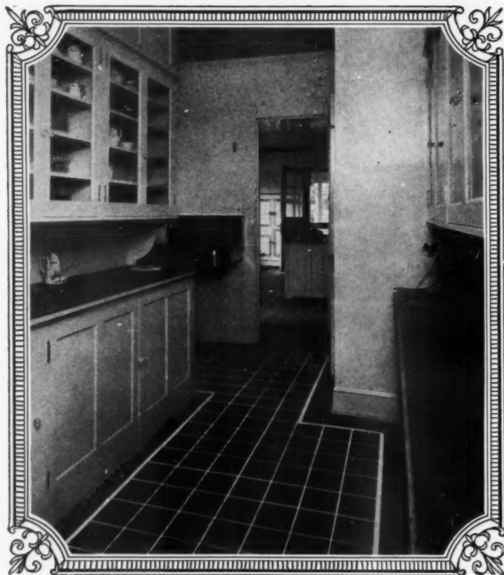
BUTLER'S Pantry and Kitchen in the residence of Mr. J. H. Brewer, Grand Rapids, Michigan. Floored with light blue Linotile, with quarter-inch white border strip. Linotile also used on shelves, with brass edging.
