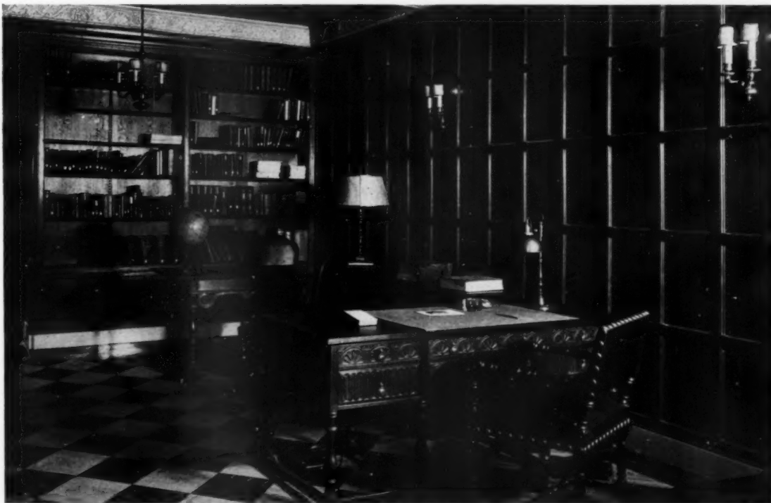
MARBLEIZED RUBBER TILE, LAID HERE IN A TESSELLATED PATTERN, HAS CERTAIN PROPERTIES WHICH OFTEN MAKE ITS USE MORE DESIRABLE THAN THE NATURAL PRODUCT WHICH ITS DESIGN AFFECTS
