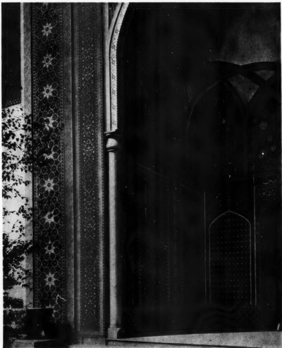
THE PERSIA BUILDING—CARL A. ZIEGLER, ARCHITECT SESQUI-CENTENNIAL INTERNATIONAL EXPOSITION, PHILADELPHIA, PA.
