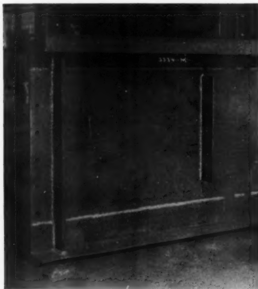
AT LEFT: DETAIL OF END OF 3'-6" x 35' BUILT UP SHOP WELDED GIRDER USED FOR A LARGE CRANE RUNWAY. AT RIGHT: TEST OF A WELDED JOINT MADE BY WELDING A 13" x 10" x \frac{3}{8} " PLATE ON EDGE TO THE WEB OF AN I-BEAM. PLATE BENT AS SHOWN BY SIXTY BLOWS WITH A TWELVE POUND SLEDGE HAMMER. A SIX HUNDRED POUND STEEL RAM HUNG FROM AN OVERHEAD CRANE AND OPERATED BY FOUR MEN DIRECTED FORTY-SIX BLOWS AGAINST THE WELDED PLATE CLOSE TO THE WELD
