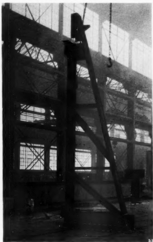
ONE OF SIXTEEN SHOP WELDED A FRAMES FOR A LARGE CRANE RUNWAY
