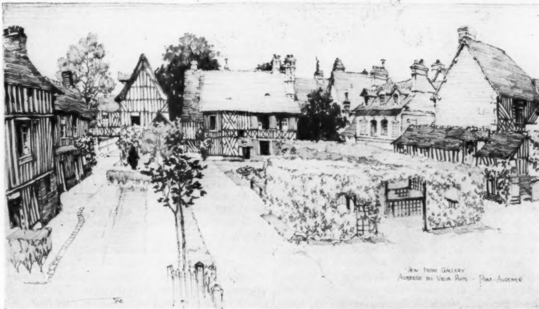
HUGE TANNING VATS FORMERLY OCCUPIED THE CENTER OF THIS ENCLOSURE. IN THEIR PLACE IS THE ARBOR SHOWN IN THIS SKETCH, WHICH SERVES AS INDIVIDUAL DINING ROOMS
