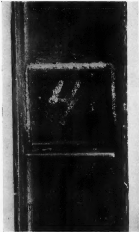
TOP SHELF ANGLE WELDED IN SHOP TO COLUMN. ALL RIVETS WERE REPLACED BY WELDING IN THE PEERLESS AUTO SALES CO. BUILDING AT CANTON, OHIO
