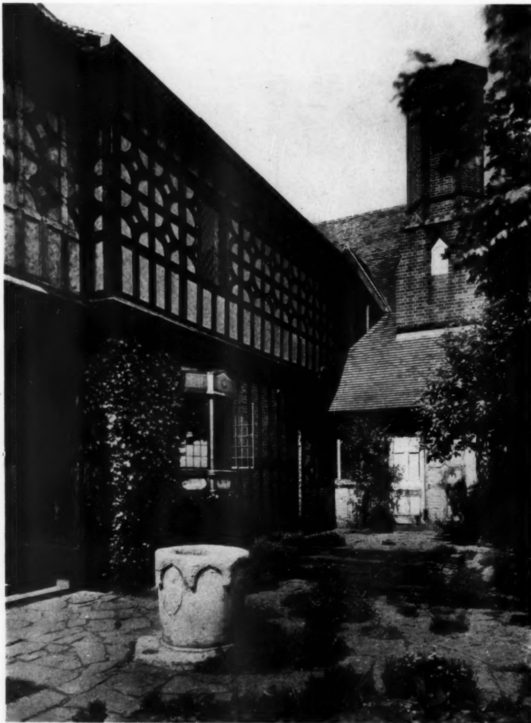
PART OF THE NEW BEDROOM WING BY MR. BENNETT AND MR. HOSSACK, SHOWING THE JUNCTION OF NEW WORK WITH EXISTING
