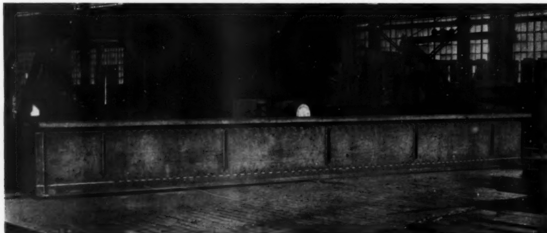
ONE OF FOURTEEN 35 FT. GIRDERS FOR A LARGE CRANE RUNWAY SHOWING SHOP WELDING COMPLETED. GIRDERS BUILT UP OF \frac{1}{2} " x 4'2" WEB PLATE; TWO 6" x 4" x \frac{3}{8} " TOP FLANGE ANGLES COVERED BY A 15" STIFFENER CHANNEL ATTACHED TO TOP FLANGE ANGLES BY INTERMITTENT WELDS ABOUT 2 \frac{1}{2} " LONG, 8" ON CENTERS, TWO 6" x 6" x \frac{3}{8} " BOTTOM FLANGE ANGLES. WEIGHT OF EACH GIRDER 6800 POUNDS
