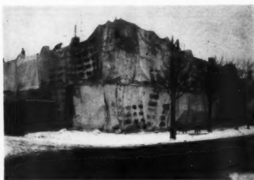
BITTEL KOW HEATING ENGINEERING CO. BUILDING, DETROIT, MICH. PHOTOGRAPH TAKEN JANUARY, 1925. THE JOB WAS ENTIRELY ENCLOSED WITH CANVAS AS A PROTECTION TO MASONRY AND WORKMEN
