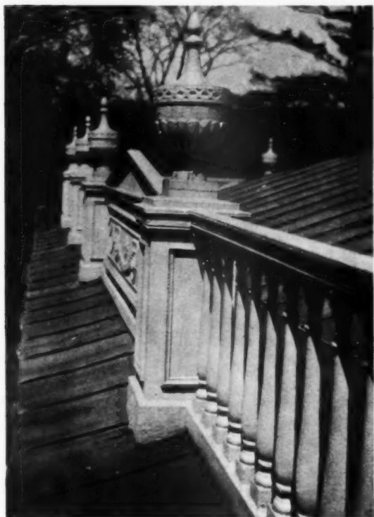
THE ROOF BALUSTRADE
