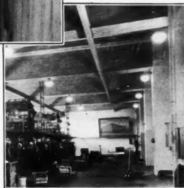
Press room, Milwaukee Journal, Milwaukee, Wisconsin. Frank D. Chase, Inc., architects. Acousti-Celotex used on ceiling to quiet noise.
