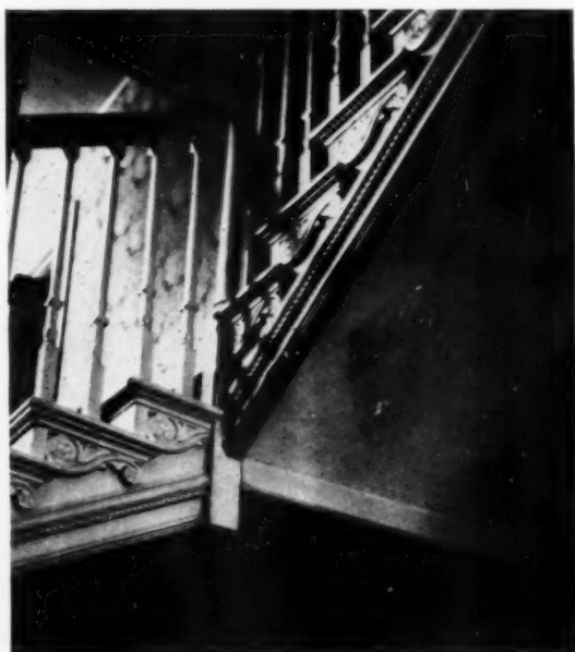
DETAIL OF STAIRWAY
