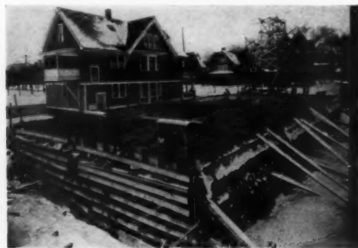
AT LEFT: APARTMENT BUILDING, MILWAUKEE, WIS. ROSSMAN-WIERDSMA, ARCHITECTS. PHOTOGRAPH TAKEN JANUARY 5, 1923. THIS FORM OF PROTECTION MUST BE CAREFULLY DONE, USING SUFFICIENT MATERIAL TO ASSURE POSITIVE PROTECTION TO THE MASONRY AND ACCOUNT TAKEN OF THE EXPECTED TEMPERATURES. AT RIGHT: DETROIT FREE PRESS PAPER BUILDING, DETROIT, MICH. ALBERT KAHN, ARCHITECT. PHOTOGRAPH TAKEN JANUARY 17, 1925. A THIRTEEN STORY REINFORCED CONCRETE STRUCTURE, WORK UPON WHICH WAS CONTINUED THROUGHOUT THE WINTER. NOTE THE PROTECTION ON BUILDING WHERE WORK IS IN PROGRESS
