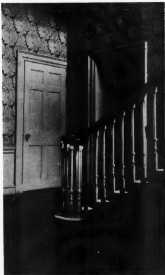
DETAIL OF STAIRWAY
