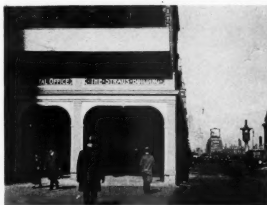
CLOSE-UP OF CONTRACTOR'S BRIDGE. THE STREET ARCADE WAS A MUCH COMMENTED FEATURE DURING CONSTRUCTION
