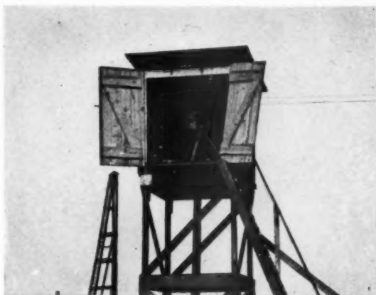
CAMERA SHACK LOCATED ABOUT 25 FEET ABOVE THE GROUND AND 325 FEET FROM THE STRAUS BUILDING
