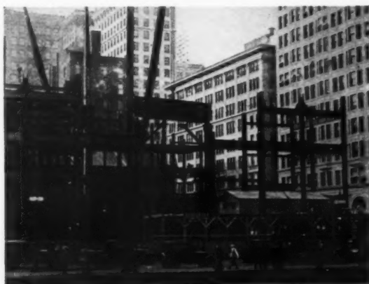
GENERAL "SHOT" SHOWING SETTING OF STEEL GIRDER OVER MAIN ENTRANCE TO THE BANK IN THE STRAUS BUILDING
