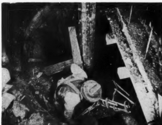
CLOSE-UP OF "SAND HOG" LEAVING A CAISSON USED FOR BUILDING THE FOUNDATIONS OF THE STRAUS BUILDING
