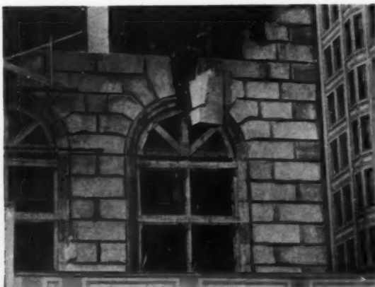
CLOSE-UP SHOWING SETTING OF INDIANA LIMESTONE KEYSTONE OF LOWER WINDOW ON PRINCIPAL FACADE
