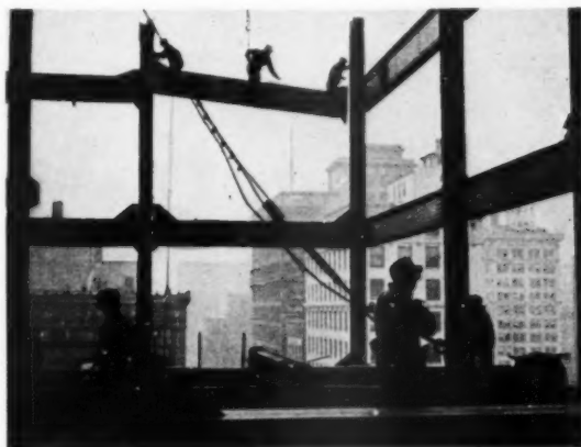
ERECTING THE STEEL FRAME OF THE OFFICE BUILDING. CLOSE-UP OF STEEL WORKERS AT THE EIGHTEENTH FLOOR
