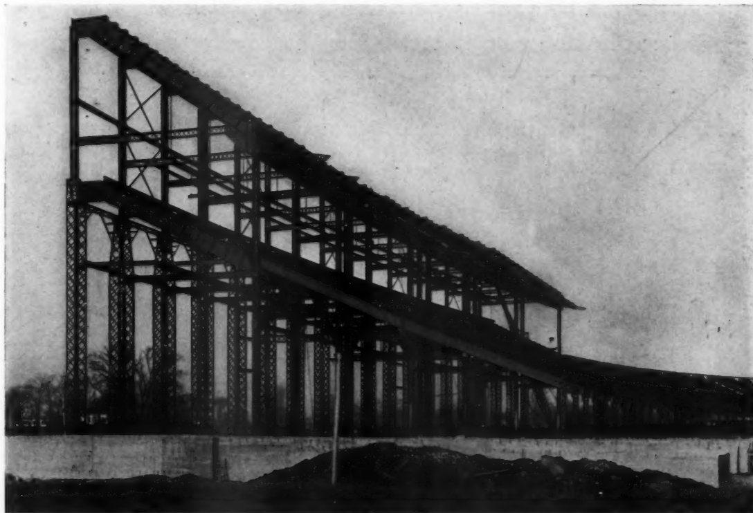
STEEL FRAME OF OHIO STADIUM
