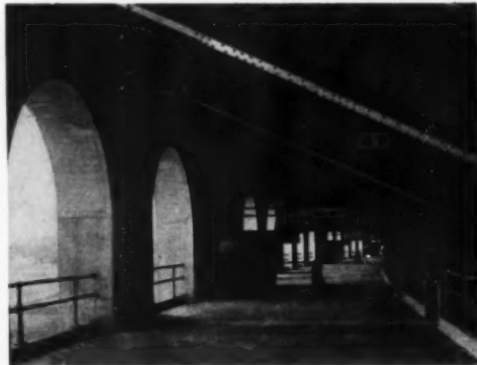
INTERIOR OF OHIO STADIUM DISTRIBUTION GALLERY SHOWING STAIRS AND PORTALS OF "AMBULATORY" ABOUT 40 FEET ABOVE THE GROUND JUST BELOW COVERED PORTION OF LOWER DECK
