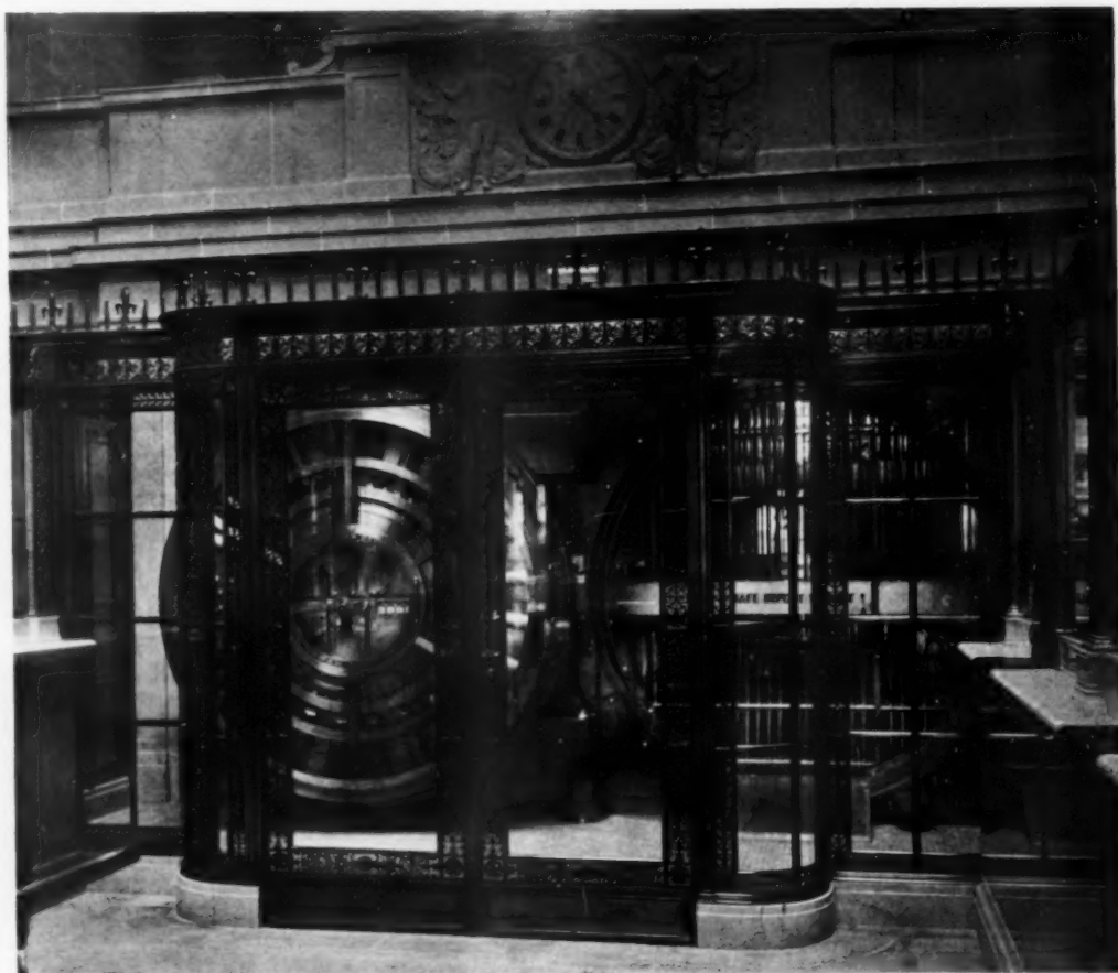
GRILLE IN FRONT OF SAFE DEPOSIT VAULTS, CITY NATIONAL BANK, GALVESTON, TEXAS
