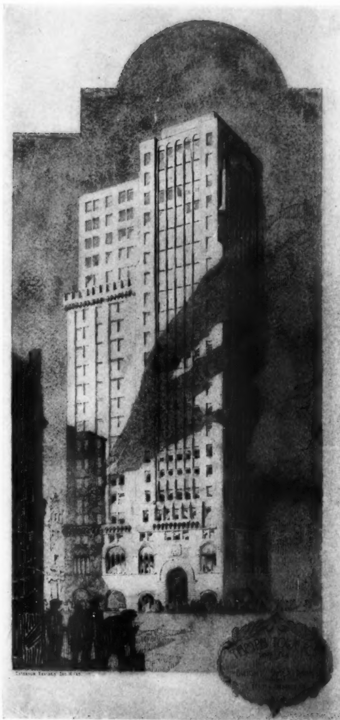
TAMPA TOWERS, TAMPA, FLA.
