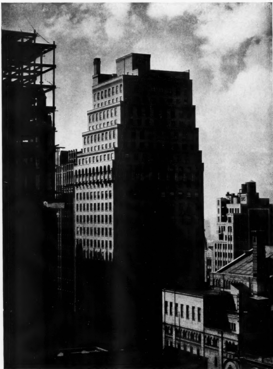
BUILDING NO. 550 SEVENTH AVENUE, NEW YORK
