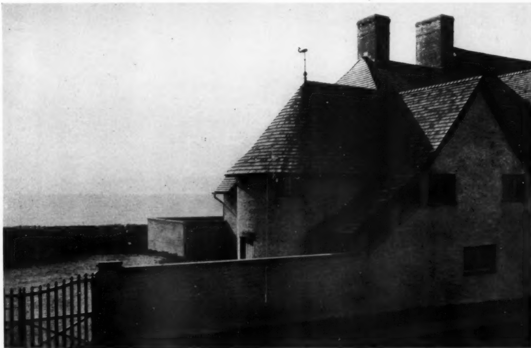
THE ROUND REFRIGERATOR ROOM COMBINED WITH THE STAIRS TO THE SERVICE WING. NOTE THE WHALE WEATHER VANE APPROPRIATE IN ITS ADAPTATION FOR EAST HAMPTON. THEY SAY THAT THE COMPLETION OF THE BUILDING WAS DELAYED SOMEWHAT IN THE PROCESS OF ITS ERECTION BY THE VISIT OF A SCHOOL OF WHALES
