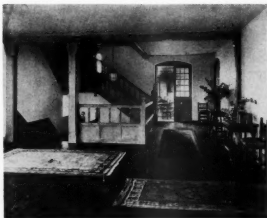
THE MAIN STAIRS WHICH DESCEND TO THE MAIN ENTRANCE AND CONTINUE UP TO THE GALLERY OF THE GREAT HALL. THE LOGGIA ON THE NORTH SIDE OF THE GREAT HALL IS SEEN THROUGH THE ARCHED OPENING. THE SIMPLICITY OF DETAIL GIVES A SUBSTANTIAL QUALITY TO THE INTERIOR WHICH IS SUITABLE TO THE EXPOSED SITE OF THE BUILDING. THROUGHOUT THIS BUILDING THE ARCHITECT HAS DESIGNED AND PLANNED TO FITTINGLY MEET THE "ATMOSPHERE" OF LOCATION THAT HAS TRADITION OF THE EARLIEST SETTLEMENT OF LONG ISLAND AND PARTICULARLY OF THE TIME WHEN EAST HAMPTON WAS ONE OF MANY PICTURESQUE WHALING PORTS ON THE EASTERN END OF THE ISLAND
