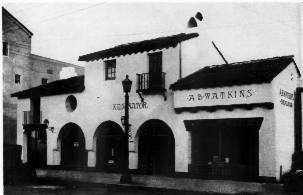
SALISBURY FIELD BUILDING—WM. A. EDWARDS, ARCHITECT; J. J. PLUNKETT, ASSOCIATE
