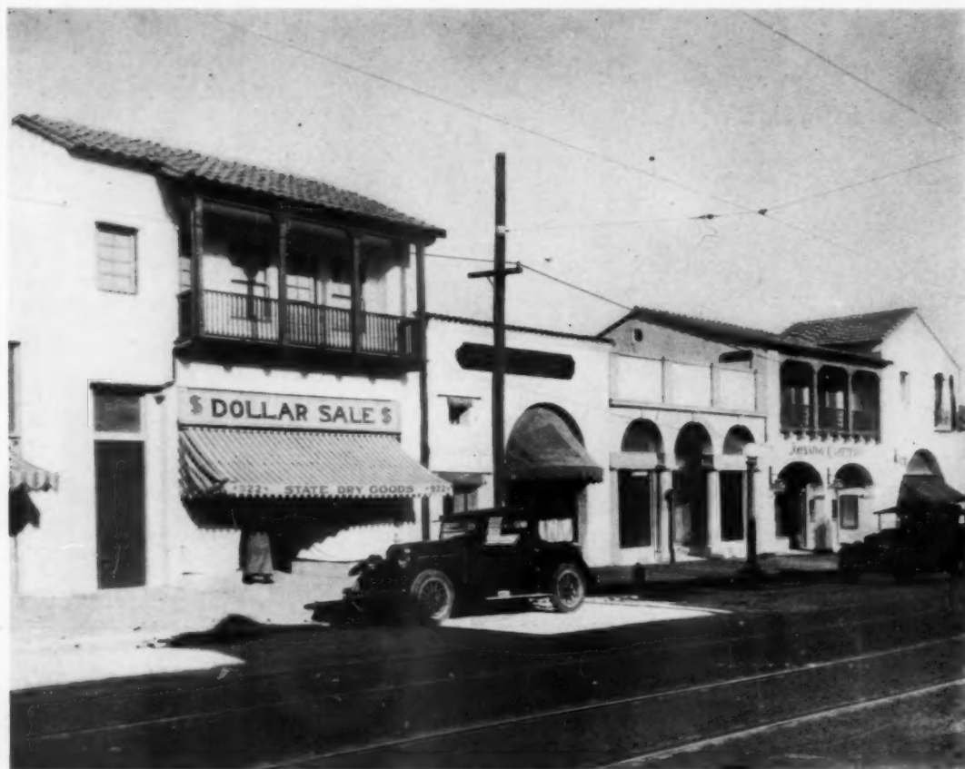
TYPICAL GROUP OF NEW BUILDINGS—THE 900 BLOCK, EAST SIDE (See leading article, "The New Santa Barbara")
