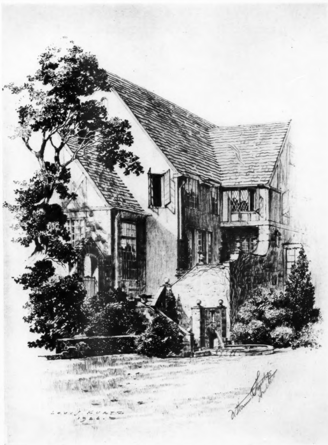
DETAIL OF HOUSE OF JAMES M. McCUTCHEON, SCARSDALE, N. Y.
