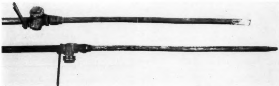
THREE-EIGHTH-INCH PIPE NOZZLES, WITH QUICK-ACTING VALVES, CONNECTED WITH ONE-HALF-INCH RUBBER STEAM HOSE SUPPLIED THROUGH A ONE-AND-ONE-HALF-INCH RISER, USED IN CLEANING THE SURFACE OF THE STONE
