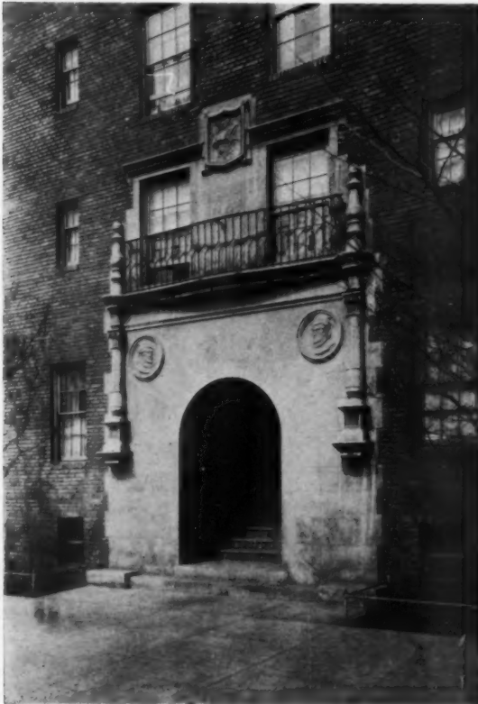
ENTRANCE DETAIL OF APARTMENT HOUSE AT 65TH STREET AND AVENUE A, NEW YORK CITY ANDREW J. THOMAS, ARCHITECT
