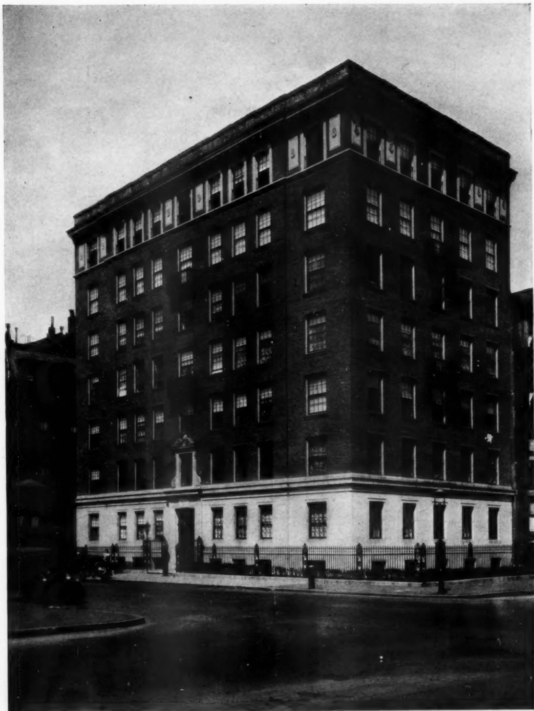
APARTMENT HOUSE AT 301 BERKELEY STREET, BOSTON, MASS.
