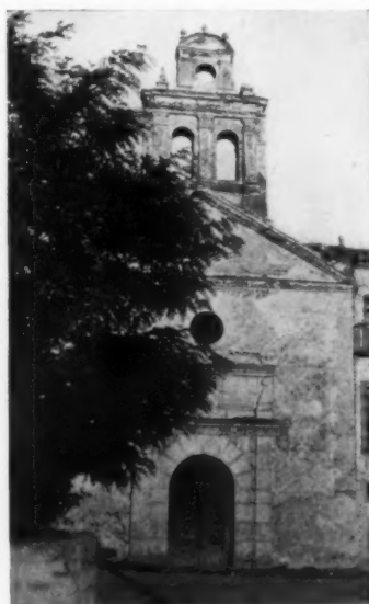
PLASTER WORK, SEGOVIA NOTE STUCCO PATTERN ON WALLS
