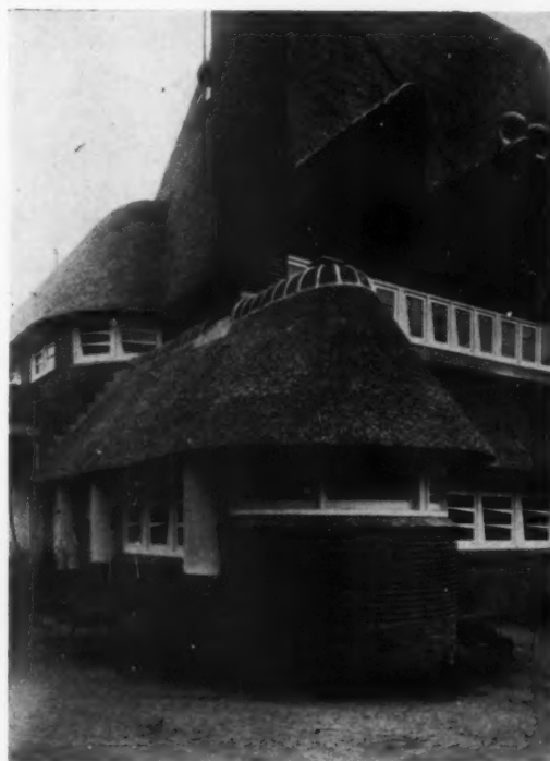
AN EXTERIOR DETAIL
