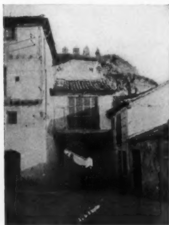
INSIDE OF OLD CITY GATE, SEGOVIA
