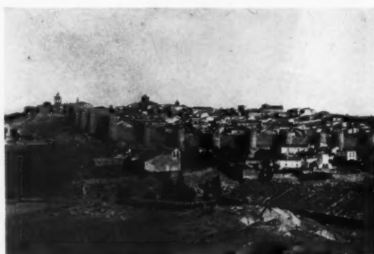
GENERAL VIEW OF AVILA
