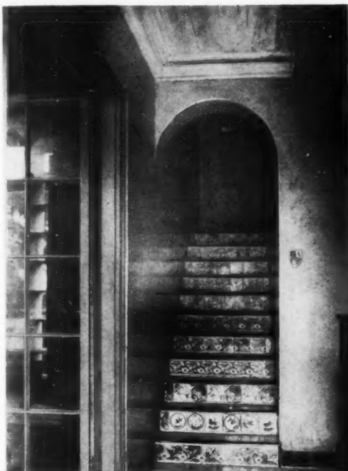
STAIRCASE, WITH TILE RISERS, LEADING TO THE OFFICE OF THE ARCHITECT
