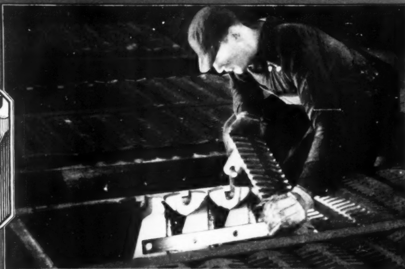
Detail of Heggie-Simplex Individual Grate Brackets
