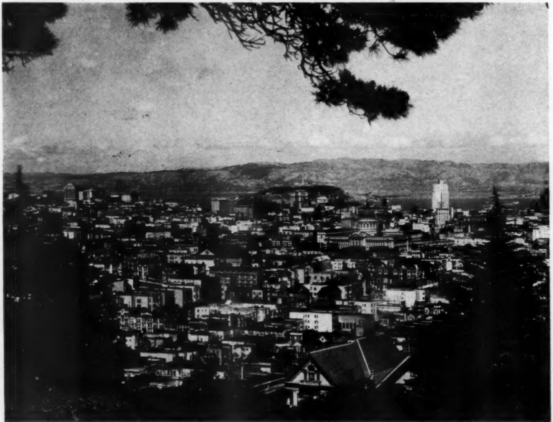
SAN FRANCISCO, CALIFORNIA, SHOWING LOCATION OF TELEPHONE BUILDING
