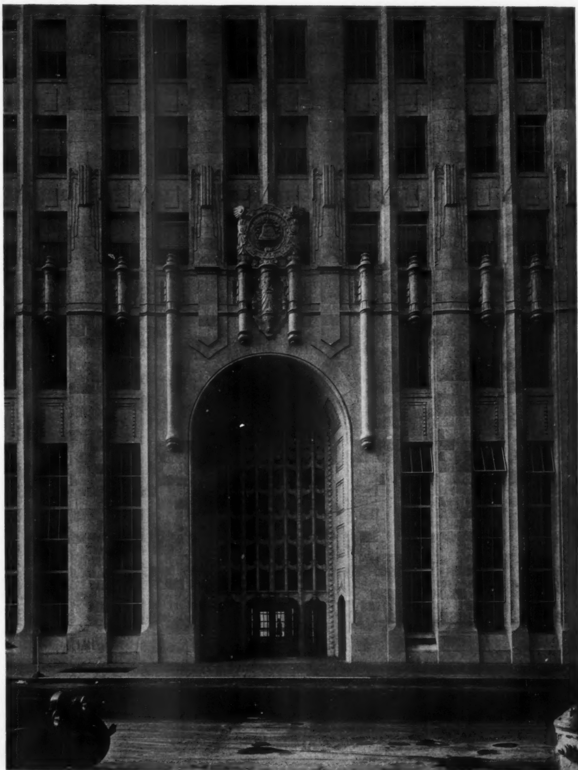
ENTRANCE ON NEW MONTGOMERY STREET, TELEPHONE BUILDING, SAN FRANCISCO, CALIF.
