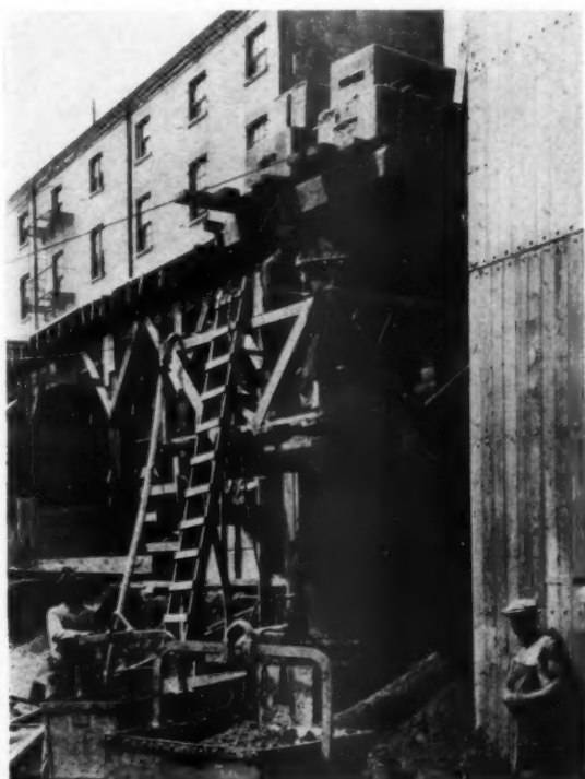
AT LEFT: CIRCULAR CAISSON, 5 FEET IN DIAMETER, BALLASTED WITH 12 TONS OF CAST IRON BLOCKS. AT RIGHT: SECTION THROUGH A FOUNDATION PIER. THE AIR SHAFT AND WORKING CHAMBER WERE FILLED WITH CEMENT AFTER CUTTING EDGES OF CAISSON HAD ENTERED HARD PAN
