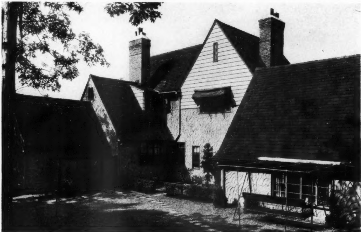
HOUSE OF MRS. E. M. PERLEY, BRONXVILLE, N. Y.—CLIFFORD C. WENDEHACK, ARCHITECT
