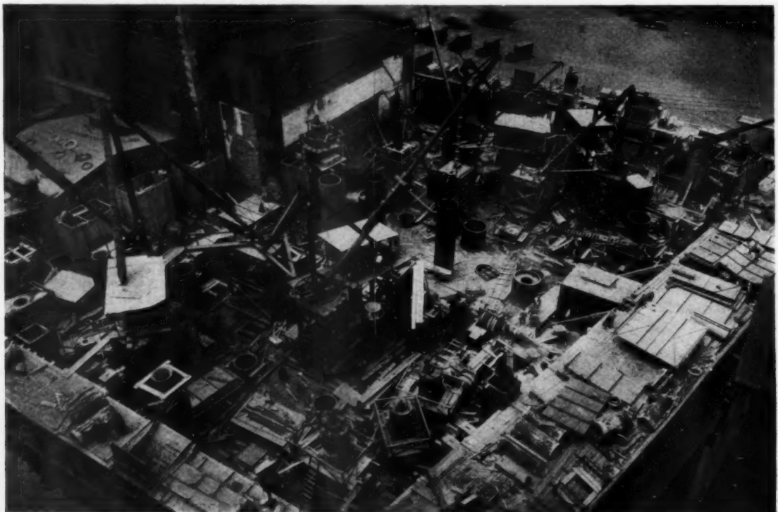
ADVANCED STAGE OF FOUNDATION CONSTRUCTION, JULY 20, 1925. CAISSONS SUNK OR SINKING, COFFERDAMS AND AIR SHAFTS OF OTHERS PROJECTING ABOVE BOTTOM OF CELLAR EXCAVATION. THREE AIR LOCKS IN SERVICE SHOWN IN CENTER FOREGROUND, FOUR OTHERS IN BACKGROUND. WOODEN COFFERDAMS ARE SEEN AT LEFT
