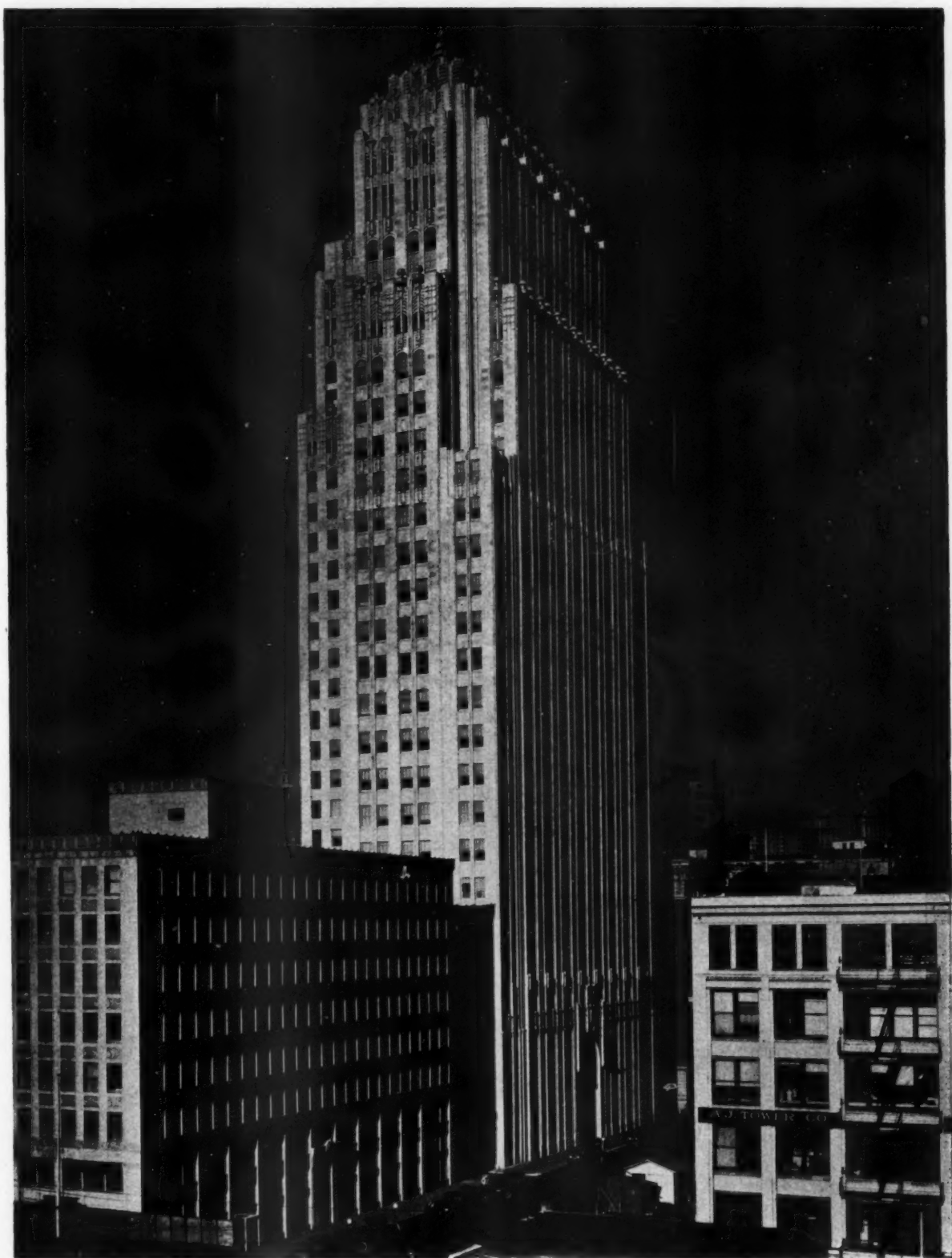
NATOMA AND MONTGOMERY STREET FACADES, TELEPHONE BUILDING, SAN FRANCISCO, CALIF.
