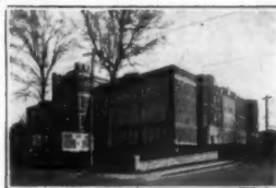
Thanks to the far-seeing judgment of school board, superintendent and architect in installing "THE AMERICAN SYSTEM" of Heat-with-Ventilation in THE ROANOKE SENIOR HIGH SCHOOL (above) and THE ROANOKE
