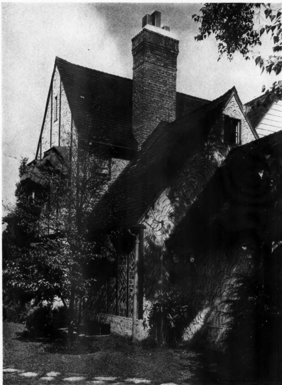
HOUSE OF MRS. E. M. PERLEY, BRONXVILLE, N. Y.—CLIFFORD C. WENDEHACK, ARCHITECT
