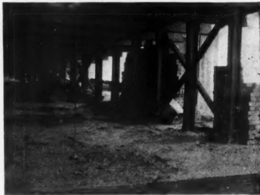
VIEW UNDER THE TANK SHOWING ACCESSIBILITY FOR INSPECTION, REPAIRS AND THE SUPPORTING COLUMNS
