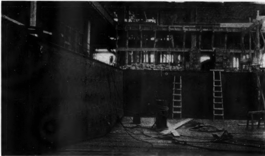
VIEW OF SWIMMING POOL DURING PROCESS OF ARC ELECTRIC WELDING THE SEAMS. THE FOUR ELECTRIC CONTROL PANELS ARE SHOWN AT THE LEFT TOP OF THE TANK SWIMMING POOL, NEW UNION LEAGUE CLUB, CHICAGO, ILL.—MUNDIE & JENSEN, ARCHITECTS
