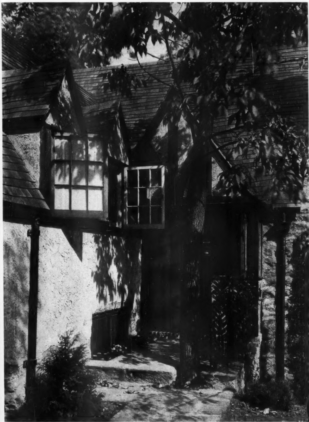
HOUSE OF E. PONCHELET, RIVERDALE, N. Y.—FRANK J. FORSTER, ARCHITECT
