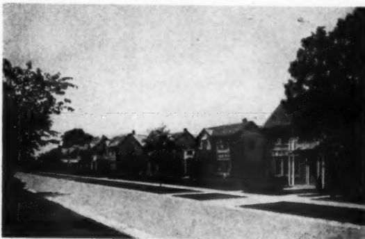
GROUP OF HOUSES ON CHURCH STREET
