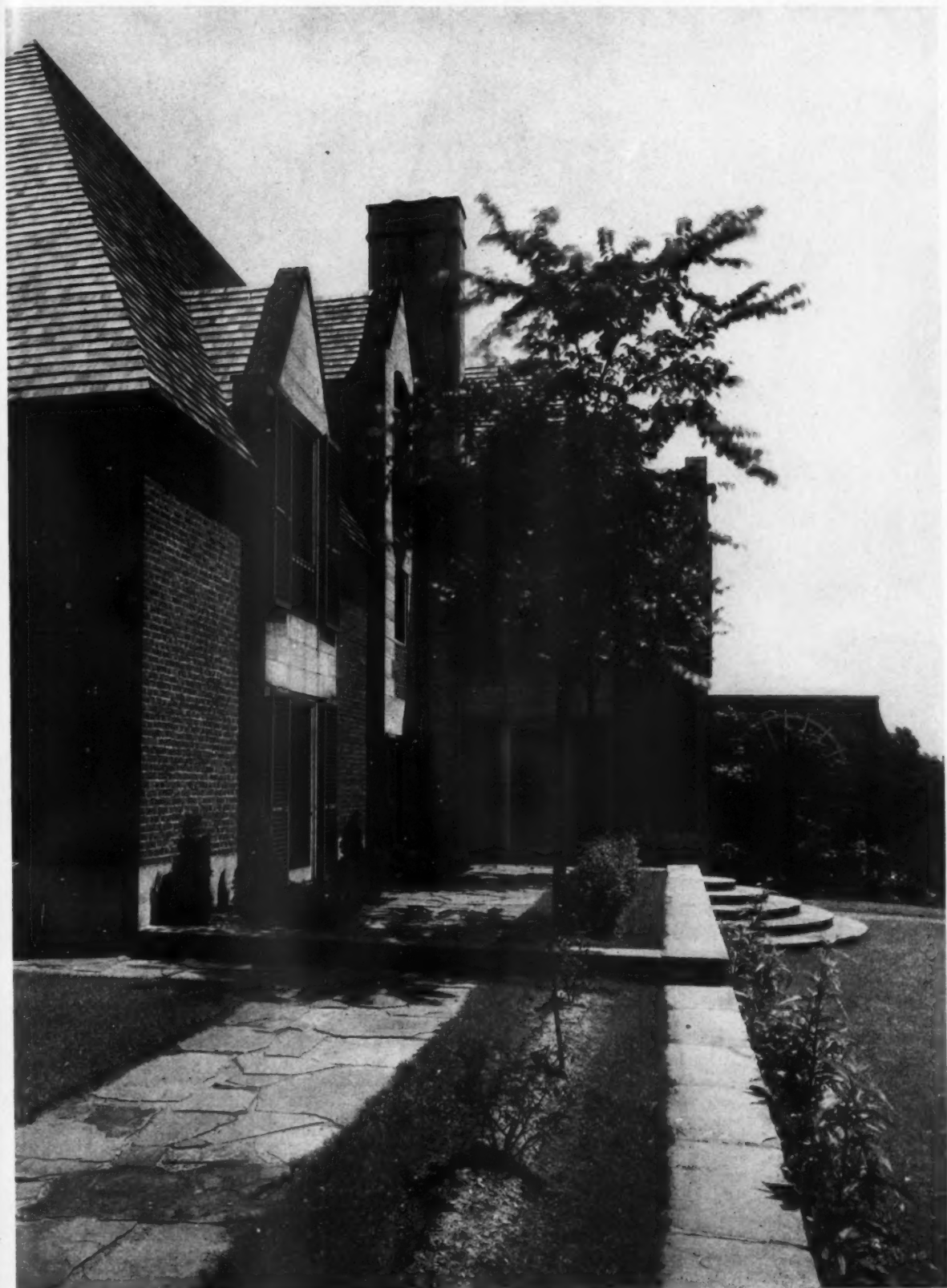
HOUSE AND GARDEN OF CARL E. SIEBECKER, BETHLEHEM, PA.—MELLOR, MEIGS & HOWE, ARCHITECTS
