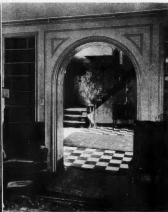
LOOKING FROM LIBRARY INTO RECEPTION HALL
