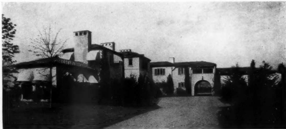
GENERAL VIEW OF THE EXTERIOR, WITH THE LOGGIA IN THE RIGHT FOREGROUND
