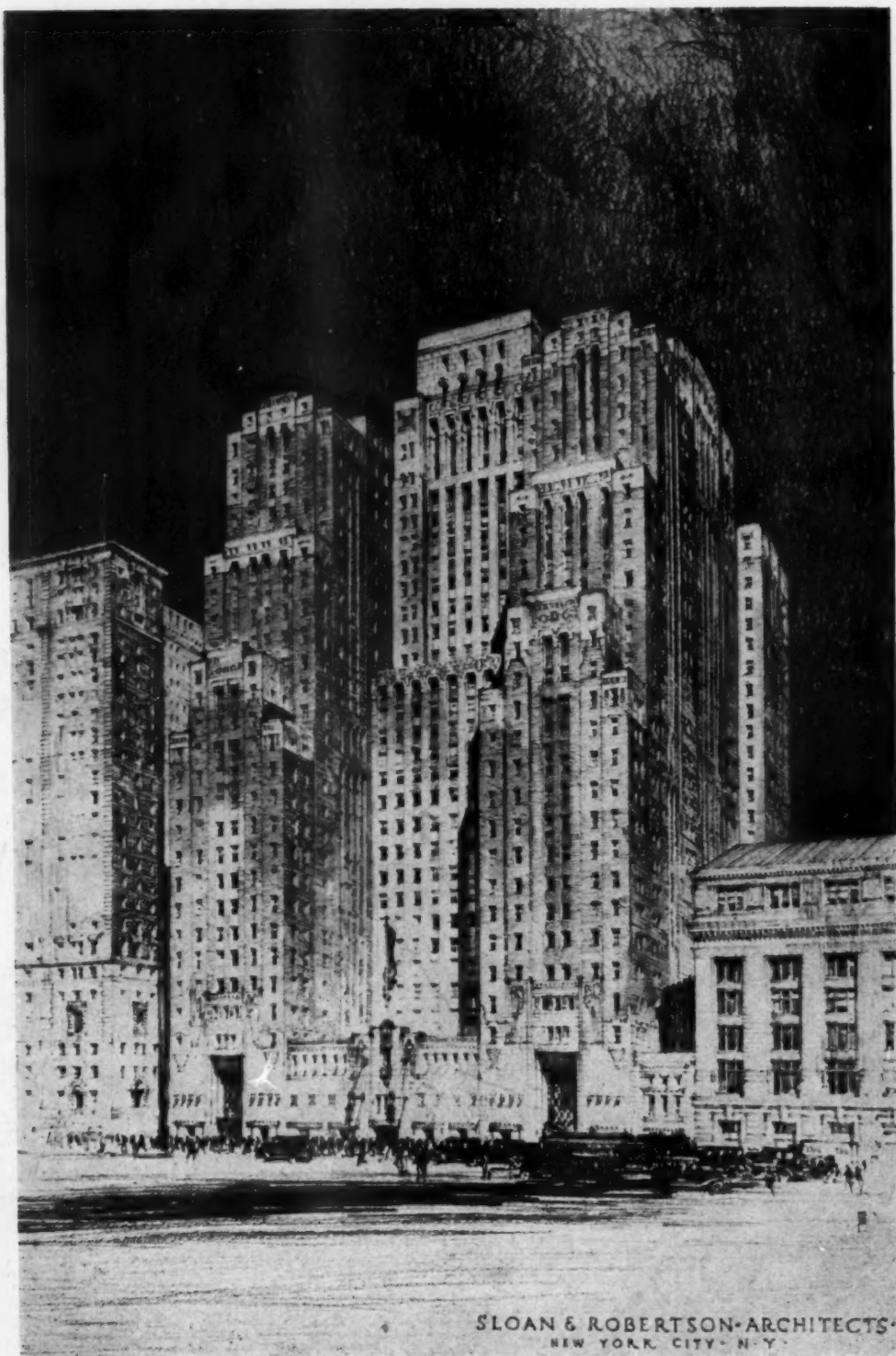
EASTERN TERMINAL OFFICE BUILDING, NEW YORK
