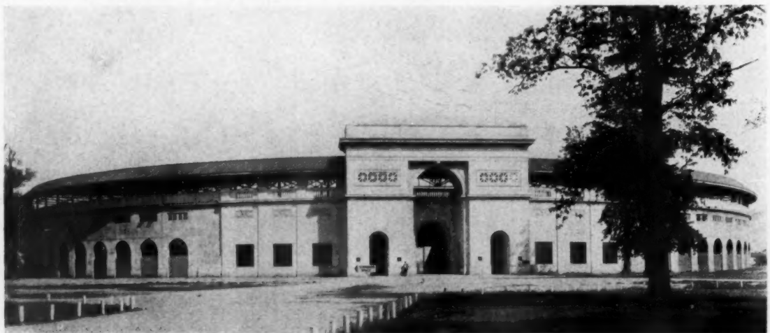
PRINCIPAL FACADE, TERRE HAUTE MEMORIAL STADIUM
