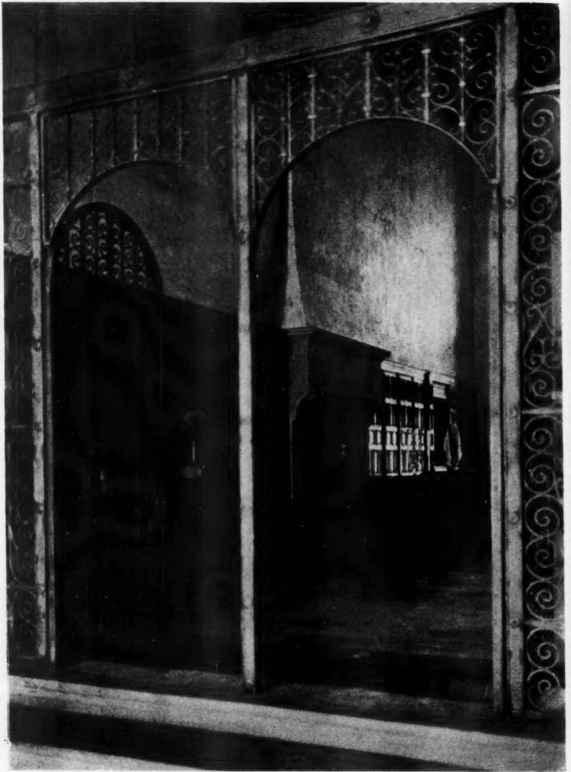
DETAIL OF WROUGHT IRON GRILLE OPENING FROM THE FOYER TO THE SHOP THE I. MAGNIN AND COMPANY SHOP, HOLLYWOOD, CALIF.—MYRON HUNT, ARCHITECT
