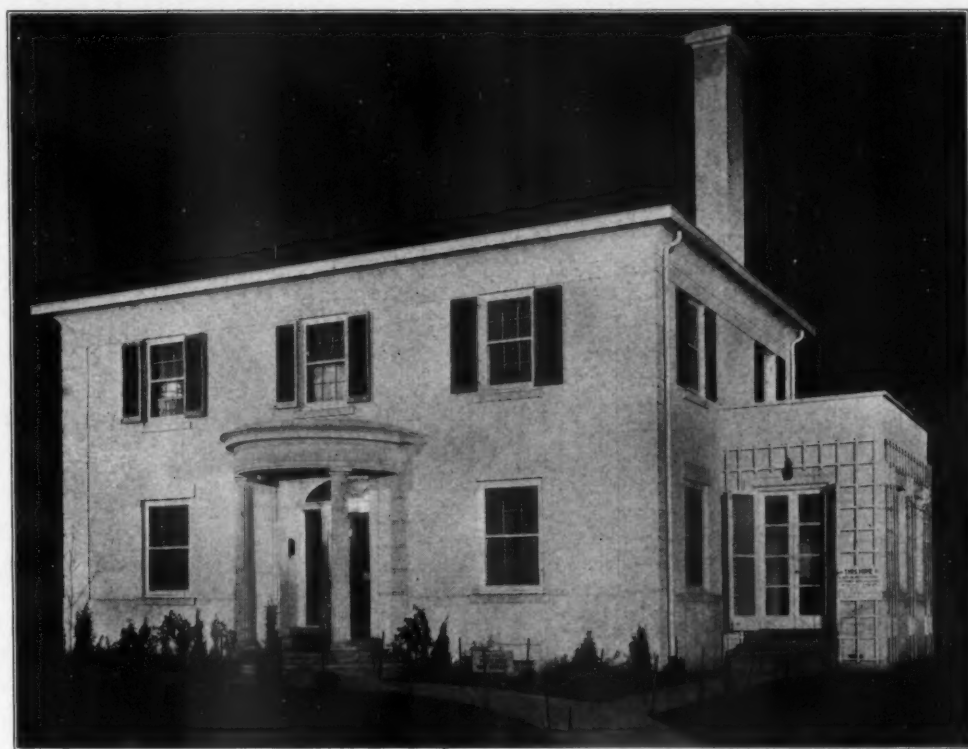
Lighted by four No. 1045-AC Pyle-O-Lytes, each with 250 watt lamp,
