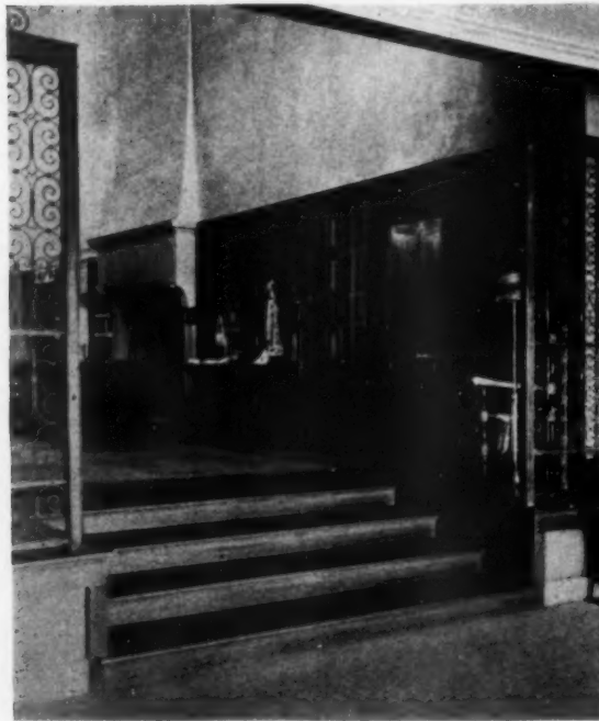
THE SALESROOM AT THE REAR IS APPROACHED BY THE WALLS OF THE SHOP, FLANKED ON EITHER SIDE BY WROUGHT IRON PANELS
