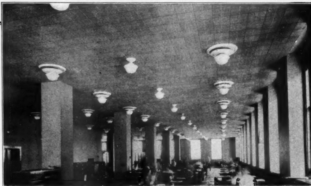
Office in Federal Reserve Bank, Cleveland, Ohio. Walker & Weeks, Architects. Fifteen thousand square feet Acousti-Celotex, Type C, used on ceiling for sound quieting. Installed by George P. Little Co., Inc., Cleveland, approved Acousti-Celotex contractor
