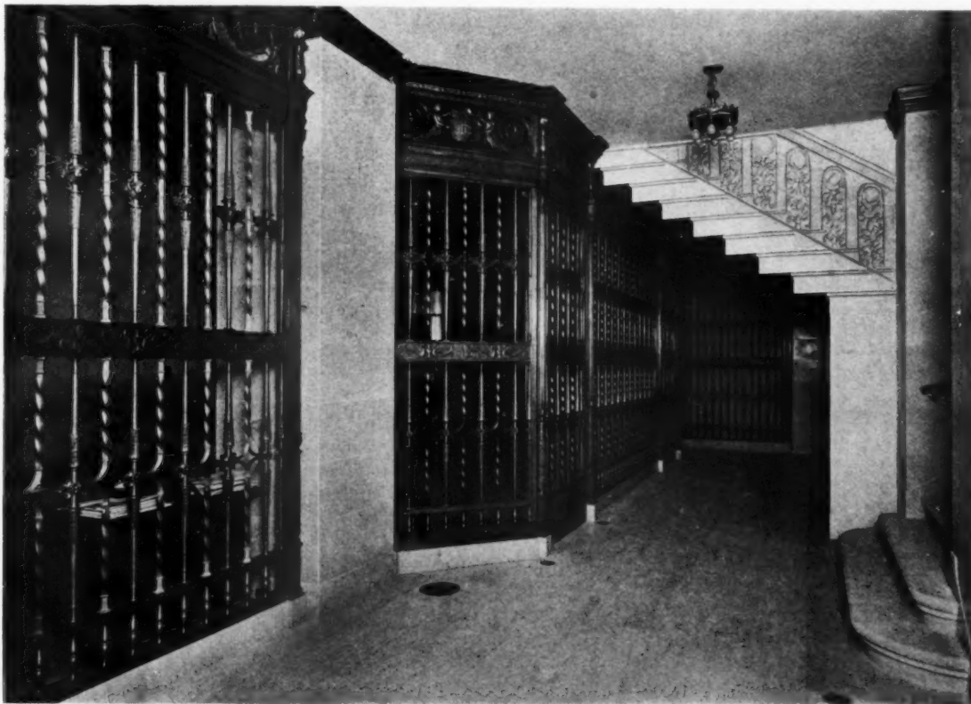
SAFE DEPOSIT VAULTS
