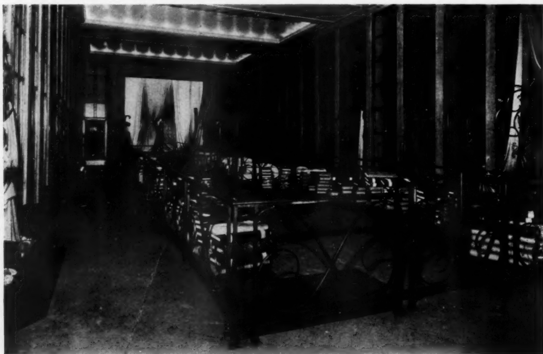
CHENEY BROTHERS' NEW STORE, NEW YORK CITY HOWARD GREENLEY, ARCHITECT
