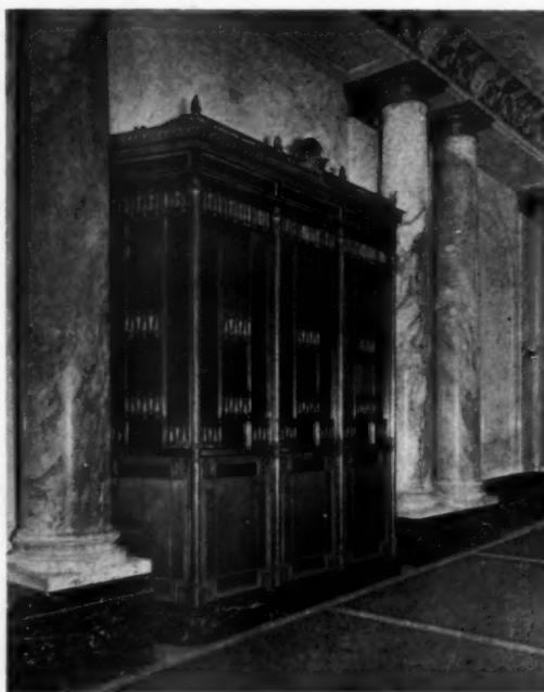
Ticket booth in the Albee Theatre, Brooklyn, New York, illustrating the use of Anaconda Extruded Bronze in combination with bronze castings. Thomas W. Land, New York, architect, William H. Jackson Company, New York, fabricators.
