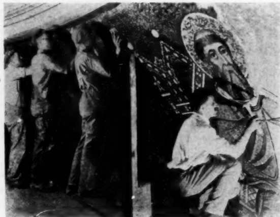
INSTALLING THE MOSAIC, AND REMOVING THE PAPER
