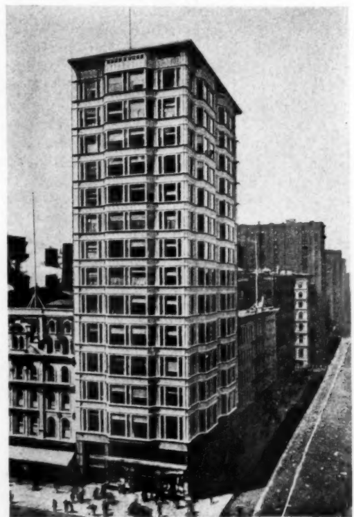
RELIANCE BUILDING, CHICAGO, ILL. ENAMELED TERRA COTTA FRONTS. THIS WAS THE FIRST LARGE BUILDING ERECTED WITH ENAMELED FRONTS
