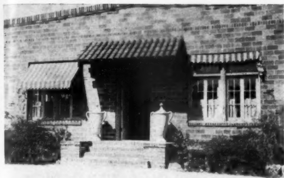
MAIN ENTRANCE TO OFFICES
