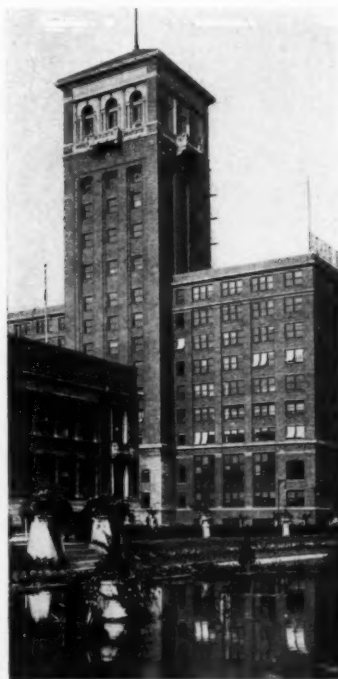
A GROUP OF WATER TOWERS OF INDUSTRIAL BUILDINGS WHICH ENCLOSE THE SPRINKLER TANKS AND WHICH FORM THE DOMINATING ARCHITECTURAL FEATURE OF THE DESIGN IN EACH CASE
