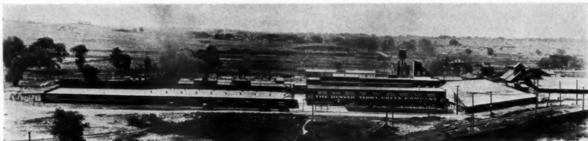
WESTERN PLANT OF THE NORTHWESTERN TERRA COTTA COMPANY, AT DENVER
