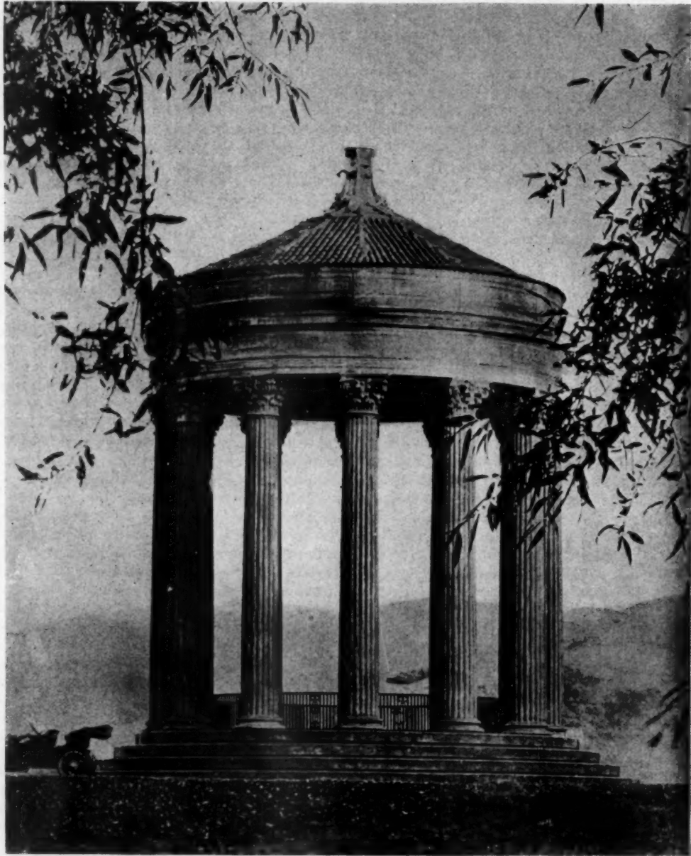
WATER TEMPLE FOR SPRING VALLEY WATER COMPANY, SUNOL, CALIF.
