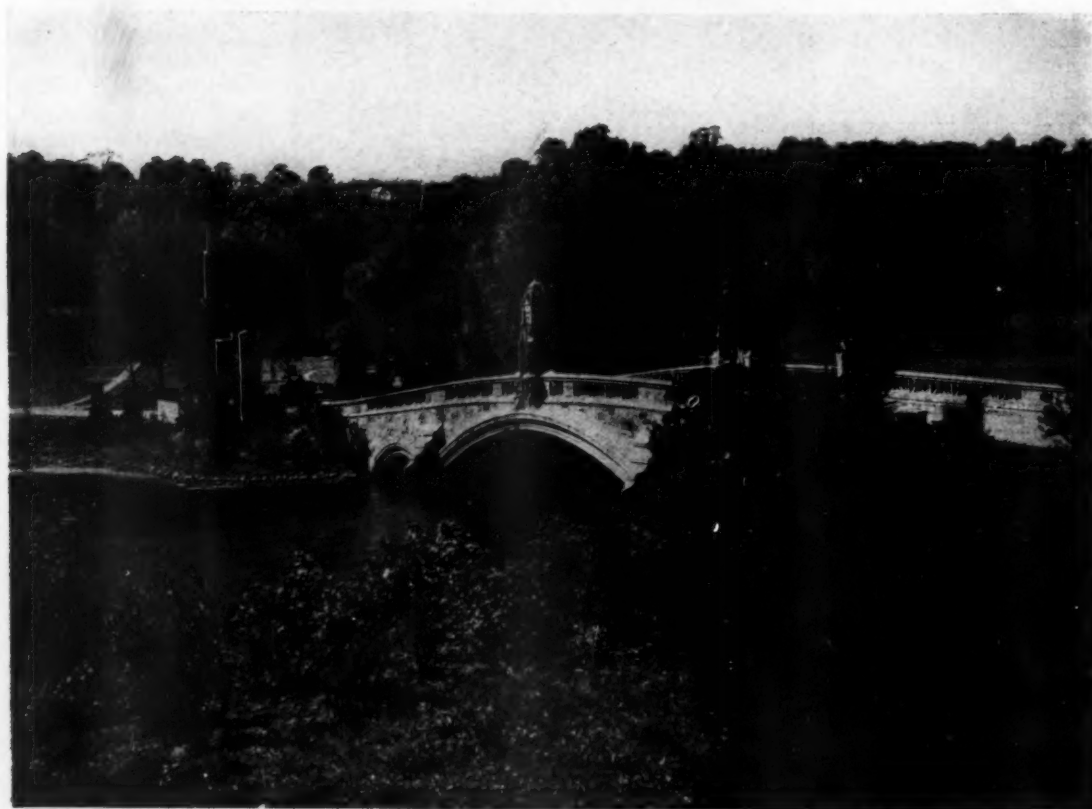
BRIDGE IN CEMETERY OF THE GATE OF HEAVEN, MT. PLEASANT, N. Y.
