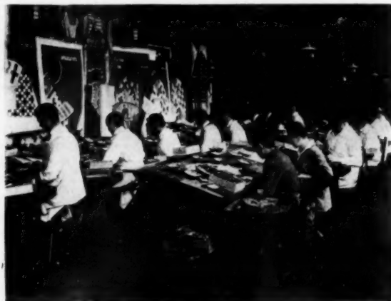
CHIPPING THE STRIPS PREPARATORY TO SETTING
