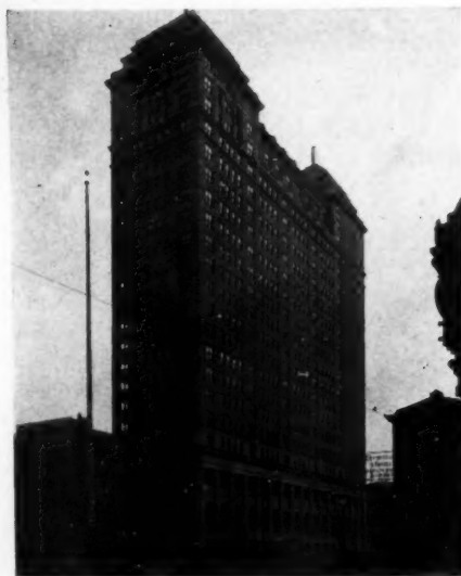
LIBERTY BANK OF BUFFALO, N. Y. ALFRED C. BOSSOM, ARCHITECT JOHN J. GILL AND SON, BUILDERS
