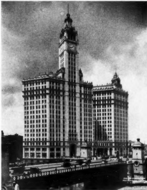
THE TWIN WRIGLEY BUILDINGS, CHICAGO. THESE MODERN BUILDINGS ARE FACED ON ALL SIDES WITH ENAMELED TERRA COTTA. GRAHAM, ANDERSON, PROBST & WHITE, ARCHITECTS.
