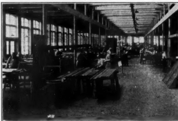
ASSEMBLING FLOOR—ARCHITECTURAL FITTING SHOP
