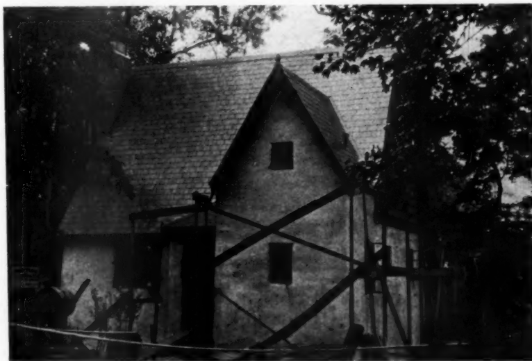
HOUSE AT SCARSDALE, NEW YORK—HARRISON GILL, ARCHITECT AND BUILDER WALLS OF HOUSE ERECTED IN THREE AND ONE-HALF DAYS BY ONE MECHANIC AND TWO LABORERS
