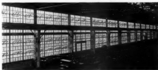
Typical Installation of Truscon Std. Windows
