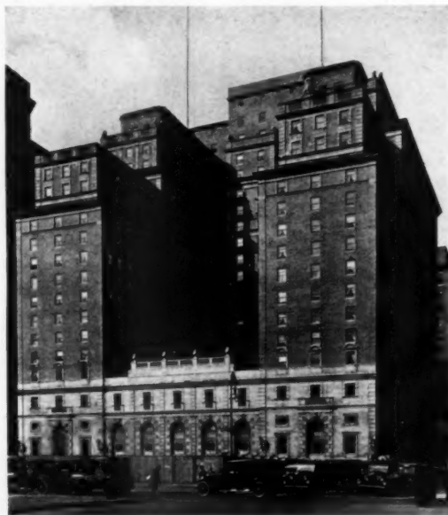
HOTEL ROOSEVELT, NEW YORK GEORGE B. POST & SONS, ARCHITECTS
