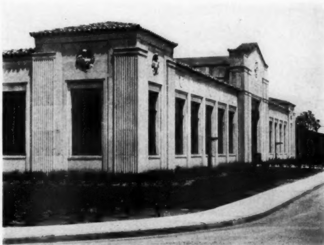
DETAIL OF END OF BUILDING
