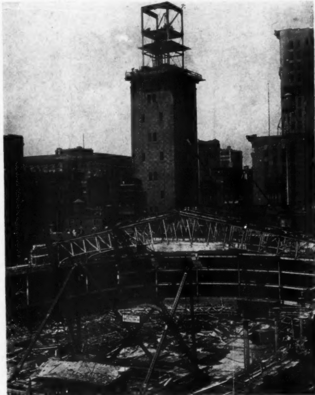
THREE STORIES OF THE TOWER AND A LARGE PORTION OF THE ROOF OVER THE ARENA REMOVED. THE PHOENIX COLUMNS WHICH SUPPORTED THE ROOF TRUSSES ARE SEEN IN THE FOREGROUND. ALL STEELWORK SHOWN IN THE ILLUSTRATION, THOUGH UNPROTECTED, WAS IN GOOD CONDITION. MUCH OF IT WILL BE USED AGAIN
