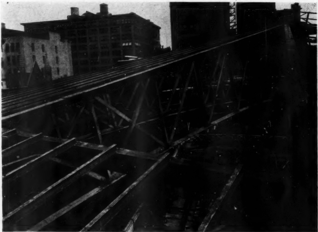
RADIAL ROOF TRUSSES OVER THE ARENA IN POSITION AS EXPOSED BY THE REMOVAL OF THE ROOF COVERING AND SHEATHING BOARDS. THIS PORTION OF THE STEELWORK WAS IN EXCELLENT CONDITION
