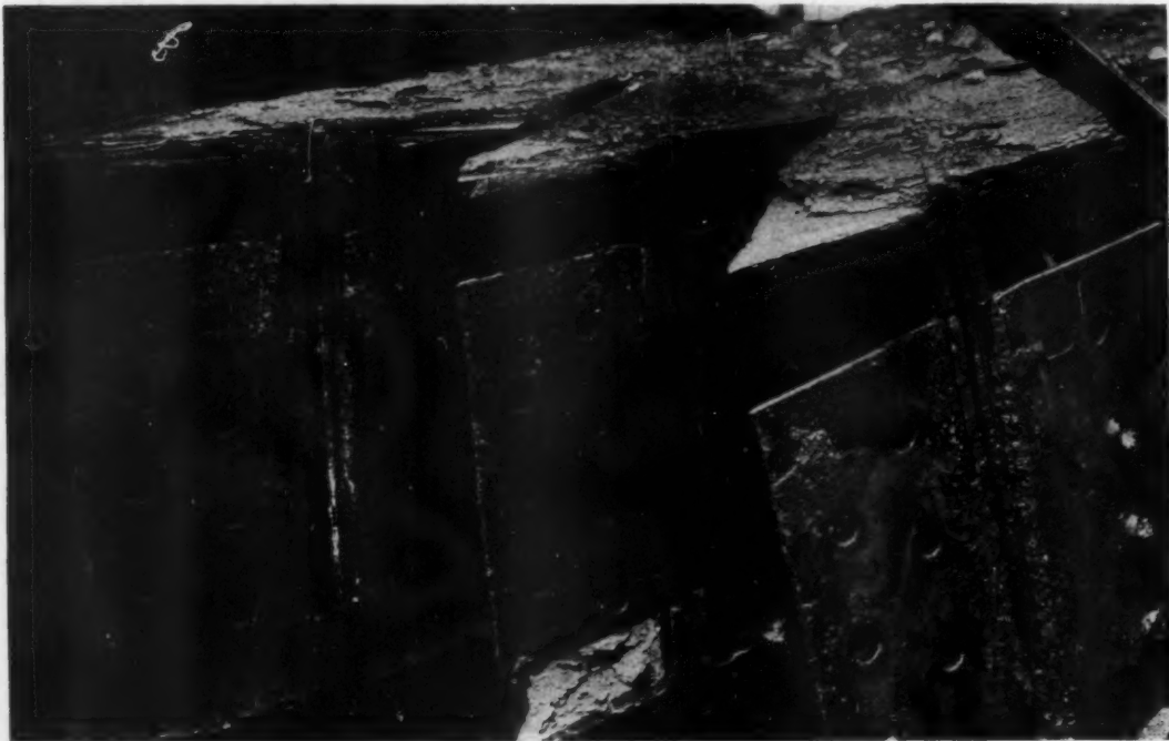
SHORT CORNER GIRDERS IN THE OCTAGONAL FRAMEWORK SUPPORTING THE LOWER DRUM OF THE UPPER TOWER OF MADISON SQUARE GARDEN. NOTE THE THIN SHEET OF METAL PROJECTING FROM THE CORRODED LAMINATION OF HORIZONTAL LEGS OF FLANGE ANGLES AND THE DEFINITE LAMINATIONS DEVELOPED IN BOTH LEGS OF THE ANGLES. THE HITCH ANGLES ARE IN GOOD CONDITION. THE PATCHES ON THEM, NOTED IN THE ILLUSTRATION, ARE CEMENT AND MORTAR. RIVETS WERE IN EXCELLENT CONDITION
