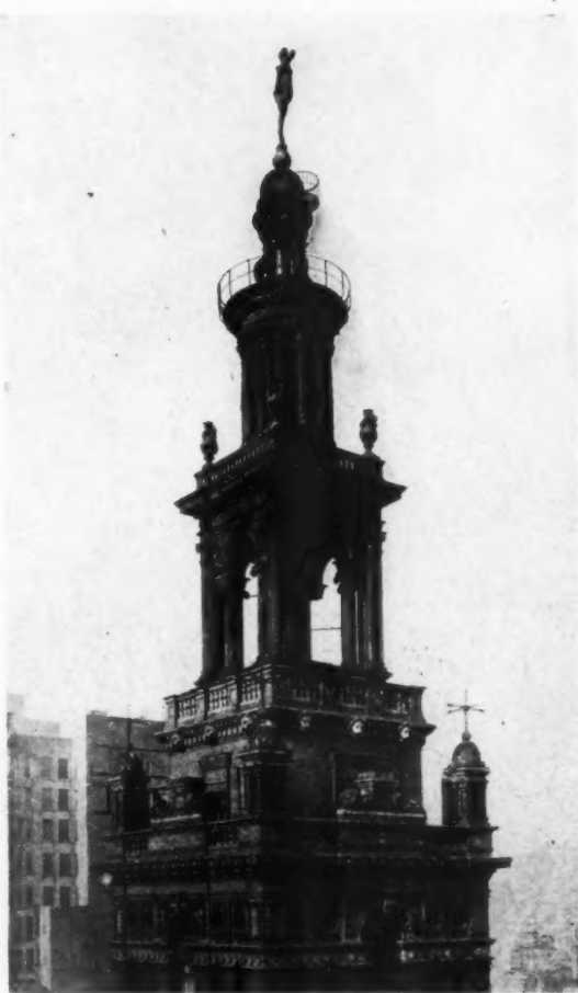
UPPER PORTION OF THE TOWER OF MADISON SQUARE GARDEN BEFORE DEMOLITION WAS BEGUN. THE PORTION ABOVE THE BRICKWORK WAS BUILT OF STRUCTURAL STEEL COVERED WITH COPPER, AS SHOWN ON FOLLOWING PAGE. IT WAS IN THIS POSITION THAT THE STEELWORK WAS SLOWLY BEING DESTROYED
