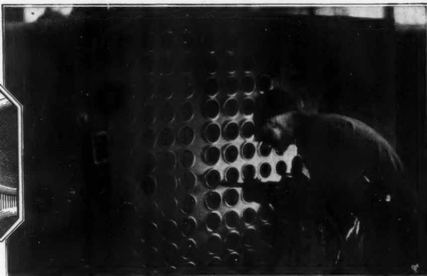
Expanding and beading make tubes water-tight.
