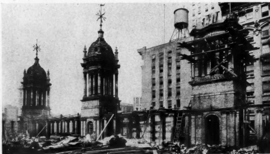
ROOF GARDEN DURING DEMOLITION AUGUST, 1925
