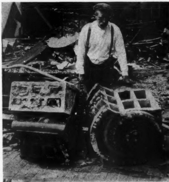
TYPICAL PIECE OF TERRA COTTA SLIGHTLY DAMAGED IN WRECKING BUT OTHERWISE IN GOOD CONDITION. NOTE THE THICK WEBS AND VOIDS SOLIDLY FILLED WITH BRICKS AND MORTAR. THE FLOOR OF THE ROOF GARDEN WAS OF BRICK LAID FLAT AND GROUTED
