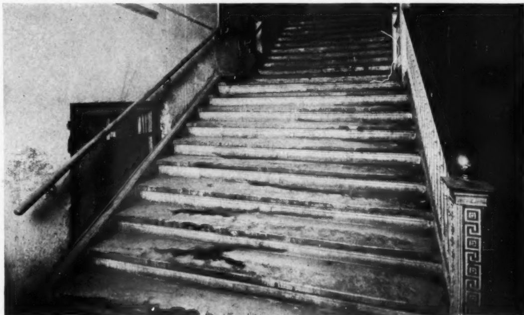
BALCONY STAIRWAYS OF THE ARENA WERE BUILT OF IRON WITH SLATE TREADS AND PLATFORMS AND IRON RISERS. NORMAL WEAR WILL BE NOTED ON THE EXTREME EDGE OF THE TREADS IN LINES OF TRAVEL
