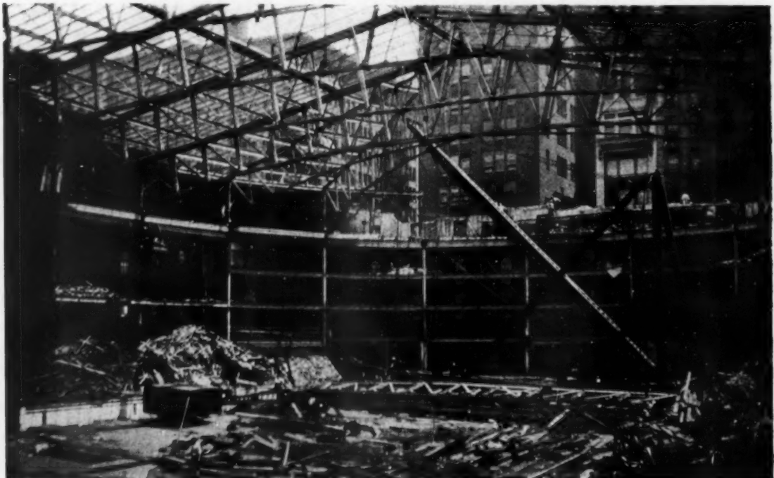
DIANA SURMOUNTING THE TOWER OF MADISON SQUARE GARDEN WAS REMOVED MAY 6, 1925, AND MARKED THE ACTIVE BEGINNING OF DEMOLITION. THE ABOVE VIEW OF THE ARENA WAS TAKEN ON JUNE 3, 1925
