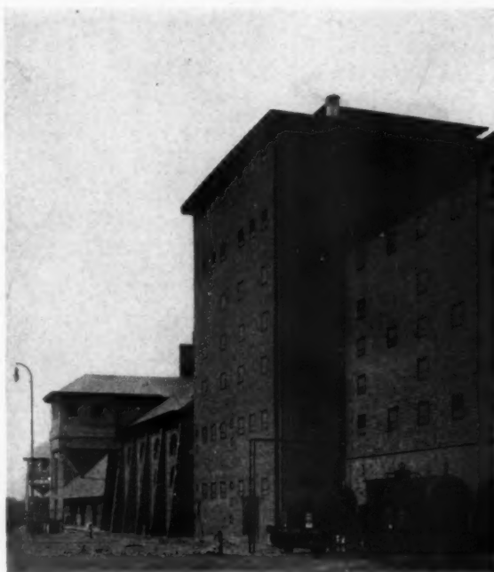
CHEMICAL PLANT, LUBAN
