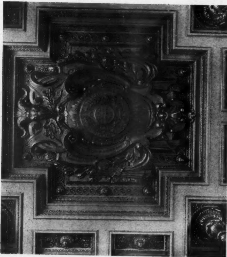
CARTOUCHE IN CEILING OF ENTRANCE VESTIBULE AT RIGHT: BUILDING ILLUMINATED AT NIGHT
