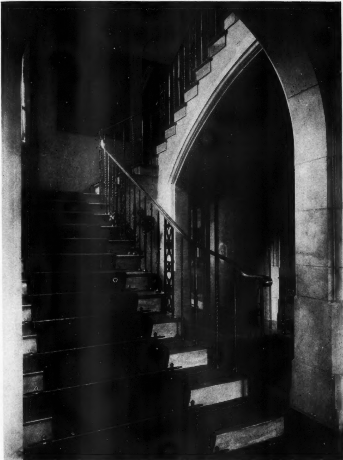
A simple wrought iron balustrade emphasizes the structural features of the main staircase HOUSE OF H. E. MANVILLE, PLEASANTVILLE, N. Y.—DONN BARBER, ARCHITECT
