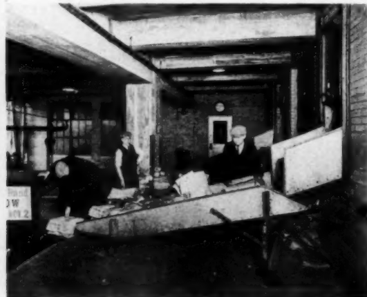
THE CHUTES THROUGH WHICH THE BUNDLED PAPERS ARE DELIVERED TO THE TRUCKS AT THE LOADING DOCK. THE SHIPPING PLATFORM IS IMMEDIATELY BELOW THE MAILING ROOM. THE RECESSED DRIVEWAY AND PARKING SPACE PREVENT BLOCKING THE ALLEY
