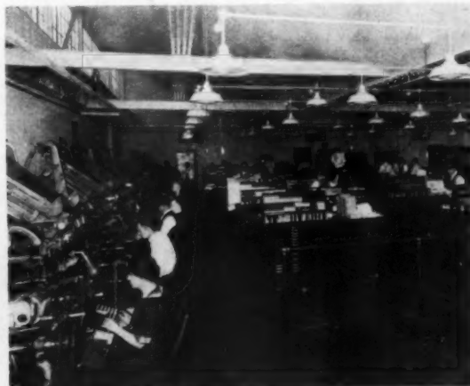
ONE MACHINE ALLEY IN THE LINOTYPE ROOM WHERE THE TYPE IS SET. TWENTY-TWO LINOTYPE MACHINES ARE CONVENIENTLY RANGED TO ALLOW PLENTY OF ELBOW ROOM FOR EACH OPERATOR
