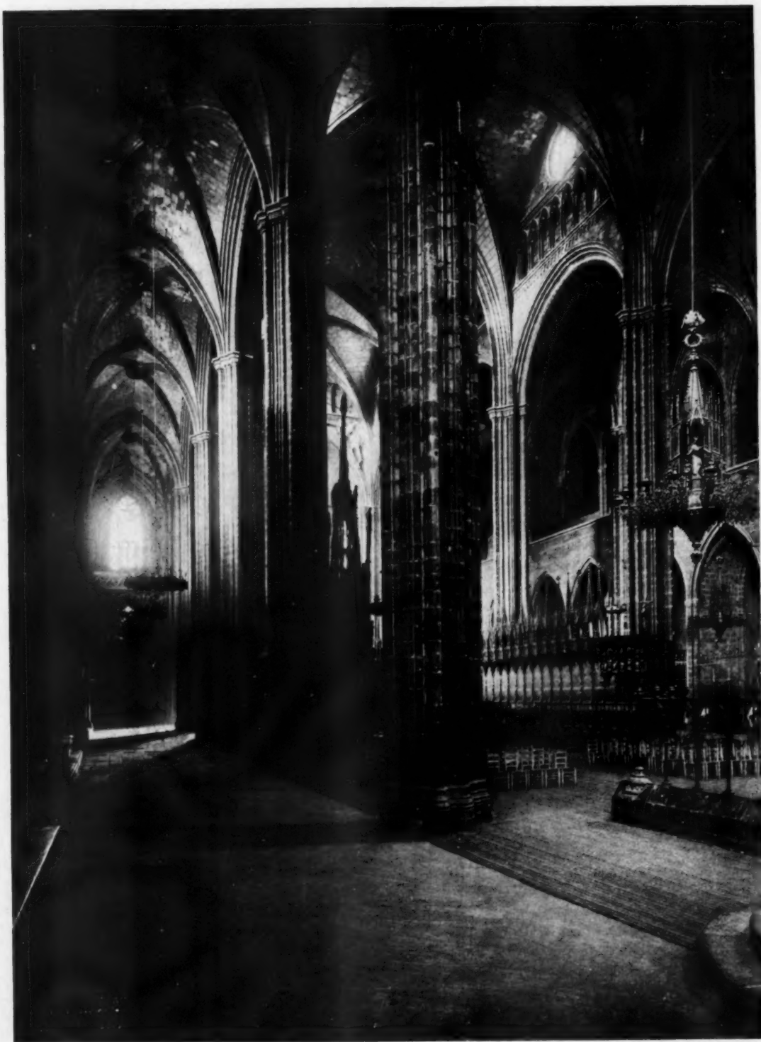
LOOKING ACROSS THE NAVE BARCELONA CATHEDRAL (Clasé Arriu Mas)
