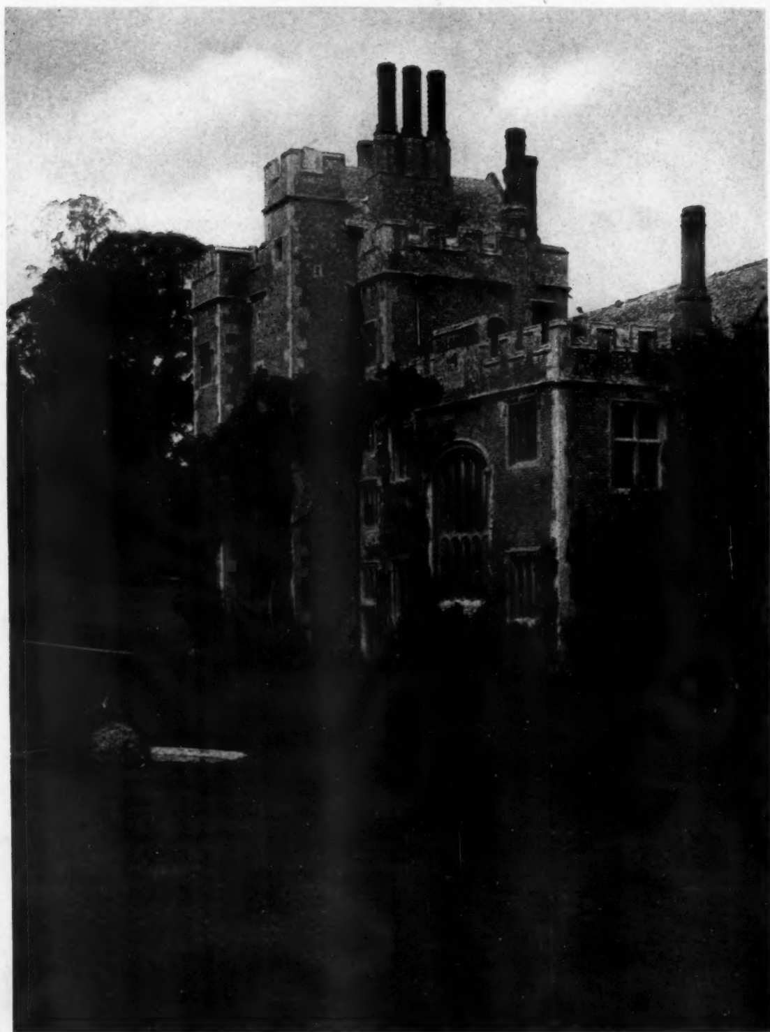
COMPTON WYNYATES MANOR HOUSE, WARWICKSHIRE, ENGLAND
