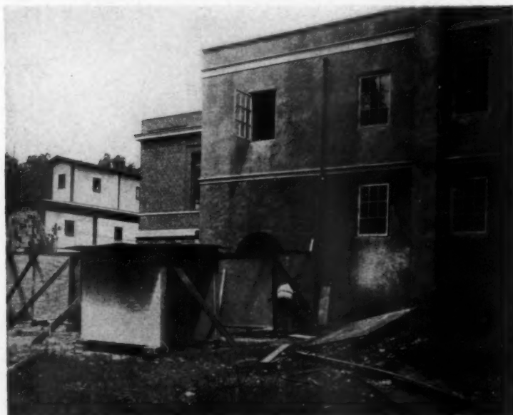
FIG. 2. VIEW OF THE REAR OF THE SOUND LABORATORY OF THE NATIONAL BUREAU OF STANDARDS, WASHINGTON, D. C., SHOWING THE CONSTRUCTION OF THE PANELS FOR TEST TO THE SIDE AND REAR OF THE CHAMBER
