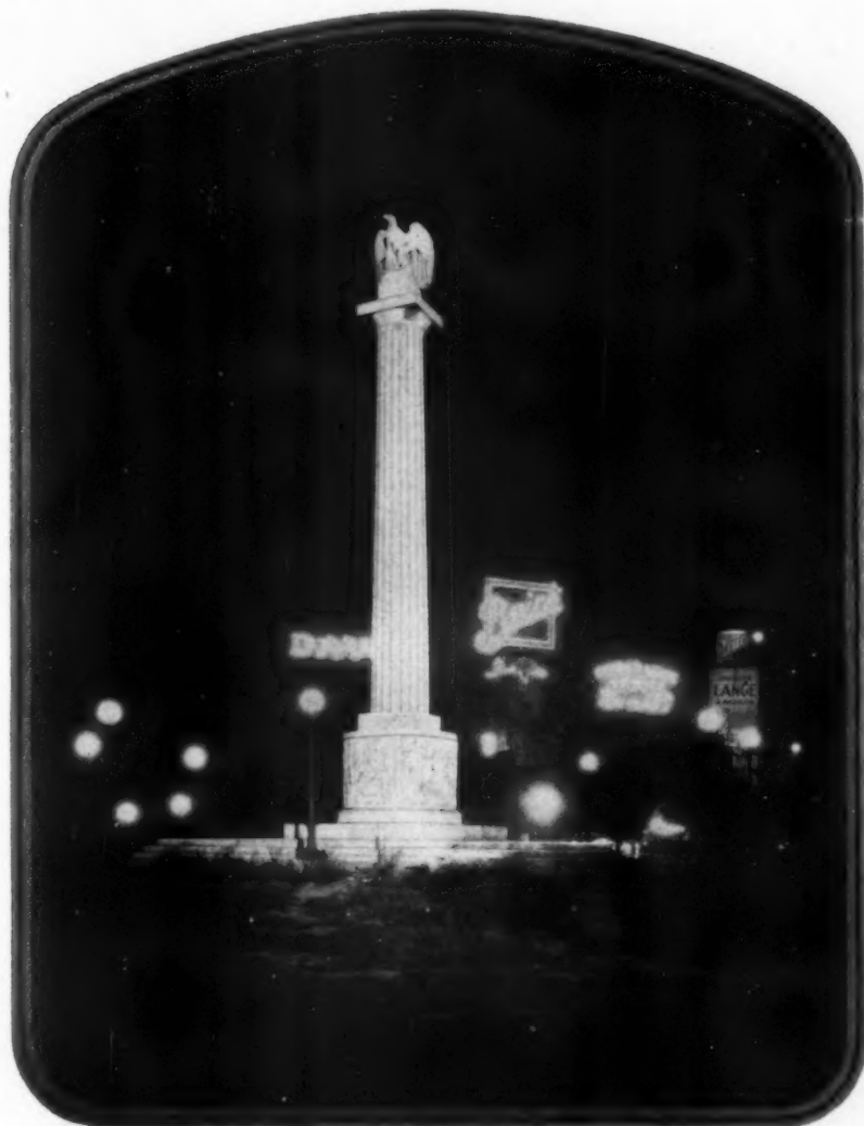
The Logan Monument, Chicago, illuminated by one 23" Pyle-O-Lyte. Note that this floodlight can be controlled to give the tall, narrow beam required to pick out the shaft without spilling light over the surroundings.
