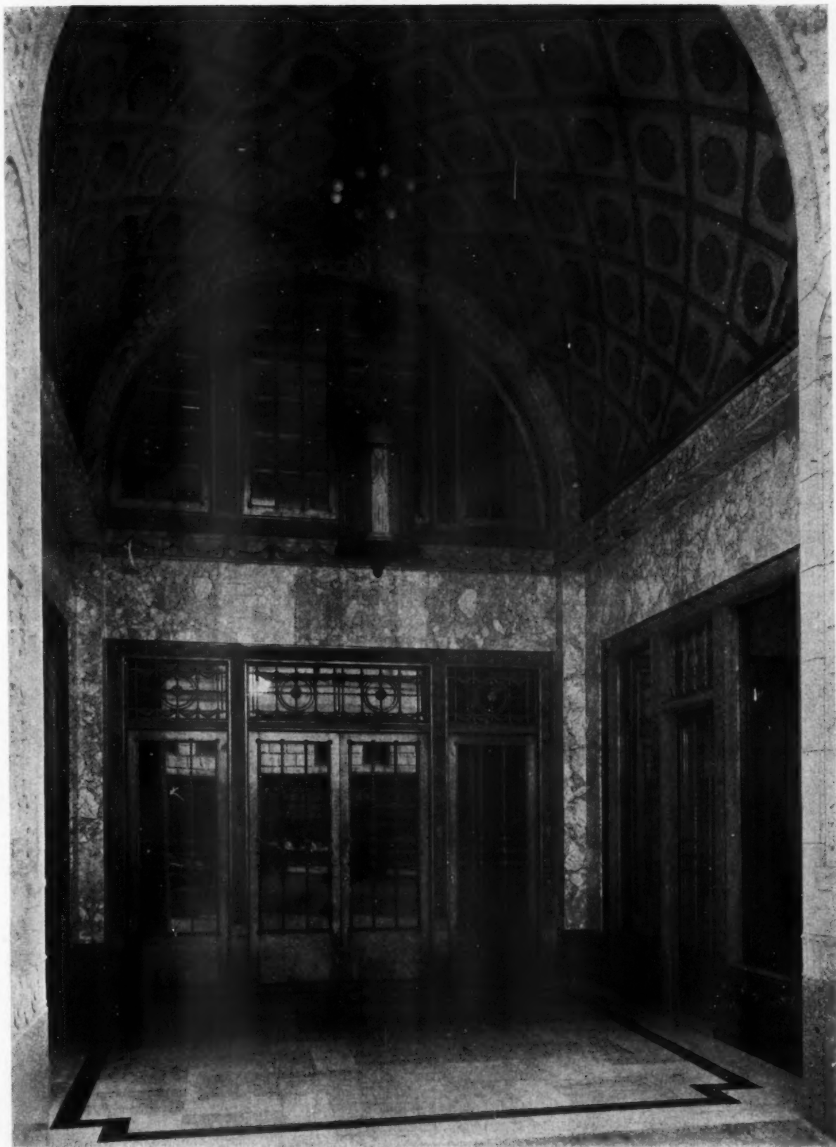
MEDICAL OFFICE BUILDING, SEATTLE, WASHINGTON
