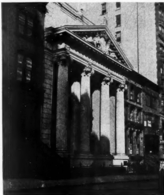
GOOD WORK BY AN ARCHITECT SPOILED BY AN ENVIRONMENTAL FRAME
