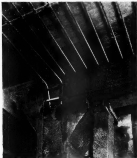
REINFORCING PLACED ON THE CORRIDOR CEILINGS OF SCHOOL NO. 68, BUFFALO, N. Y. THE ENDS OF THE BARS ARE ATTACHED TO THE HORIZONTAL BAR NEAR THE LOWER EDGE OF THE GIRDER. HEAD OF THE RECONSTRUCTED COLUMN SHOWN AT THE LEFT
