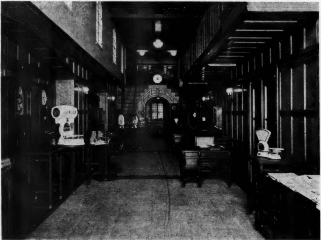
THE DECORATIVE SCHEME OF THE MAIN DISPLAY ROOM INCLUDES AN OAK PANELLED WAINSCOT, A PLASTER CEILING OF NEUTRAL TINT AND A TRAVERTINE FLOOR
