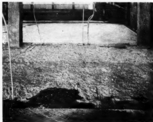
VIEW IN SCHOOL NO. 68, BUFFALO, N. Y., SHOWING THE REFINISHED CLASSROOM FLOORS AND THE OLD CONCRETE TOP REMOVED FROM THE CORRIDOR FLOORS TO RECEIVE THE GUNITE
