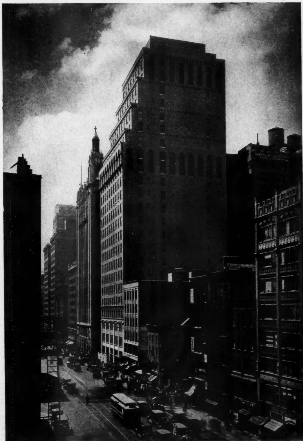
VIEW LOOKING SOUTH BUILDING NO. 550 SEVENTH AVENUE, NEW YORK BUCHMAN & KAHN, ARCHITECTS
