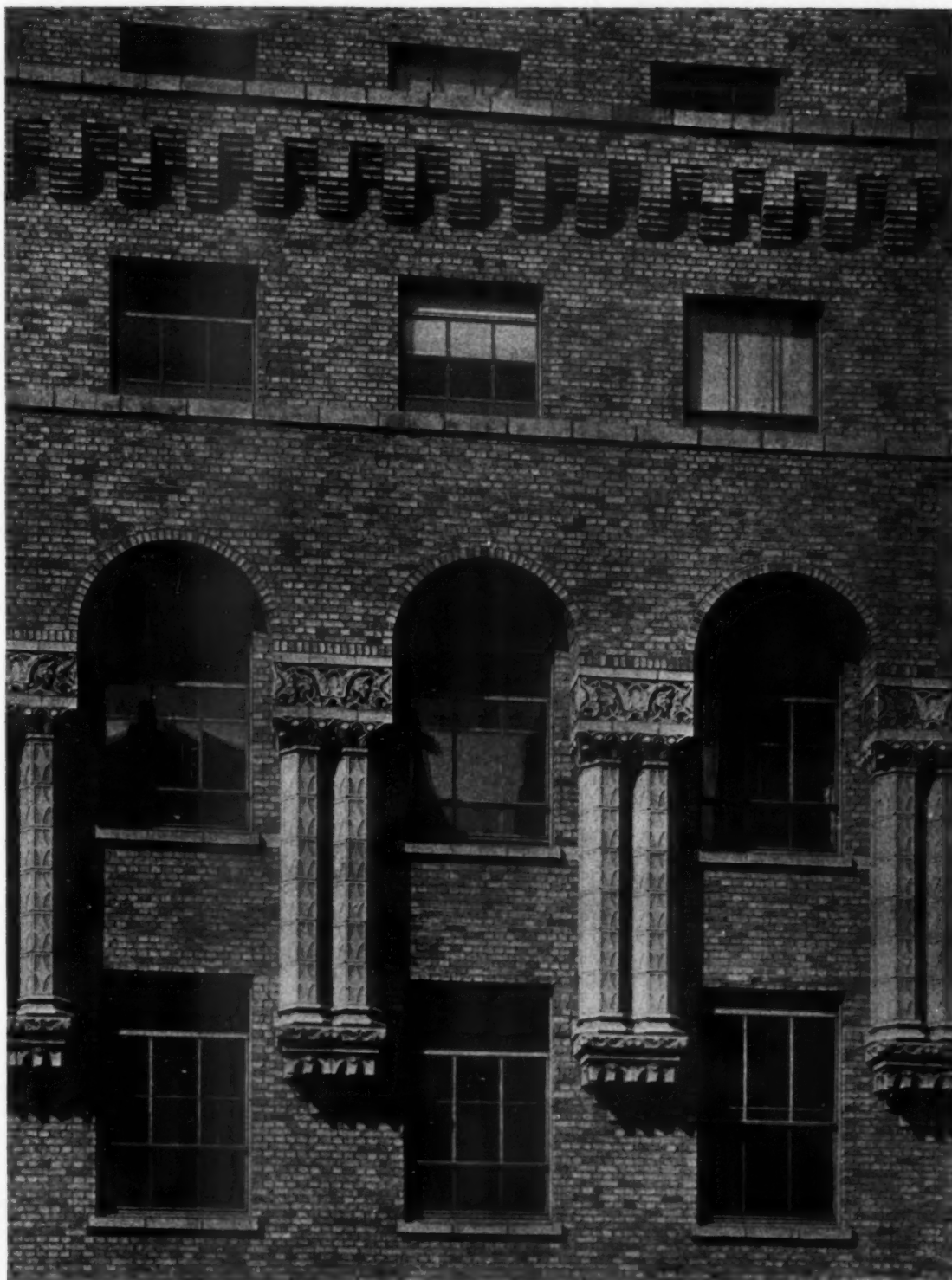
DETAIL OF UPPER STORIES BUILDING NO. 550 SEVENTH AVENUE, NEW YORK BUCHMAN & KAHN, ARCHITECTS
