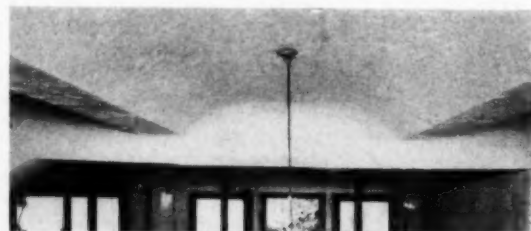
THE RECONSTRUCTED FLOOR SYSTEM OF THE HEARD BUILDING, PHOENIX, ARIZONA, SHOWING THE GUNITE ARCH, WHICH STRENGTHENS THE ORIGINAL FLOOR PANEL, BETWEEN THE BEAMS
