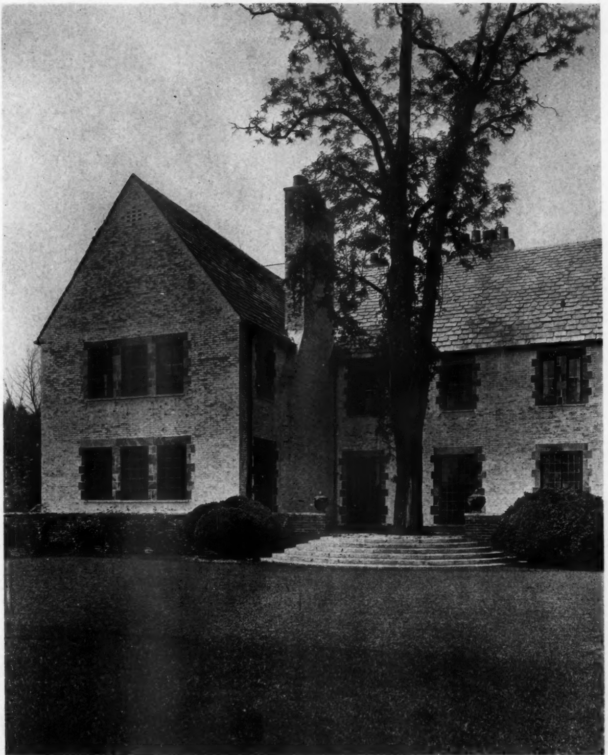
SOUTH END OF TERRACE FRONT, OVERLOOKING LONG ISLAND SOUND HOUSE AT PORT WASHINGTON, LONG ISLAND, N. Y.
