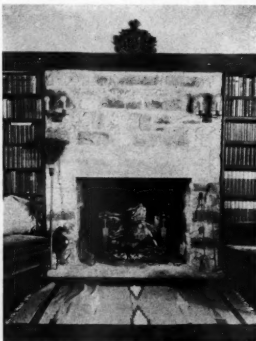
THE BACK PLATES OF THESE BRACKETS ARE OF WROUGHT IRON IN A CRUDE LEAF PATTERN TO HARMONIZE WITH THE STONE CHIMNEY BREAST. NOTE THE DARK STONES IN BACK OF THE LIGHTS IN THE HOUSE OF MELVIN PRATT SPALDING, ARCHITECT
