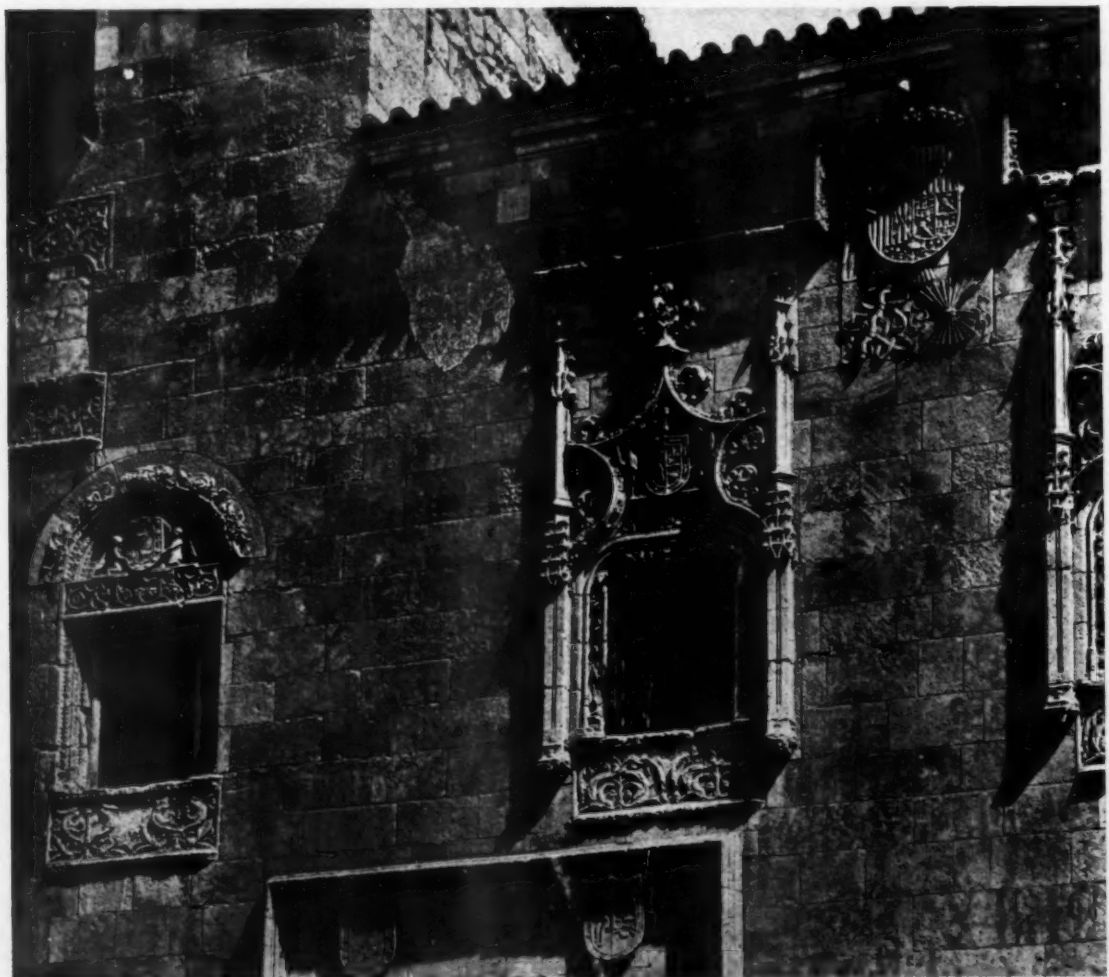
DETAIL OF WINDOWS, UNIVERSITY OF SALAMANCA, SPAIN
