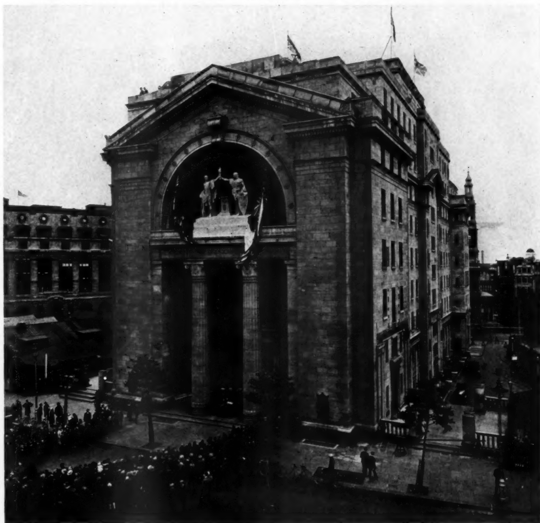
DETAIL OF ALDWYCH FRONT OF BUSH HOUSE, LONDON
