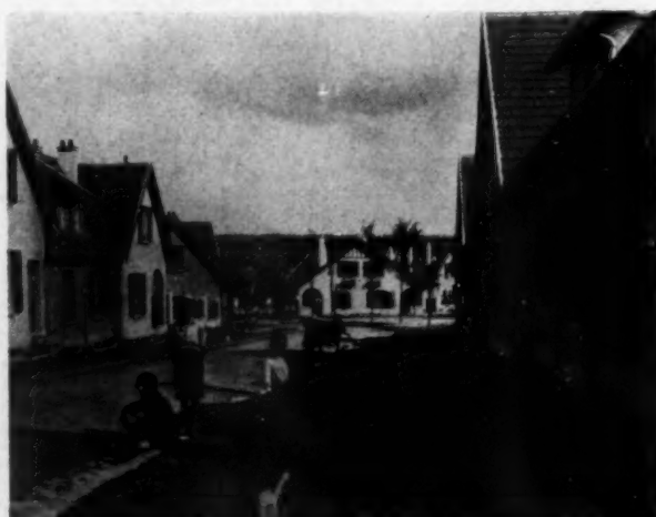
A HOUSING OPERATION IN FRANCE
