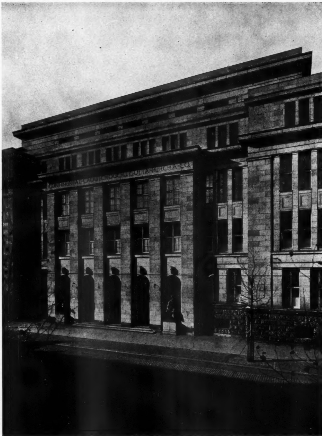
ENTRANCE PAVILION, OFFICE BUILDING OF THE CONTINENTAL CAOUTCHOUC & GUTTAPERCHA COMPANY, HANOVER
