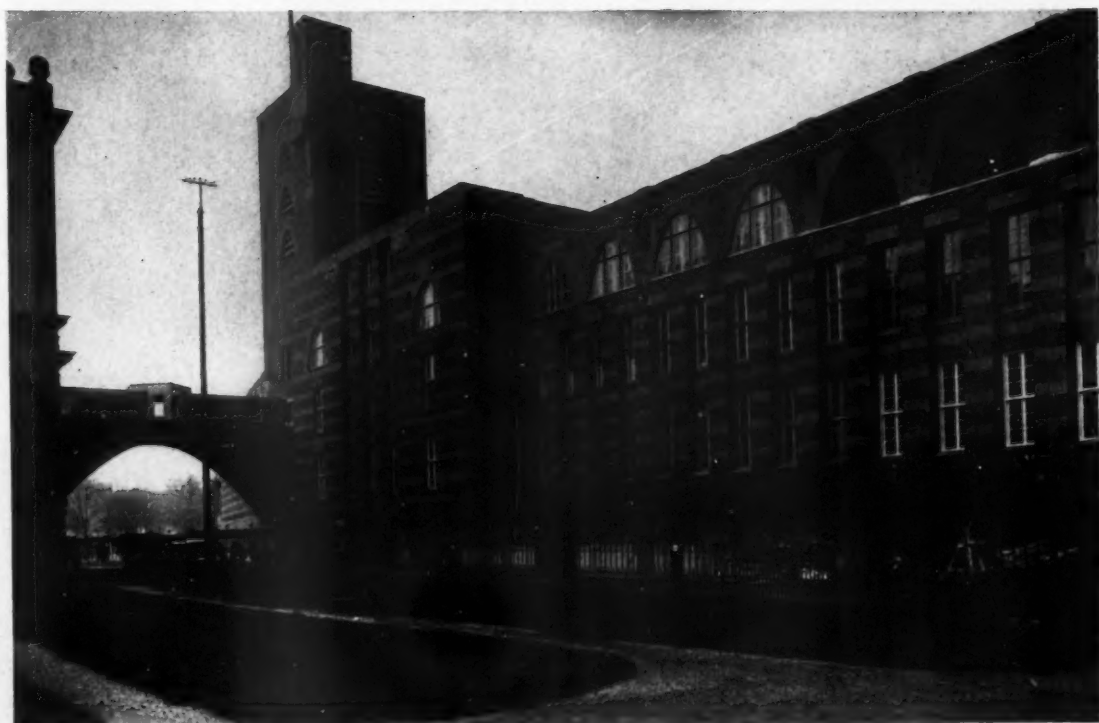
EXTERIOR VIEWS OF THE HÖCHSTER FARBWERKE, HÖCHST-ON-THE-MAIN PROF. DR. PETER BEHRENS, ARCHITECT
