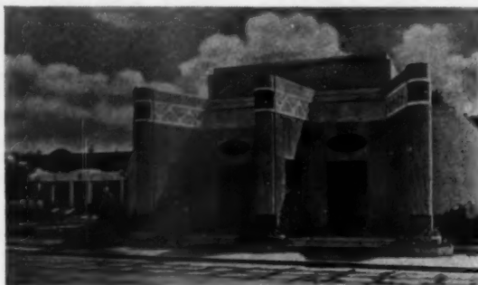
AN EXHIBITOR'S PAVILION
