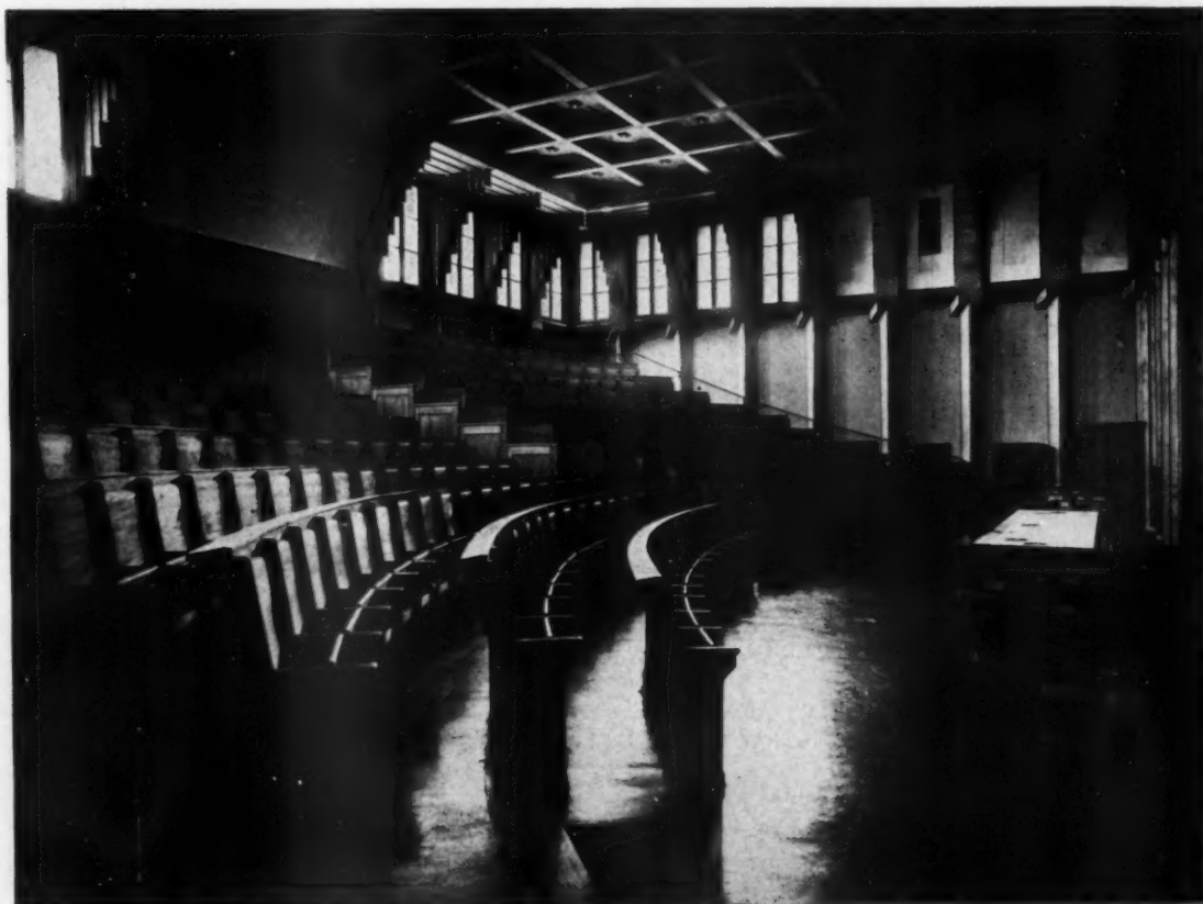
AUDITORIUM, OFFICE BUILDING OF THE HÖCHSTER FARBWERKE, HÖCHST-ON-THE-MAIN. WALLS, CEILING AND SEATS OF WOOD. BRICK DEMONSTRATION TABLE CONNECTED TO LABORATORY WITH A DUMBWAITER
