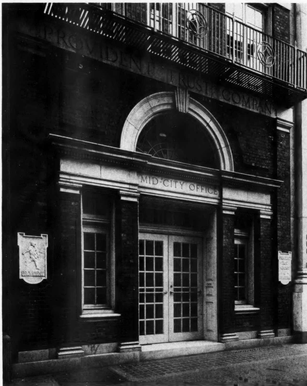
BUILDING FOR PROVIDENT TRUST CO., PHILADELPHIA, PA.
