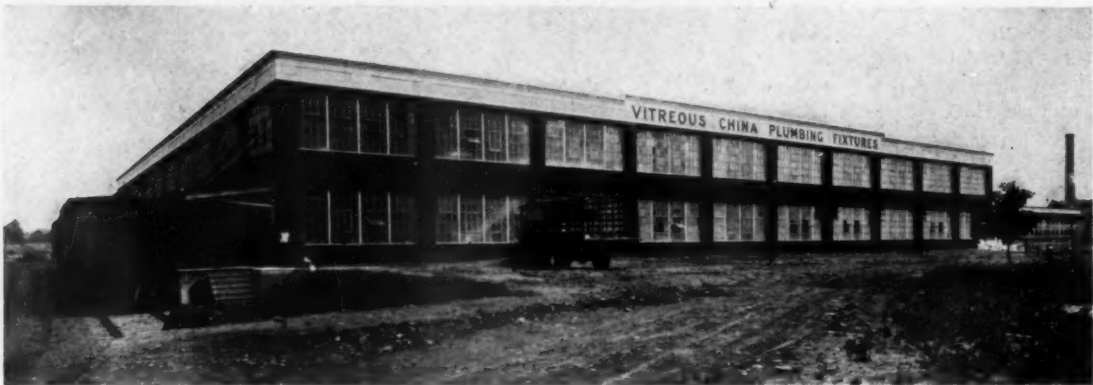
VIEW OF BUILDING NO. 1 FROM THE SOUTHWEST
