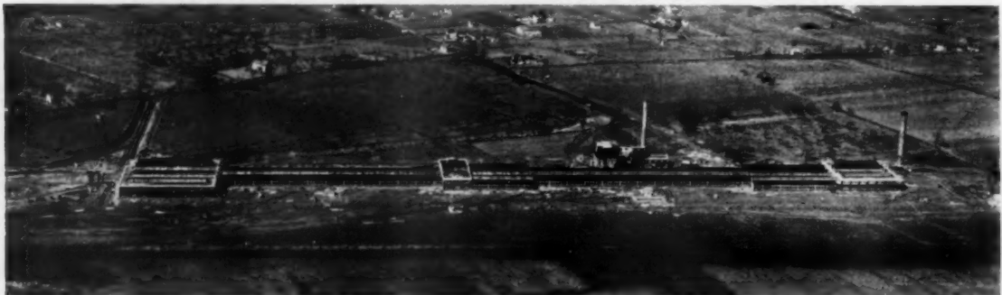
AIRPLANE VIEW OF THE PLANT DURING CONSTRUCTION, BUILDING NO. 1 AT LEFT AND BUILDING NO. 7 AND WATER TOWER AT RIGHT. PRODUCER GAS HOUSE, BOILER HOUSE, ENGINE ROOM AND CHIMNEY IN THE REAR OF BUILDING NO. 5
