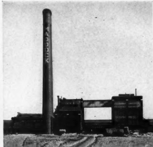
REAR VIEW OF GAS PRODUCER HOUSE, BOILER HOUSE AND ENGINE ROOM. CONVEYOR BRIDGE SERVING THE TWO SETS OF COAL BUNKERS
