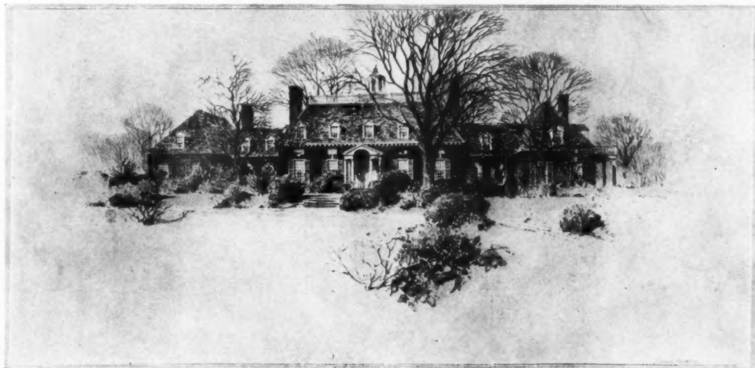
HOUSE OF WAYNE JOHNSON, LONG ISLAND
