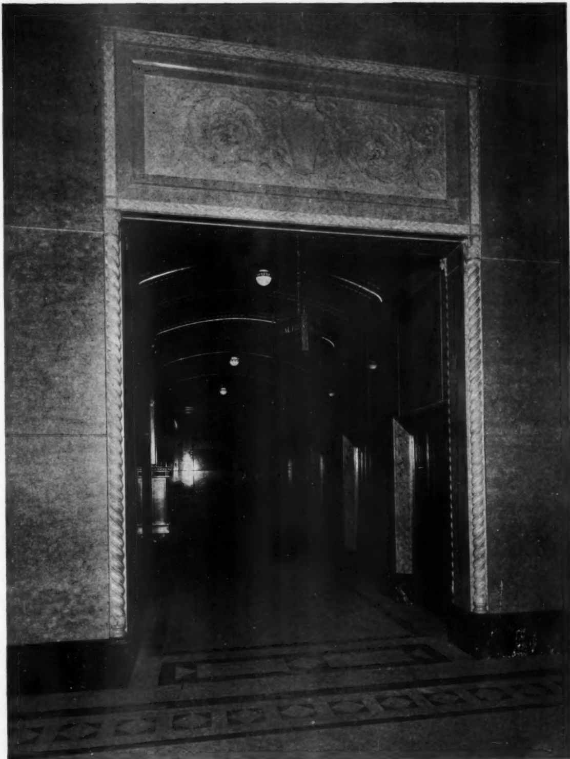
BUILDING FOR EQUITABLE ASSURANCE SOCIETY, SEVENTH AVENUE, NEW YORK STARRETT & VAN VLECK, ARCHITECTS
