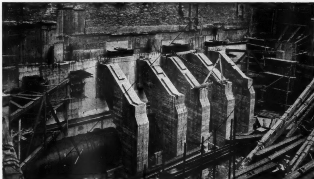
VIEW ALONG THE EAST BASEMENT WALL
