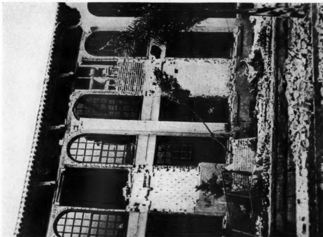
At left: One of the destroyed portions of the Alexandria Hotel illustrating the freak nature of the damage. At right: The structural damage to the Public Library consisted principally of the displacement of the cornices, and facing of the exterior walls, leaving windows intact
