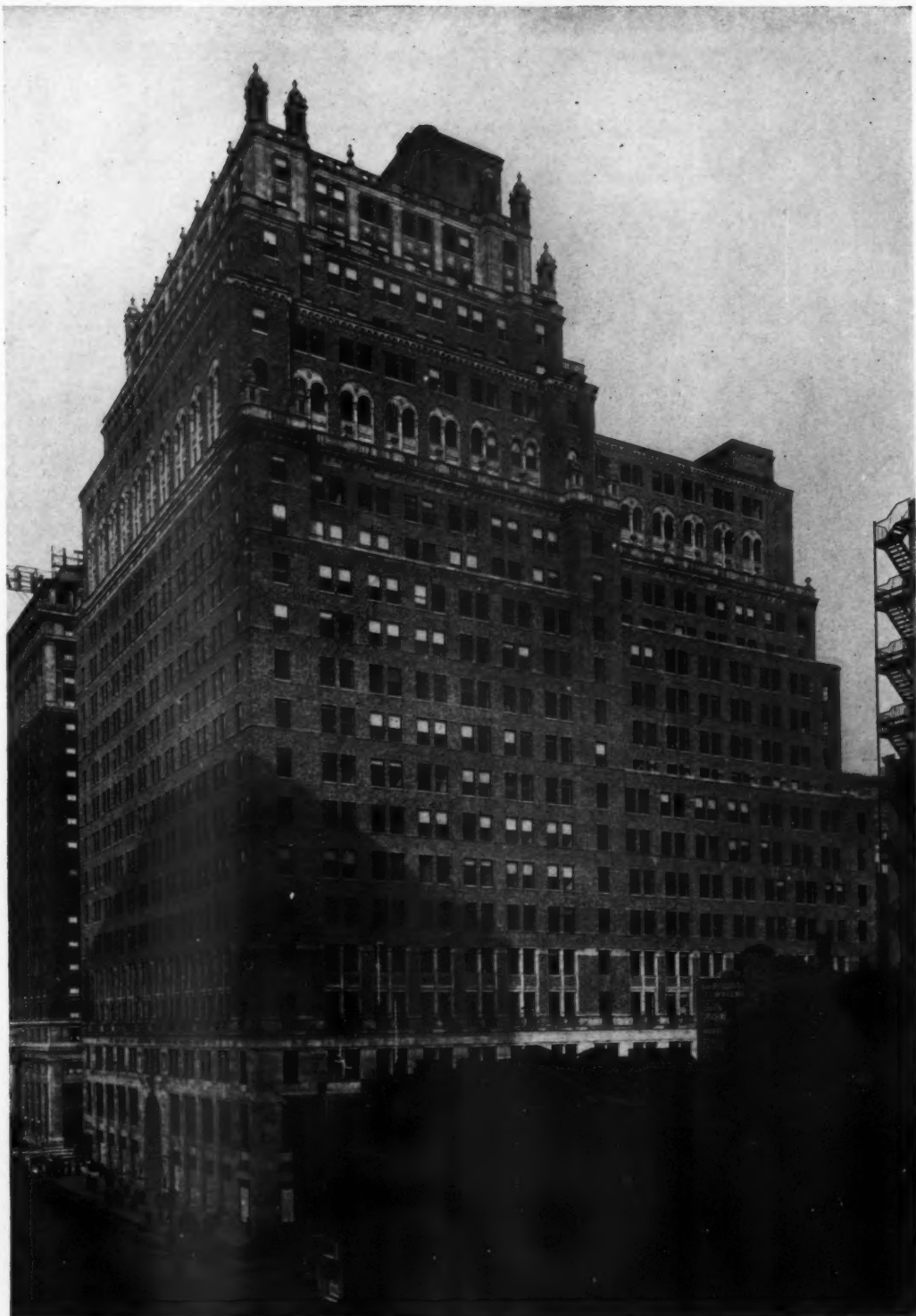
BUILDING FOR EQUITABLE ASSURANCE SOCIETY, SEVENTH AVENUE, NEW YORK
