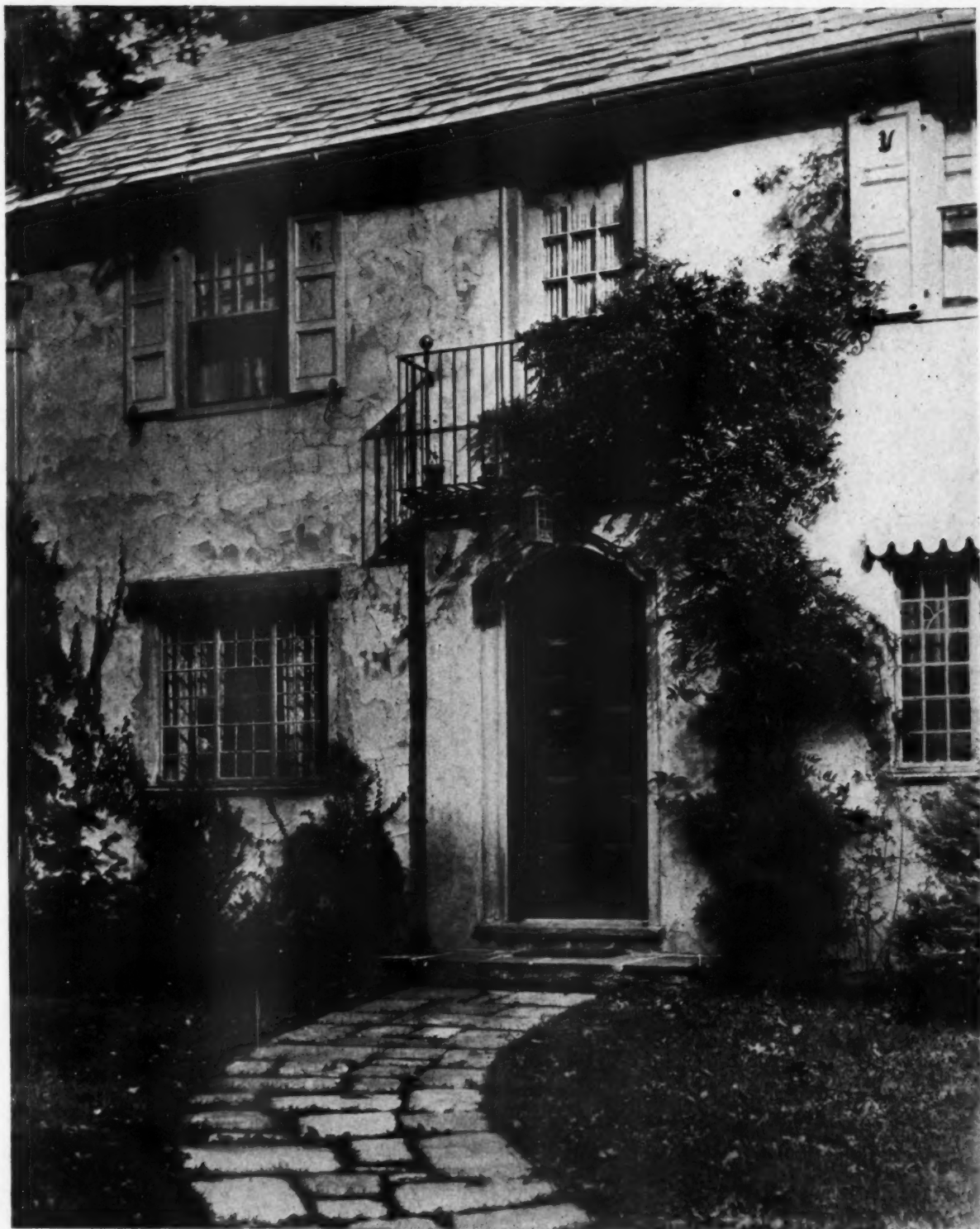
OWN HOUSE OF WILLIAM GEHRCN, ARCHITECT, PELHAMWOOD, N. Y.
