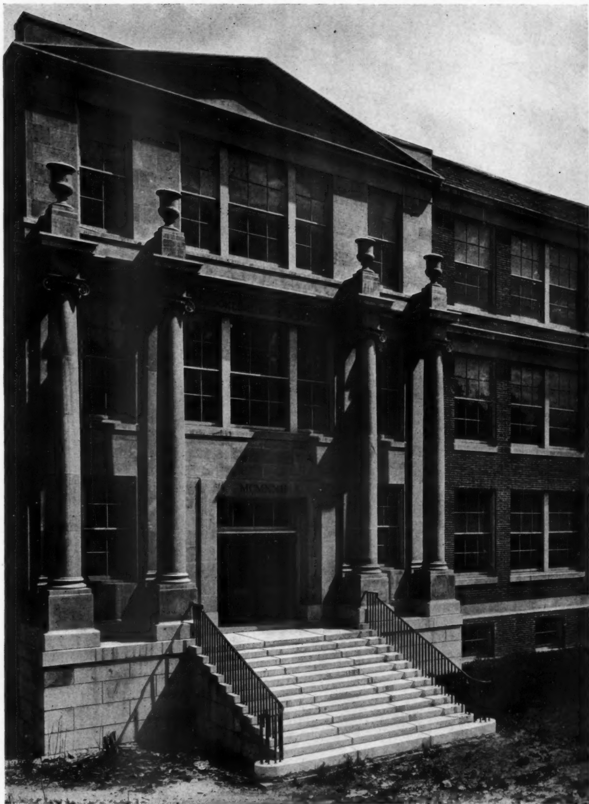
DETAIL OF ADMINISTRATION WING BROOKLINE HIGH SCHOOL, BROOKLINE, MASS. KILHAM, HOPKINS & GREELEY, ARCHITECTS
