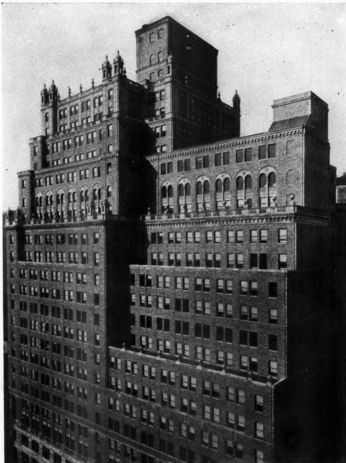
BUILDING FOR EQUITABLE ASSURANCE SOCIETY, SEVENTH AVENUE, NEW YORK
