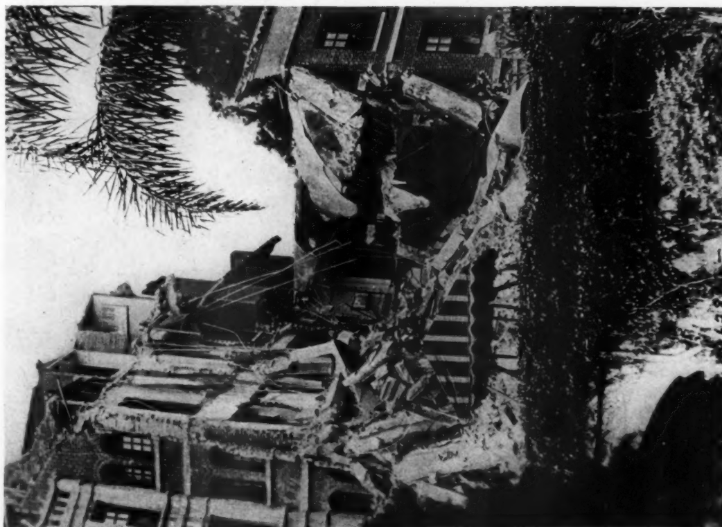
At left: One of the destroyed portions of the Alexandria Hotel illustrating the freak nature of the damage. At right: The structural damage to the Public Library consisted principally of the displacement of the cornices, and facing of the exterior walls, leaving windows intact
