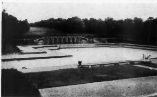
VIEW LOOKING SOUTHWEST
