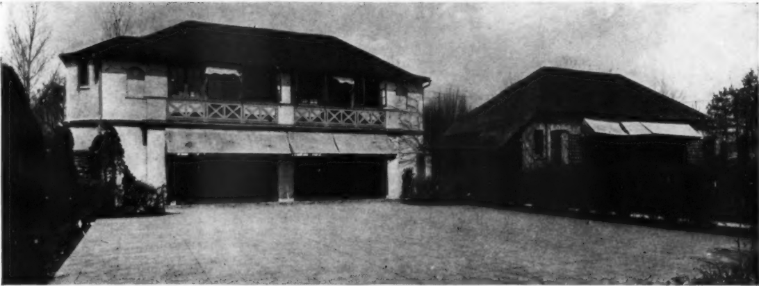
SOUTH VIEW OF PREPARATORY SCHOOL
