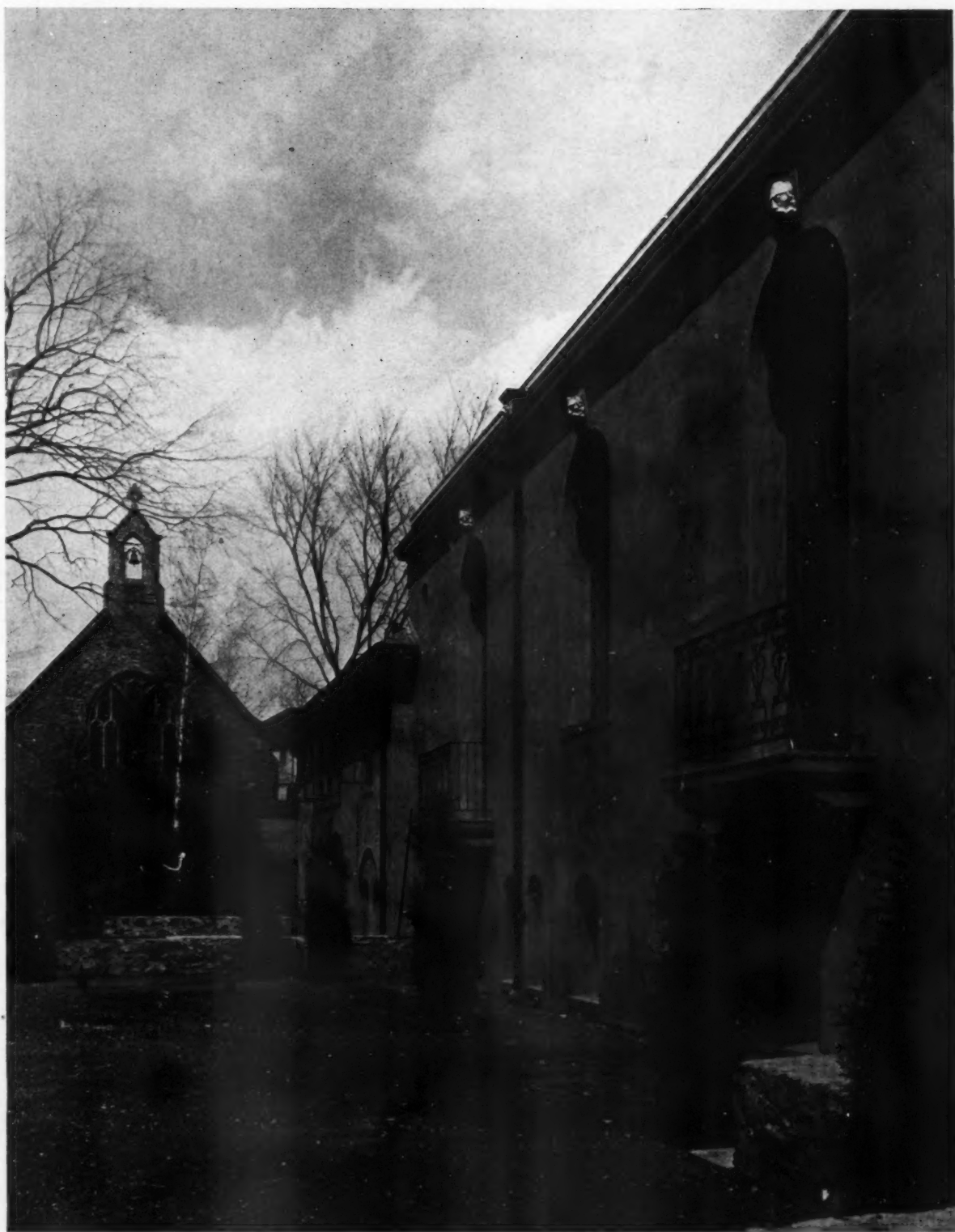
VIEW LOOKING ALONG WEST FRONT OF DINING HALL ROSEMARY HALL, GREENWICH, CONN., A SCHOOL FOR GIRLS THEODORE E. BLAKE, ARCHITECT
