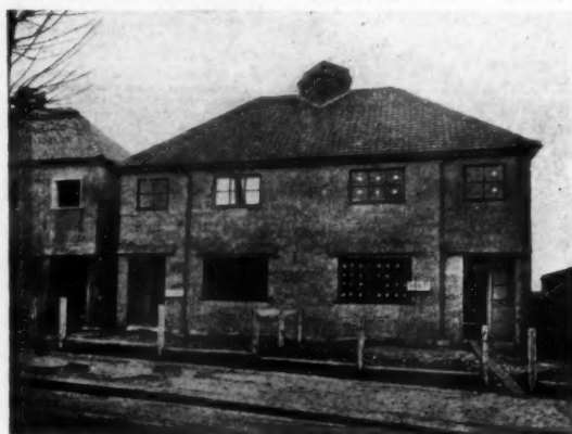
A STEEL HOUSE OF THE BRAITHWAITE TYPE
