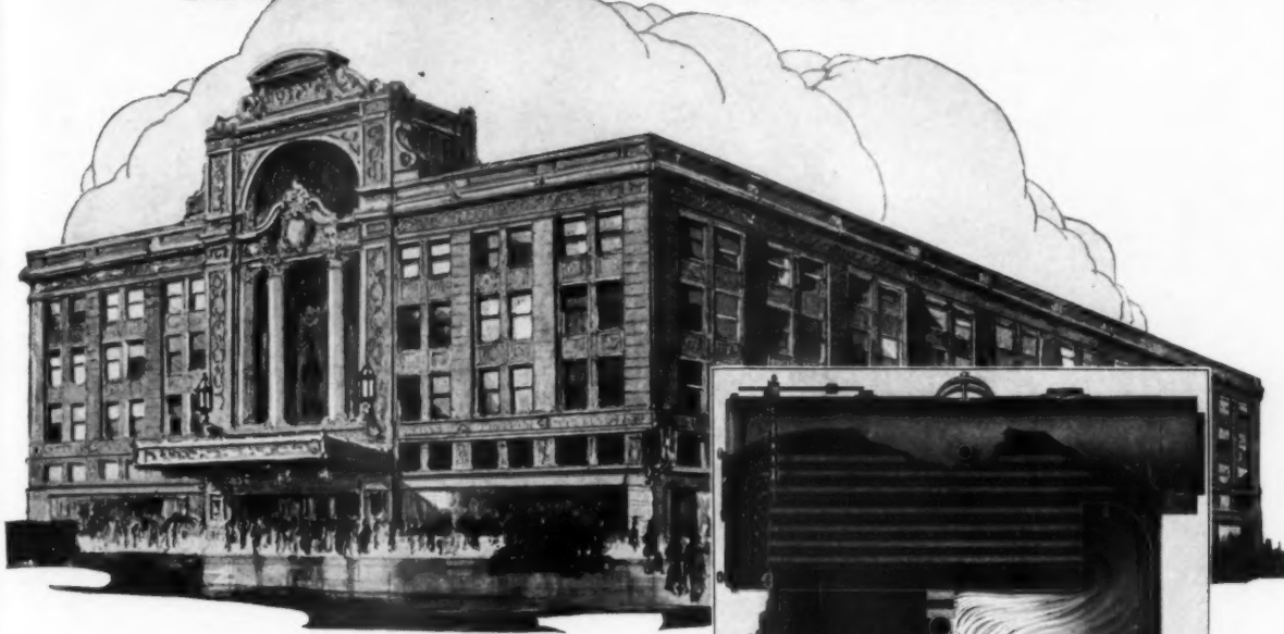
RIALTO THEATRE, Joliet, Illinois. Heated by Heggie-Simplex Boilers. Rapp & Rapp, Chicago, Architects. J. J. Borchard, Chicago, Heating Contractor.
