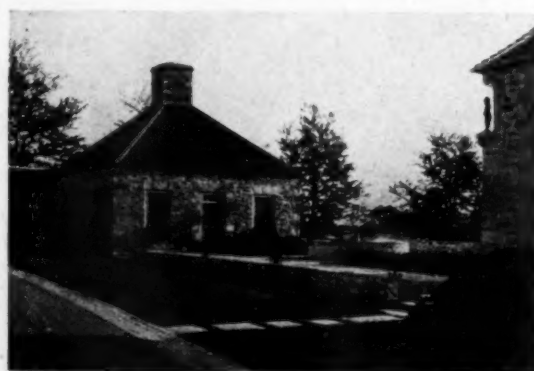
CARETAKER'S COTTAGE, ESTATE OF DONALD H. COWL, PORT WASHINGTON, L. I., N. Y.
