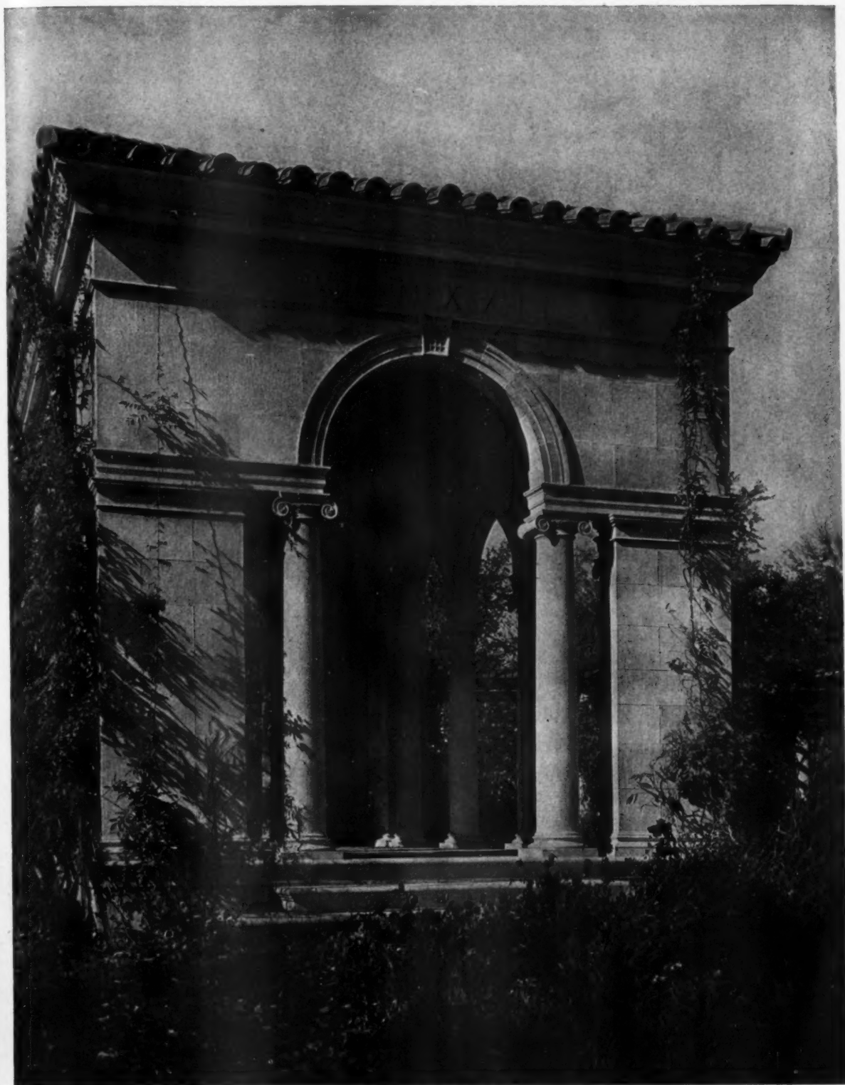
DETAIL OF GARDEN HOUSE, ESTATE OF J. A. TROWBRIDGE, NOROTON, CONN.
