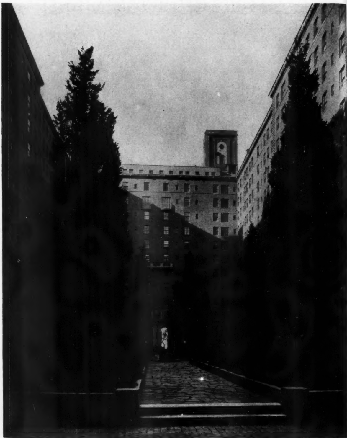
GARDEN COURT, APARTMENT HOUSE ON PARK AVENUE, NEW YORK McKIM, MEAD & WHITE, ARCHITECTS—FERRUCCIO VITALE, LANDSCAPE ARCHITECT (International Exposition of Architecture and Allied Arts)
