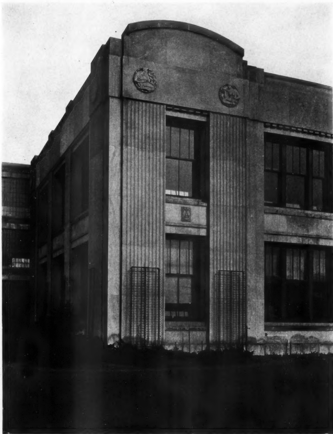
DETAIL OF BUILDING FOR HUDSON MOTOR CAR CO., DETROIT, MICH.
