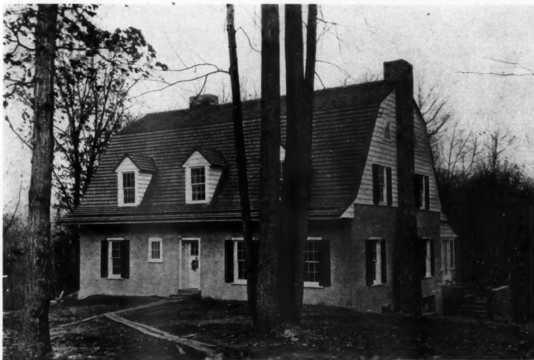
FRONT VIEW OF THE NEW RAMMED EARTH WALL HOUSE, THE FIRST IN THE UNITED STATES
