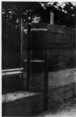
INTERIOR VIEW OF A WINDOW OPENING, SHOW- ING THE RECESS FOR THE WEIGHT BOX AND THE WOODEN NAILING BLOCKS
