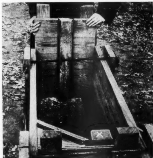
The rammers weigh about 15 pounds each. The large hardwood block is shod with iron and is the best for starting the work, the smaller ones are used for the finishing pounding
