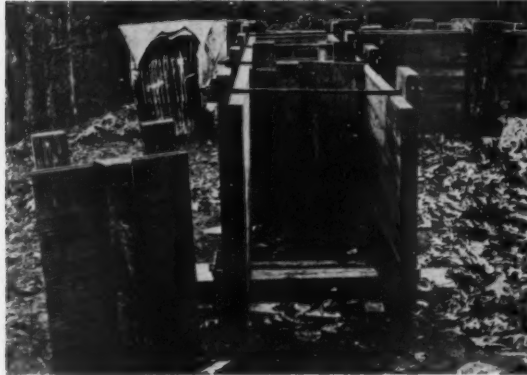
VIEW OF THE MOULD SET UP WITH THE END BLOCK READY TO BE PUT INTO THE FORM
