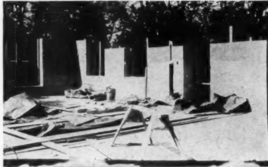
OPENING FOR THE FRONT DOOR AND TWO FRONT WINDOWS. AT THE LEFT OF THE DOOR IS A CHASE FOR THE SOIL PIPE
