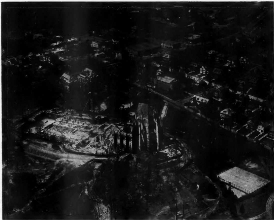
AIRPLANE VIEW OF FOUNDATION AND CHOIR CONSTRUCTION TAKEN IN WINTER OF 1922
