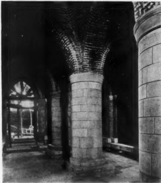
RECENT CONSTRUCTION PHOTOGRAPH OF CRYPTS
