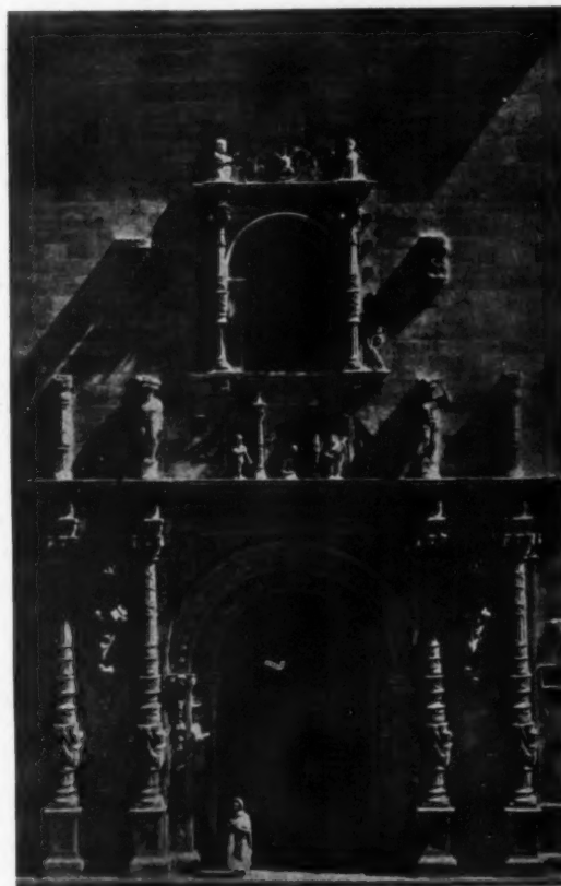
AN EXTERIOR FACADE MADE DOUBLY INTERESTING BY THE SHADES AND SHADOWS THROWN AND CAST BY THE DIRECT RAYS OF THE SUN
