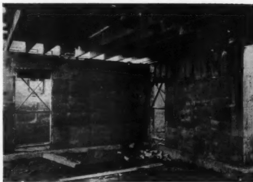
SECOND FLOOR JOISTS IN PLACE, WALL ENDS RESTING ON A WOODEN WALL PLATE. ONE COURSE OF FORMS STILL IN PLACE. THE DOOR FRAMES ARE SET IN PLACE AND THE WALL CAST AGAINST THEM, THE FRAME BEING STAYED TO PREVENT DISTORTION DUE TO THE PRESSURE OF THE CONCRETE
