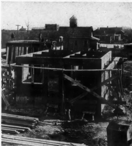
A HOUSE READY FOR THE ROOF RAFTERS AND CEILING JOISTS, THE WALL PLATE IN POSITION AND ANCHORED TO THE WALL. THE INTERIOR PARTITIONS ARE COMPLETE AND BUILT UP WITH THE EXTERIOR WALLS
