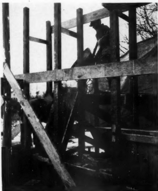
SECTIONAL WOODEN FORMS SET UP BETWEEN UPRIGHT WOODEN POSTS. THE LABORER IS DEPOSITING THE CONCRETE BY MEANS OF A CHUTE INTO THE FORMS WHERE IT IS PUDDLED SLIGHTLY IN ORDER TO REMOVE THE ENTRAINED AIR
