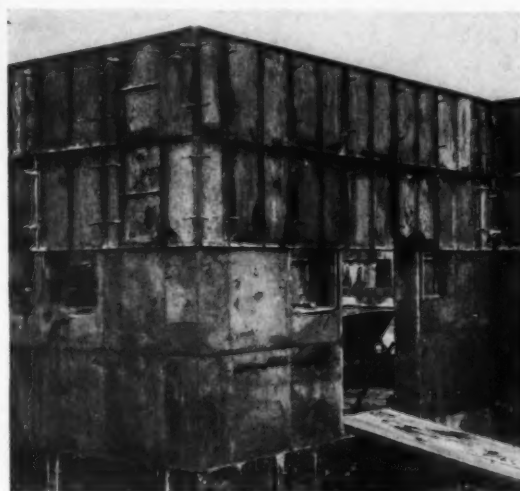
FORMS MADE OF SHEET STEEL WITH ANGLE IRON FRAMES WHICH ARE EASILY FASTENED TOGETHER AND REMOVED AFTER THE CONCRETE IS SET. THE DOOR AND WINDOW FRAMES AND BUCKS ARE SET UP BETWEEN THE FORMS
