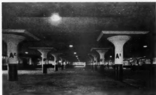
THE PUBLIC GARAGE ON THE SECOND FLOOR OF THE MARKET BUILDING
