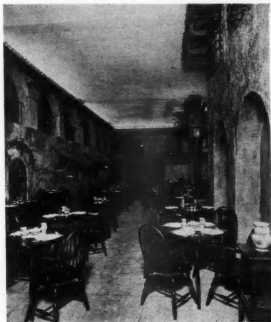
LOOKING TOWARD THE STAIRCASE IN THE DISTANCE
