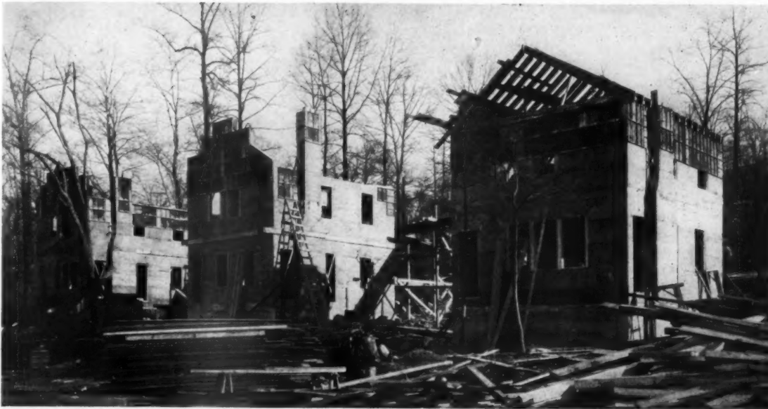
A GROUP OF TWO STORY DWELLINGS, UNDER CONSTRUCTION, WHOSE WALLS ARE BUILT OF STRUCTURAL QUALITY GYPSUM CONCRETE. NOTE THE EASE WITH WHICH THE FORMS ARE APPLIED TO THE WALLS, THE GABLES AND THE CHIMNEYS
