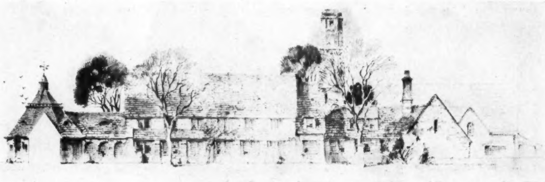
DINING HALL AND SERVICE WING
