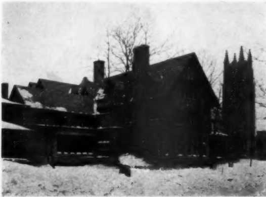
SUNDAY SCHOOL AND SOCIAL BUILDING, FIRST CONGREGATIONAL CHURCH, OAK PARK, ILL.
