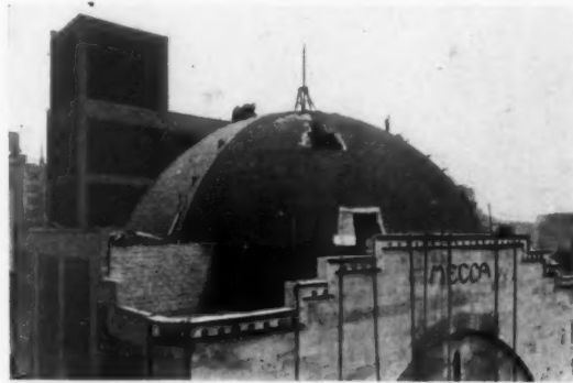
THE DOME COVERED WITH ROOFING FELT AND PARAFFIN. THE LOWER HALF IS PARTIALLY COVERED WITH ROOFING TILE
