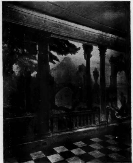
A WALL OF THE CORRIDOR
