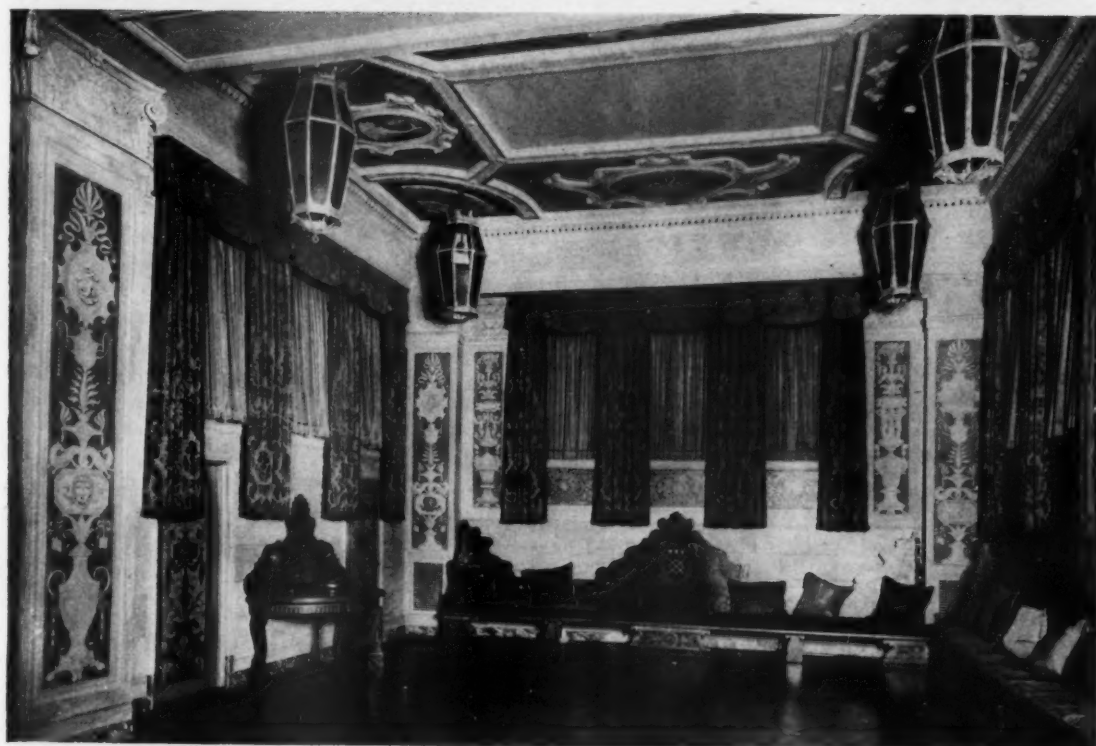
OPPOSITE ENDS OF THE BALLROOM, TWENTY-TWO FEET WIDE THE SULGRAVE, NEW YORK ROUSE & GOLDSTONE, ARCHITECTS—ARDEN STUDIOS, DECORATORS MURALS BY J. ALDEN TWACHTMAN
