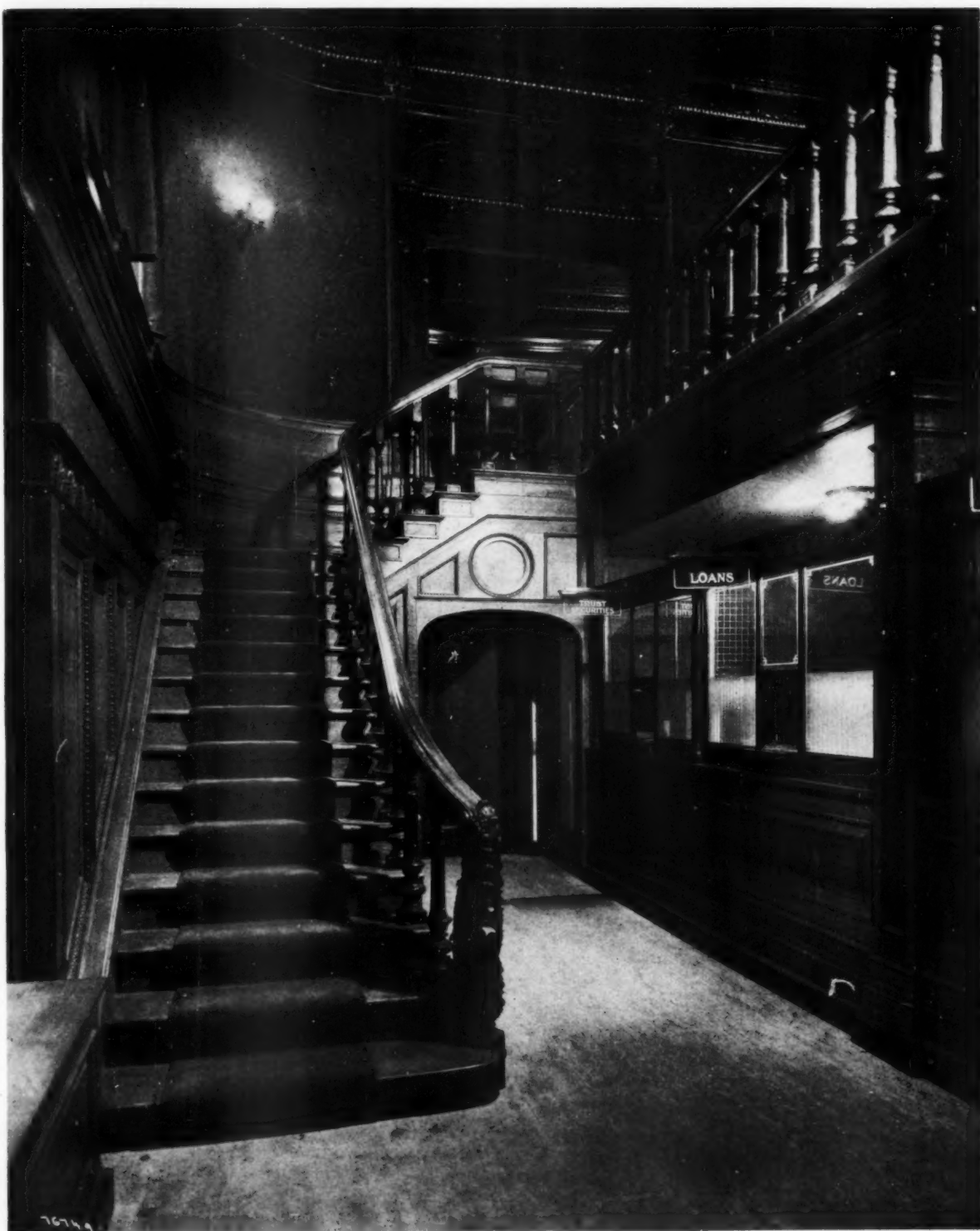
STAIRWAY TO MEZZANINE FLOOR
