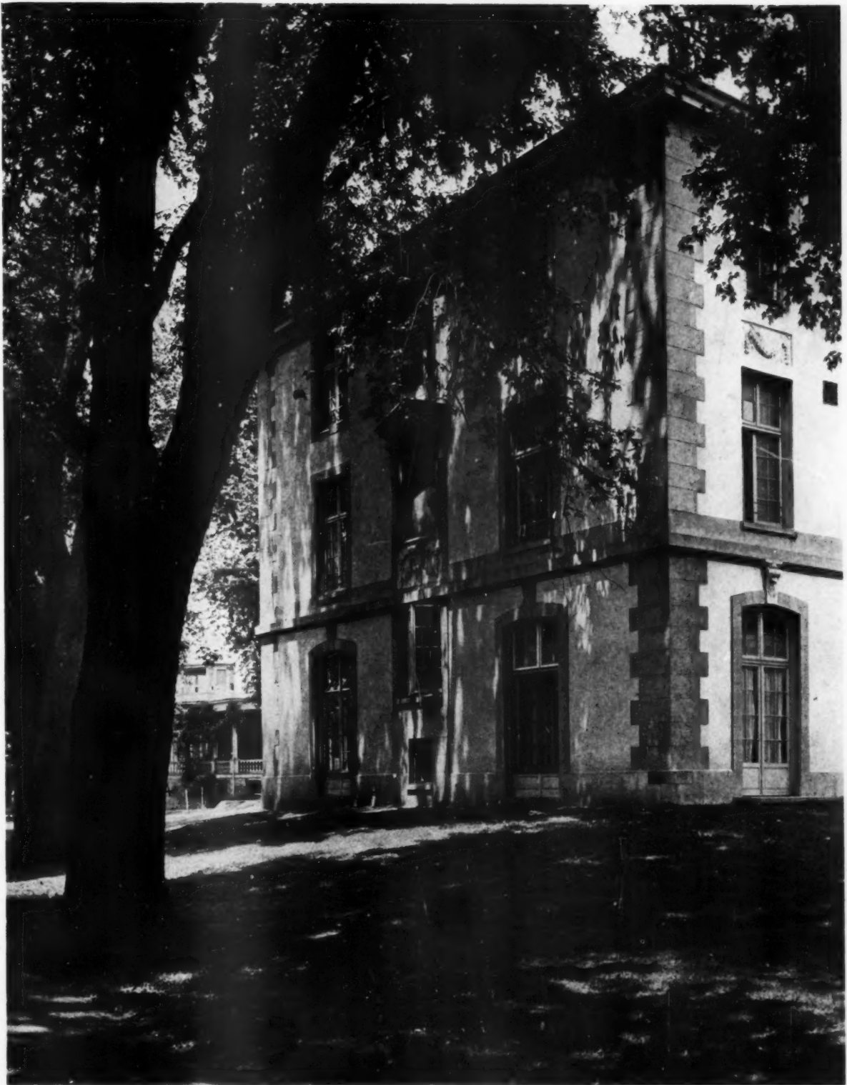
DORMITORY BUILDING, ASYLUM OF ST. VINCENT DE PAUL, TARRYTOWN, N. Y.
