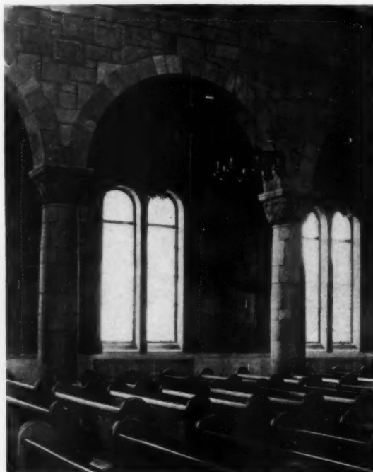
NORTH WALL OF THE NAVE
