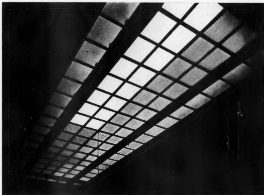
View of ceiling light from the corner of the gallery. Compare the brightness of the light which is refracted by the prismatic plates to the near side wall and corner with the light which is transmitted vertically. The border lights are of plain etched glass
