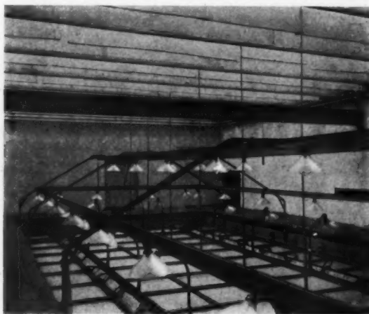
View below the louvres which are set for noontime in mid-winter, all louvres vertical and parallel, looking north
