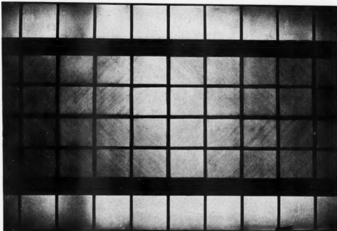
View of the ceiling light directly below its center, showing the prismatic plates refracting the light toward the side walls. Compare the dimness of the light which is transmitted vertically with the brightness of the light which is refracted toward the wall shown in upper illustration on page 587. The border lights are of plain etched glass
