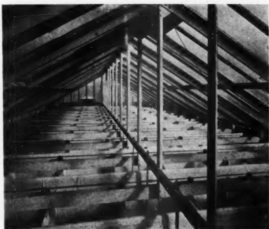
View taken above the louvres which are in cellular position for morning, evening or overcast sky conditions
