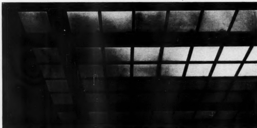
View of ceiling light looking directly across the room near its end. Compare the brightness of the light which is refracted by the prismatic plates directly to the near side wall with the light that is transmitted vertically. The border lights are of plain etched glass
