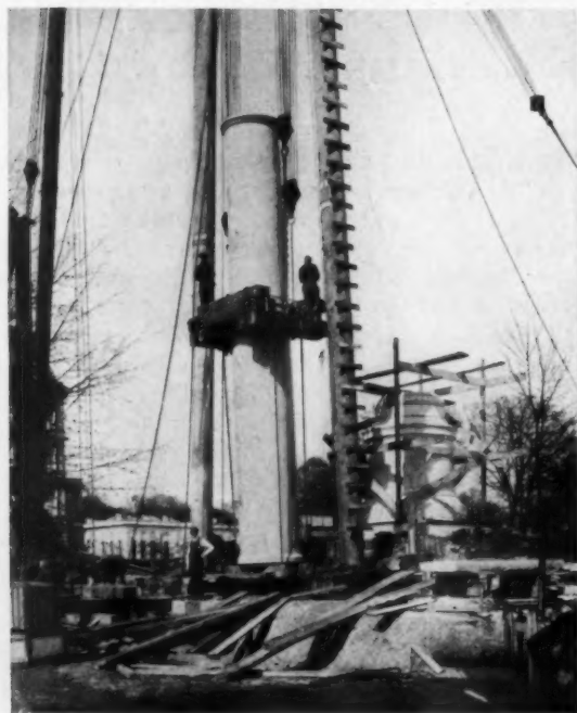
THE SHAFT RAISED TO A VERTICAL POSITION. A SET OF CLAMPS NEAR THE CENTER AND CROSS TIMBERS UNDER THE BOTTOM OF THE SHAFT ARE IN PLACE, READY FOR THE INSTALLATION OF THE SECOND SET OF CLAMPS NEAR THE BOTTOM
