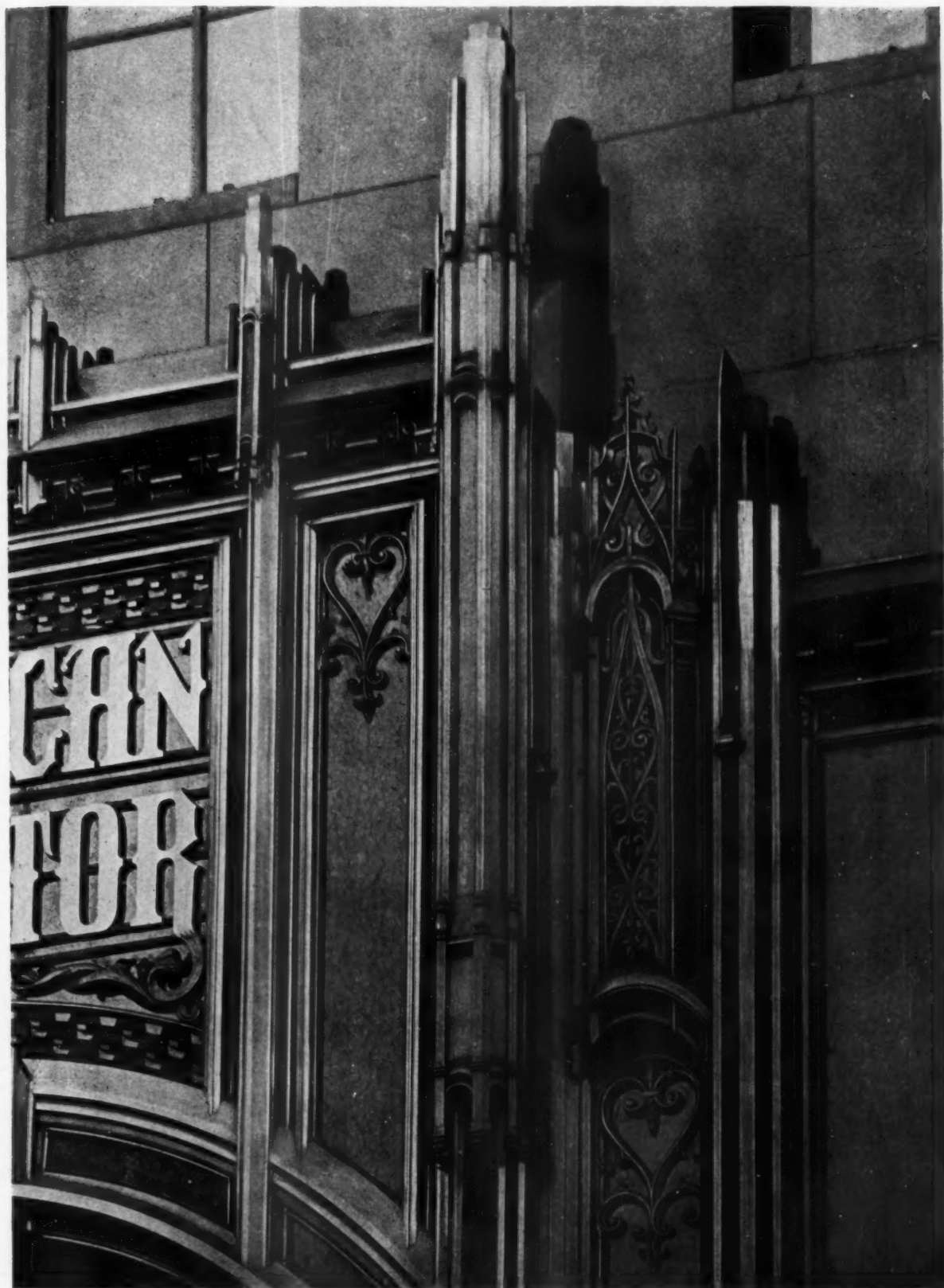
BRONZE DETAIL, MAIN ENTRANCE BUILDING FOR AMERICAN RADIATOR CO., WEST 40TH STREET, NEW YORK RAYMOND M. HOOD, ARCHITECT
