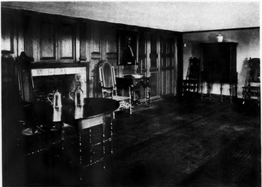
ROOM BUILT AROUND THE PANELLED FIREPLACE WALL WHICH CAME FROM A HOUSE IN PORTSMOUTH, R. I. The design is a provincial rendition of the Renaissance theme, with stile and rail panelling set between pilasters whose flutes are reeded in their lower portions
