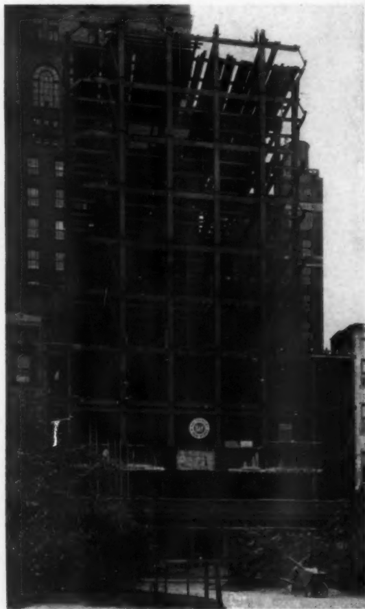
LOWER PORTION OF THE STEEL FRAME SHOWING THE REARRANGEMENT OF THE FRONT COLUMNS AT THE THIRD FLOOR AND THE CORNER BAY CONSTRUCTION
