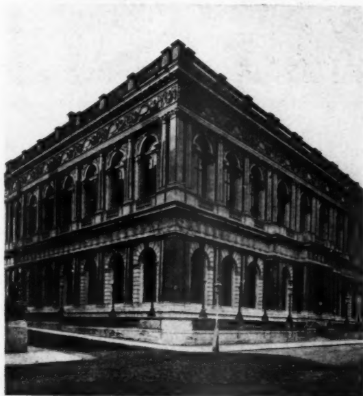
THE CARLTON CLUB, PALL MALL, LONDON, BEFORE REFACING
