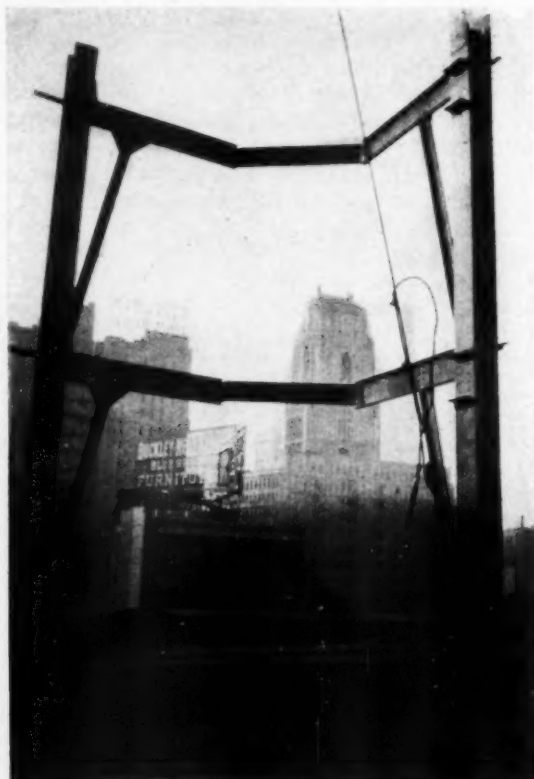
A DETAILED VIEW OF THE CORNER BAY CONSTRUCTION
